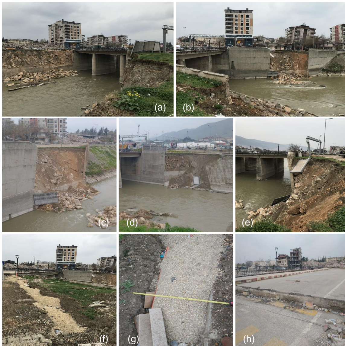
Figure 64: Bekir Karabacak Bridge / Retaining wall failure (36.215443, 36.162129). (a-e) retaining wall failure, (f-g) slope instability related cracks (h) vertical displacement.
