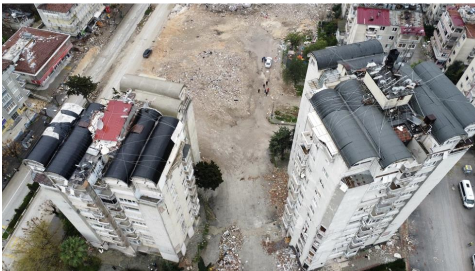
Figure 151: Aerial drone footage of remaining two blocks after the earthquake.
