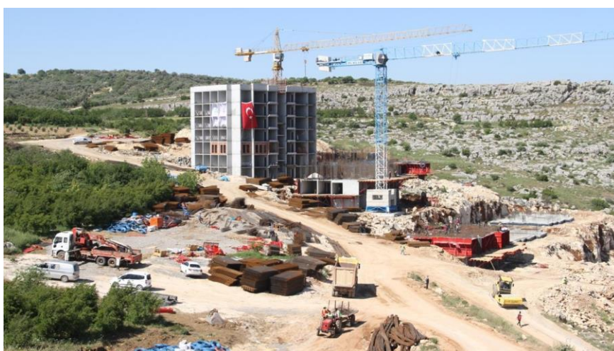
Figure 259: Hatay Altınözü Permanent Housing Area in Antakya province (TRT Haber, 03.05.2023)
