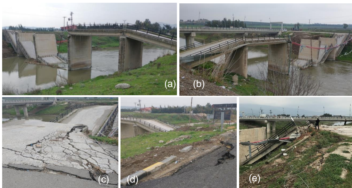
Figure 58: Hatay state hospital bridge (a) the old bridge (b) the new bridge behind the old one (c) slope failure at the connection point of the deck with the ground (d) slope failure next to the bridge (e) slope failure at the connection point of the deck with the ground.
