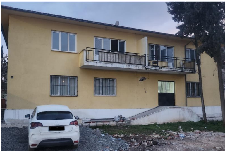
Figure 154: Standing masonry building at Fevzipaşa Train Station.
