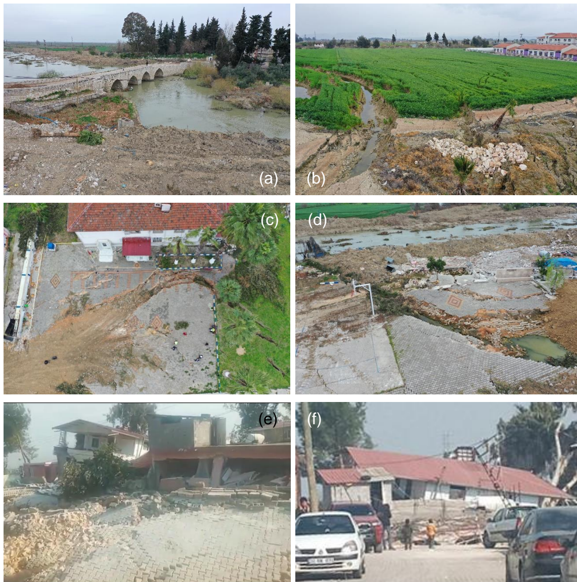
Figure 53: Liquefaction-related failures in Demirköprü. (a) The masonry bridge of Demirköprü did not suffer major damage (36.248750, 36.354769), (b) Lateral spreading cracks in close proximity to the masonry bridge, (c) Lateral spreading at the school of Demirköprü (36.250107, 36.352776), (d) Lateral spreading towards the river, (e-f) Shallow founded structures in the zone of spreading next to the school of Demirköprü
