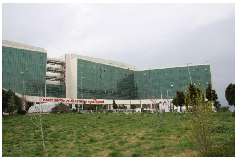
Figure 185: Hatay State Hospital (as observed on 14 of March 2023)
