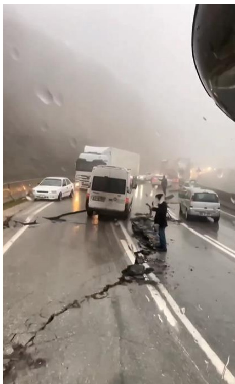
Figure 202: Reduced road capacity by cracked pavement – retrieved from https://www.instagram.com/reel/CpxR_U9ouLT/?ugsgud=YzAyMDM1MGJkZA%3D%3D
