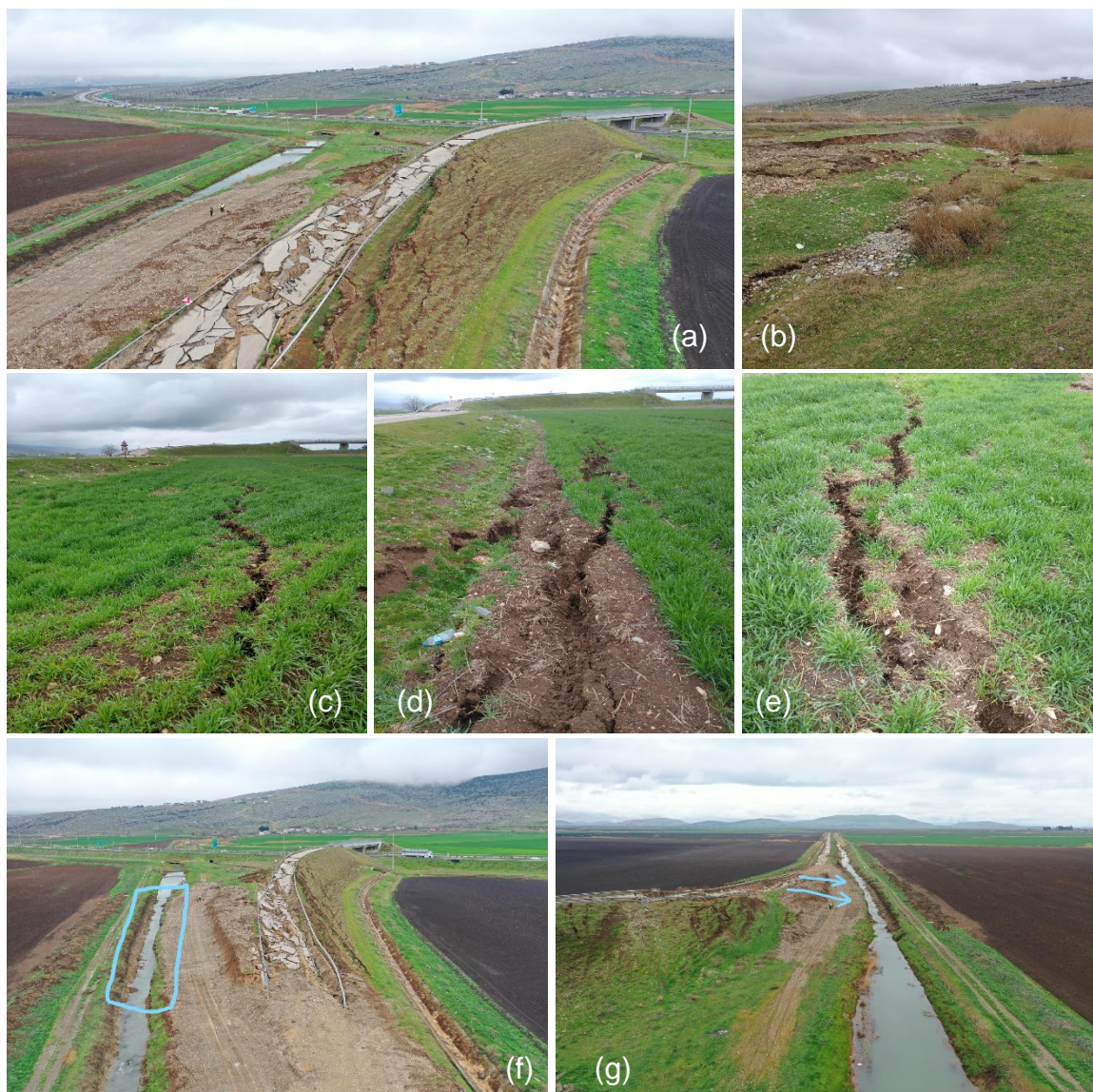
Figure 63: Embankment between the villages of Evri and Çöçelli (37.283724, 37.113888). (a) general view of embankment failure, (b-e) surface crack, (f-g) water channel-related failure
