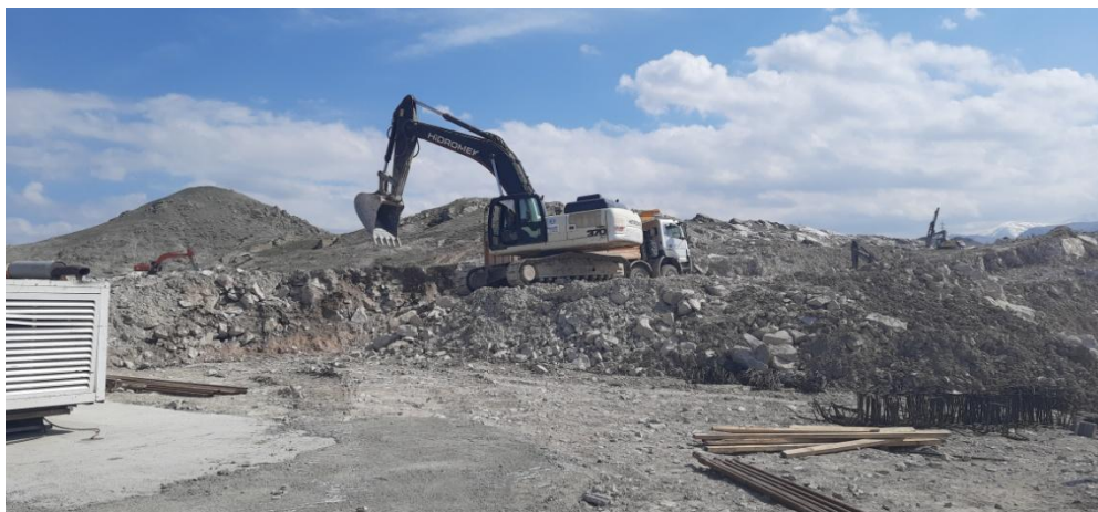
Figure 263: GelincikTepe Permanent Housing Area in Malatya province.
