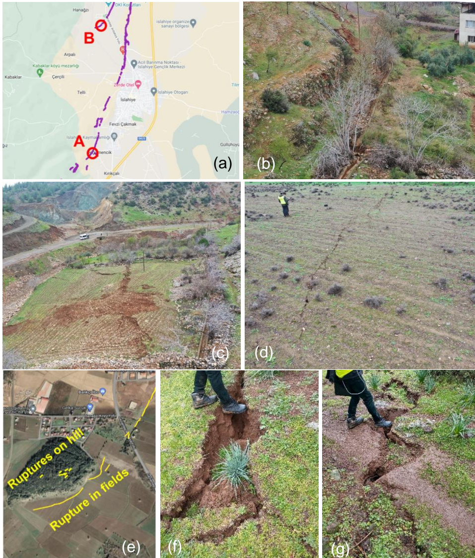
Figure 37: Observations of surface rupture in locations around Islahiye. (a) Areas where the surface rupture was inspected by the field team, (b) Surface rupture manifesting along a slope in area A. Notice the toppled electricity transmission tower and the lateral displacement along the canal. (c) Fault surface rupture in area A. (d) Rupture in the plains of area B. (e-g) Surface rupture on a hill in area B. Multiple fissures were visible, which were deeper and wider than the rupture observed in the fields.
