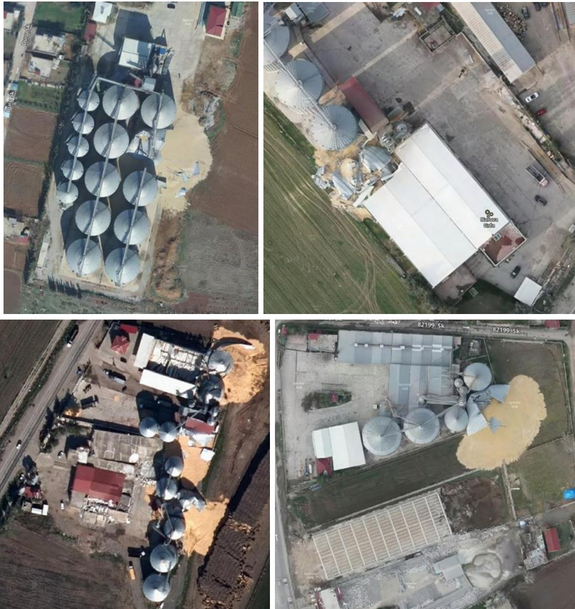
Figure 220: Satellite images of grain silo failures.
