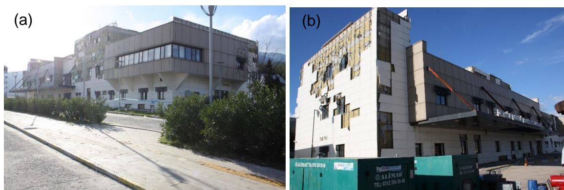
Figure 184: Nurdağı State Hospital (as observed on 15 of March 2023)
