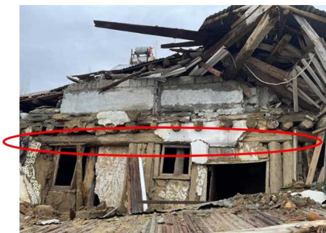
Figure 115: Timber beams on the top of the openings.
