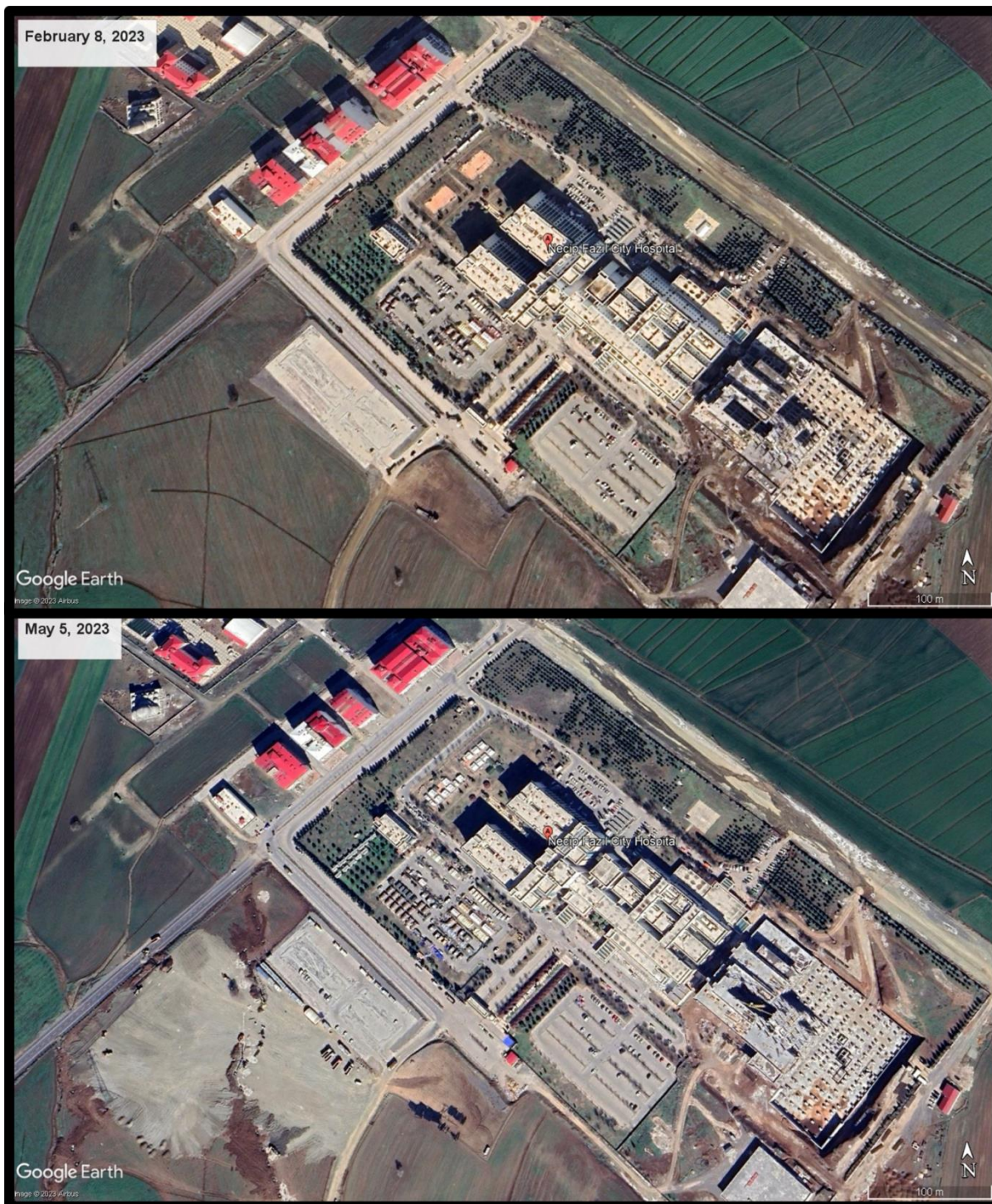
Figure 254: Rubble piles nearby NecipFazıl City Hospital in Dulkadiroğlu, Kahramanmaraş.
