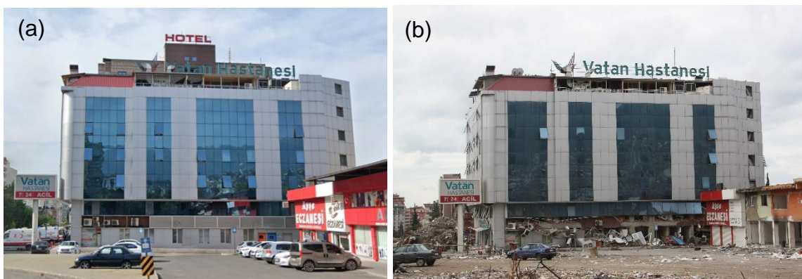
Figure 181: Vatan Private Hospital (Kahramanmaraş), north façade: a) before (Google Maps Street view) and b) after the earthquake (as observed on 16 of March 2023)
