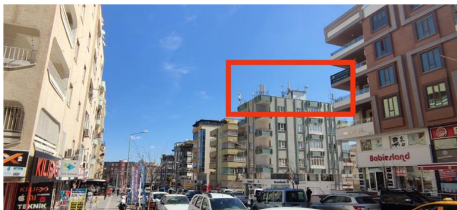
Figure 232: A base station on the rooftop a building.
