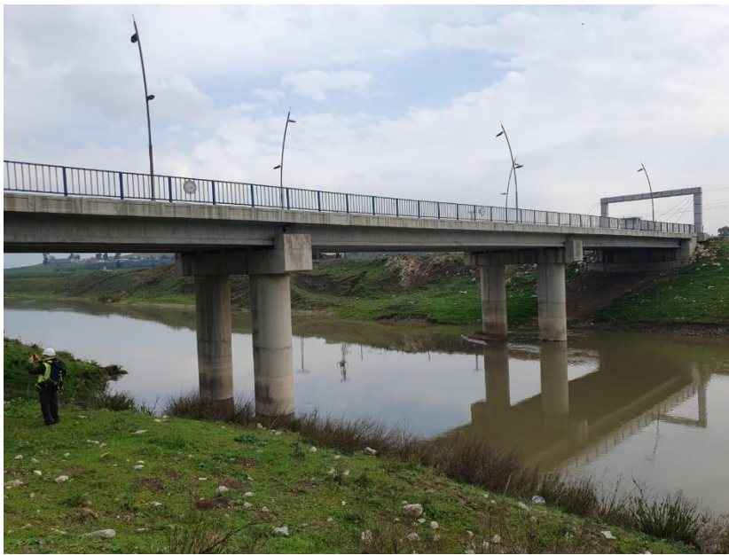
Figure 200: An intact bridge crossing the Karasu çayı river (location: Lon 36.2724, Lat 36.2074)
