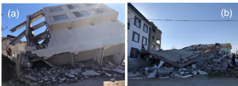
Figure 95: Torsional damage (a) Knife-cut damage in Gölbaşı/Adiyaman; (b) Torsional collapse in Center/Adiyaman.
