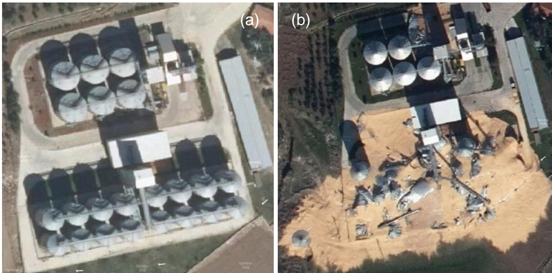
Figure 222: Satellite image of Nurdağı Grain Silos, before (a) and after (b)
