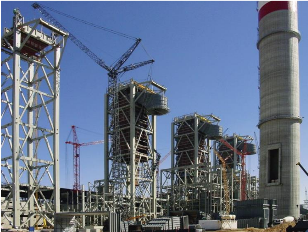
Figure 215: Construction Photo of Afşin-Elbistan B
