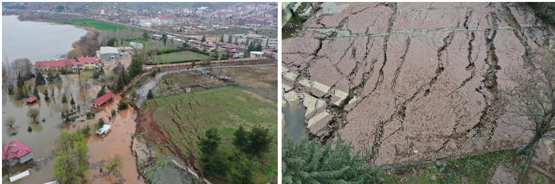
Figure 56: Lateral spreading in a lake-side park in Gölbaşı (37.794157, 37.649400).
