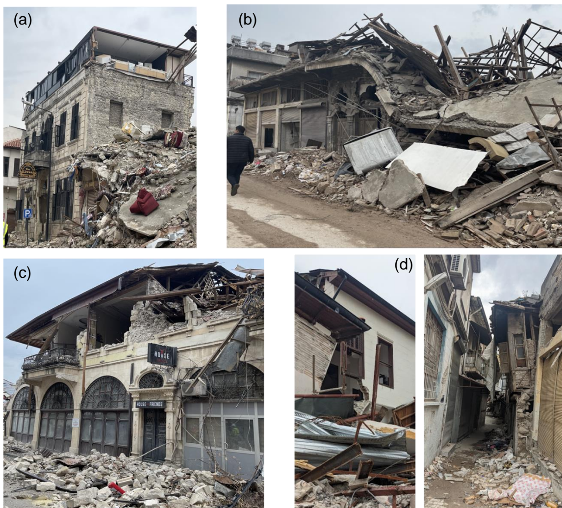
Figure 111: (a) Failure of the veranda built on the original building, (b) Failure of the RC flooring built to replace the original floor, (c) Lack of connections within party walls and bearing walls, and (d) Failure due to pounding.
