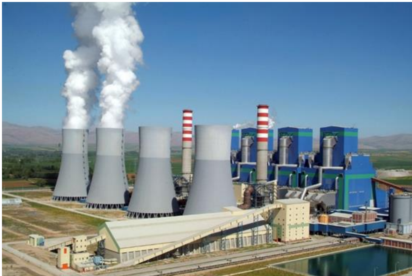
Figure 214: Afşin-Elbistan B Thermal Power Plant
