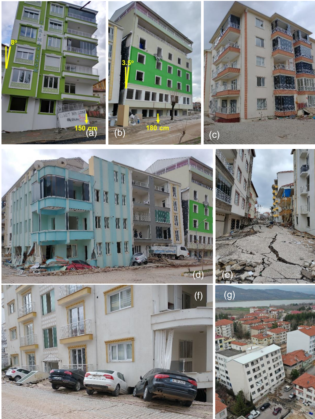
Figure 57: Liquefaction-related damage of buildings in Gölbaşı. (a) Building with a shallow foundation (37.789275, 37.645262) (b) Building founded on piles (37.787486, 37.642252) (c) Settlement of residential building (37.788127, 37.642037) (d) Series of buildings affected by liquefaction (37.787687, 37.642644) (e) Series of buildings affected by liquefaction (37.787367, 37.642858) (f) Large settlement of structure with shallow foundation (37.787958, 37.643190) (g) Significant tilting (37.787730, 37.643366)
