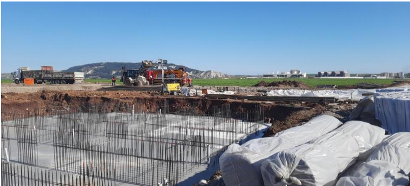
Figure 262: İndere Permanent Housing Construction Site in Adıyaman province.
