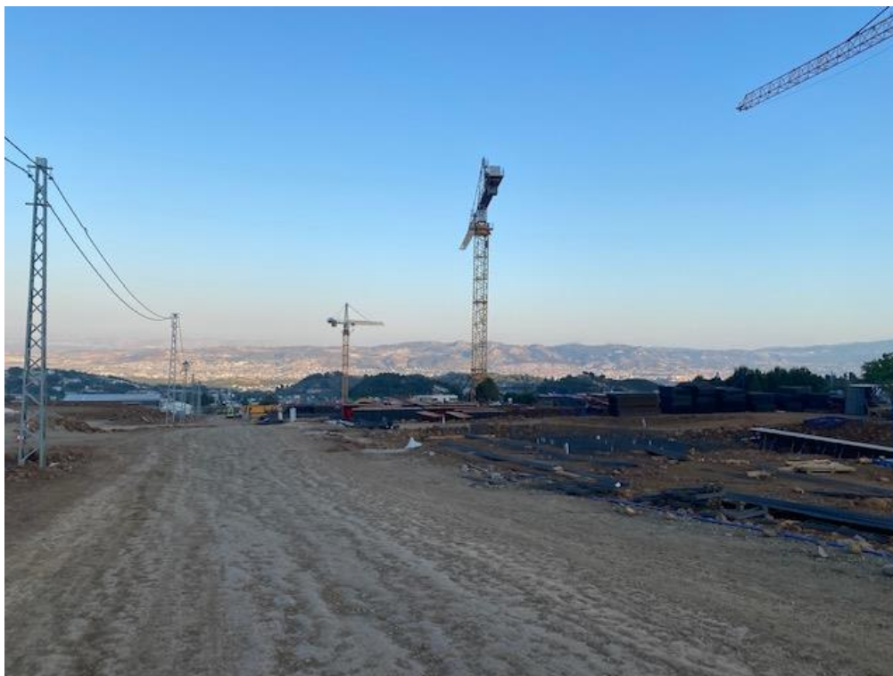
Figure 264: Permanent Housing site under construction in June 2023, Gülderen Neighbourhood, Antakya
