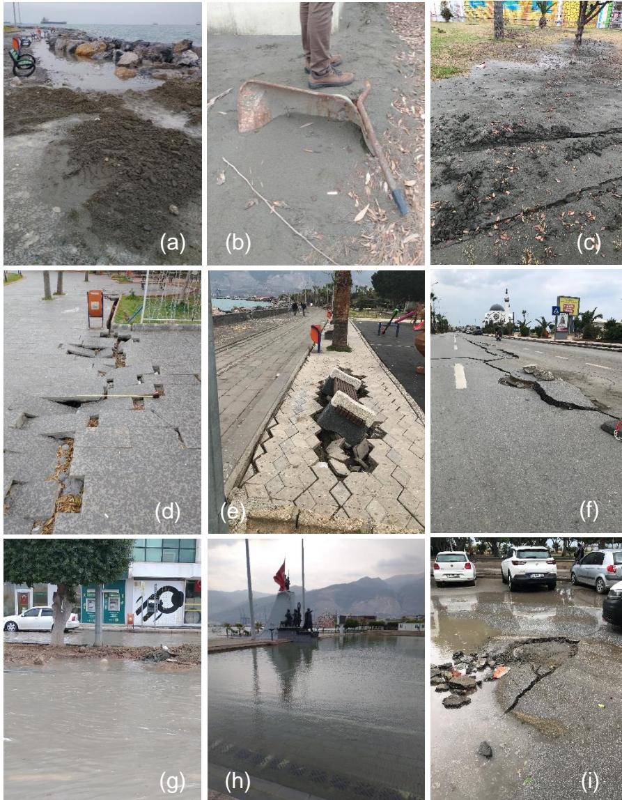
Figure 49: Characteristic surface features of liquefaction in İskenderun. (a) Sea wall movement (b-c) Ejected material (d-e) Lateral spreading crack, Yenişehir district C Boulevard, Pirireis district. (g) Subsidence along Atatürk Boulevard, Yenişehir district. (h) İskenderun Anıt Meydanı square subsidence. (i) Manhole in Atatürk Boulevard, Yenişehir district.
