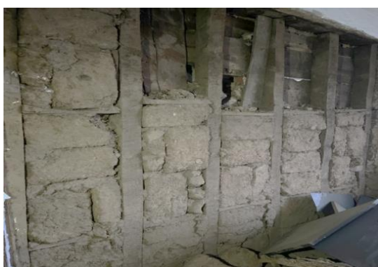
Figure 114: Timber (vertical and horizontal) elements filled with earth blocks (adobe)
