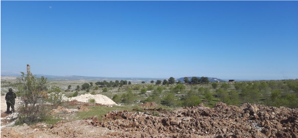
Figure 261: Örenli Permanent Housing Construction Site in Adıyaman province.
