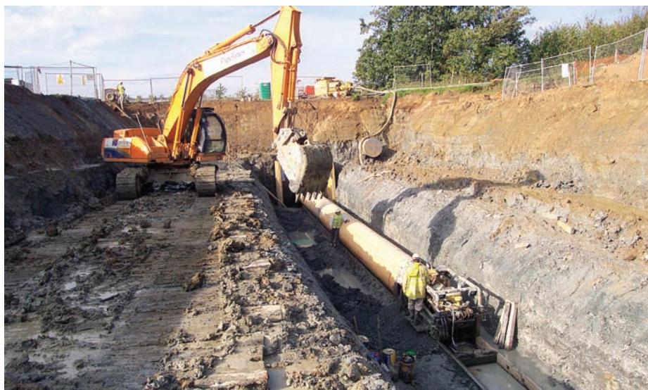
Figure 5 Installing replacement high pressure gas pipeline
