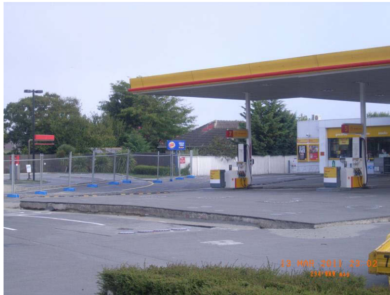
Figure 95 Floatation of a petrol storage tank
