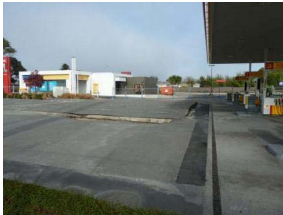
Figure 43 – A petrol station having suffered liquefaction. The underground storage tanks at this station have floated when the soil was in a liquefied state. The station was closed at time of survey.
