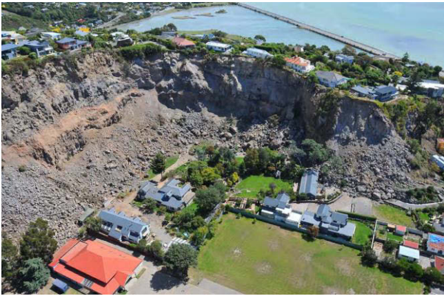
Figure 85 – Large rock falls from the quarried former sea-cliff at Redcliffs affected Redcliffs School and Moa Cave Guest House. The houses along the ridge on top of the slope in the right of the image experienced very intense ground shaking. (Taken by G Hancox, GNS Science)
