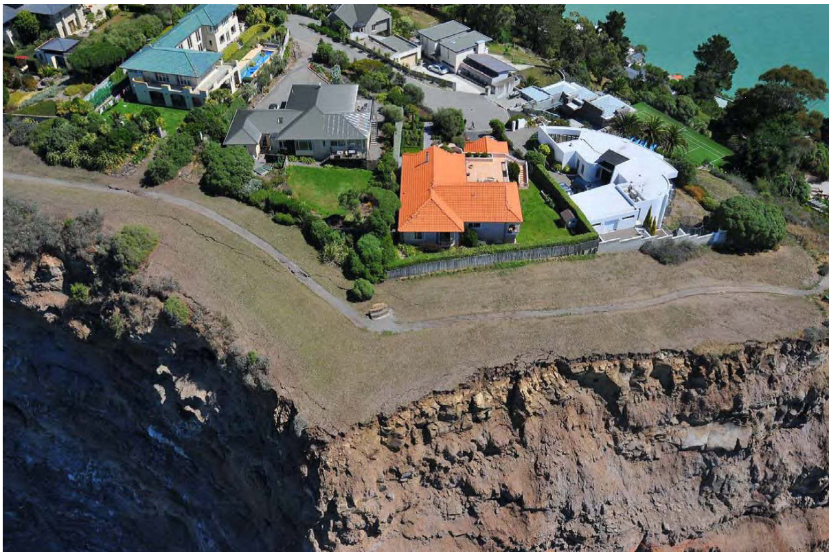
Figure 77 – Tension cracks affected the grass and path along the top of the 80 m high sea cliff at Sumner Head in the eastern Port Hills. NZTM 1581943, 5175709. Photo taken by Graham Hancox/GNS on 24 February 2011.
