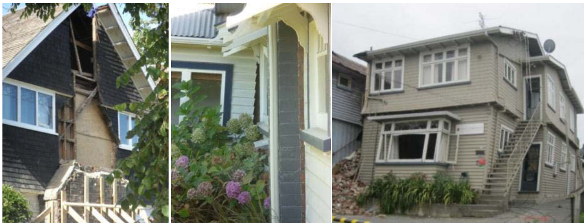
Figure 19 – (a) Collapse of a stone chimney breast on a timber frame house; (b) lateral spreading towards the river (left of photo) has resulted in differential movement and separation at the connection between the small extension and the main house; (c) soft storey failure at the ground floor level of a two storey timber frame house, as well as collapse of masonry facade.
