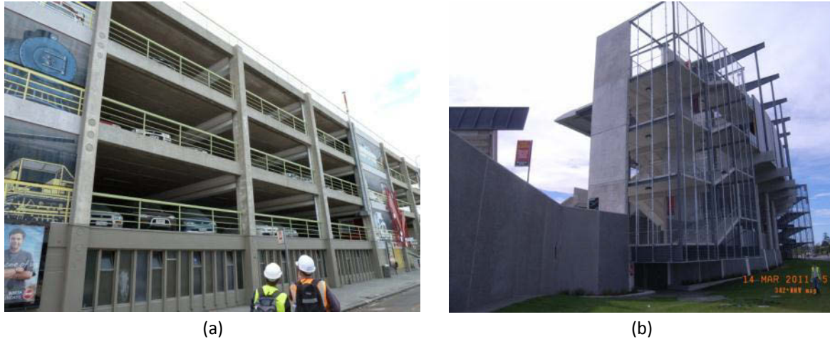
Figure 27 – Precast concrete structures. (a) Parking building on Gloucester Street with post-tensioned, precast beams, showing little damage. (b) AMI Stadium, with little damage visible from the outside (despite significant liquefaction), but reportedly damaged internally (The Press, 2011a).
