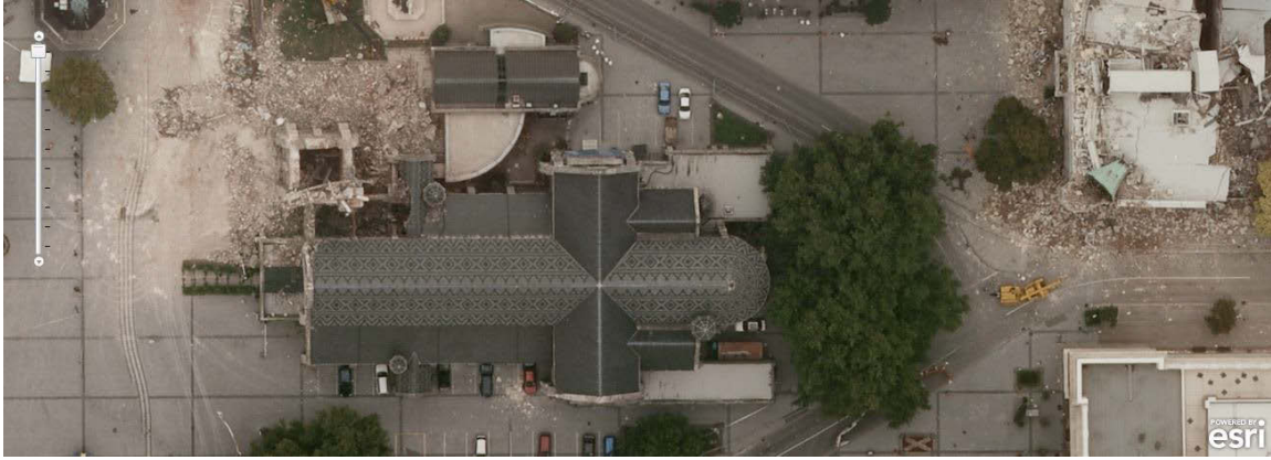
Figure 105 – Damage and debris around the Christchurch Cathedral (Source: NZAM, 2011 Creative Commons Attribution 3.0 NZ)
