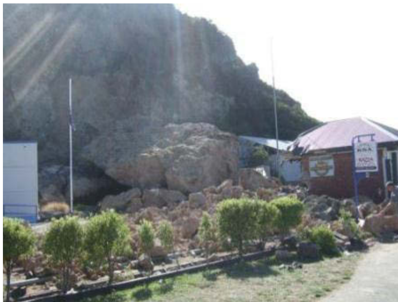
Figure 90 – A 15 m long boulder of tuff toppled from the quarried slope above the RSA building at the northern end of Wakefield Ave. The rock fragmented upon impact with the ground and some boulders bounced across Wakefield Ave for a distance of 60 m, twice the height of the slope.
