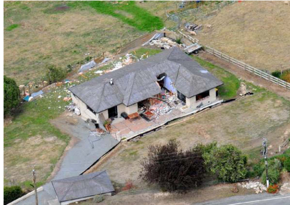
Figure 91 – A house at Governors Bay Rd, in Rapaki was hit by a boulder that had bounced 600 m from a bluff to the north west. (Credit: G Hancox, GNS Science).
