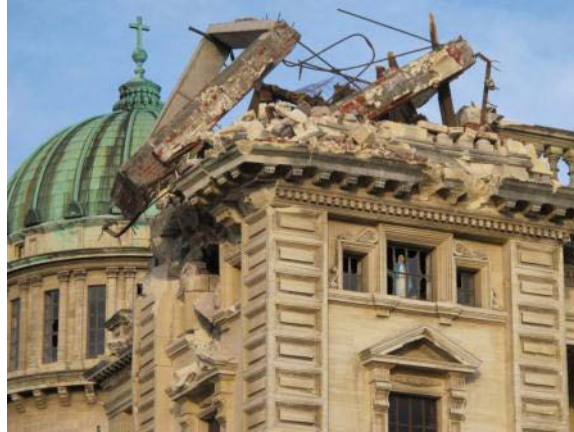
Figure 102 – One of Christchurch’s most notable heritage buildings, the Cathedral of the Blessed Sacrament, built in 1905. The cathedral was closed for repairs and seismic strengthening after the 4 September earthquake. The 22 February earthquake put the building on the demolition list.
