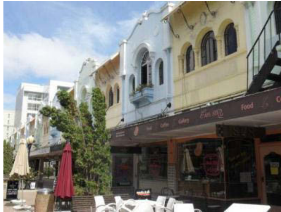
Figure 40 – Row of undamaged or lightly damaged RM buildings.
