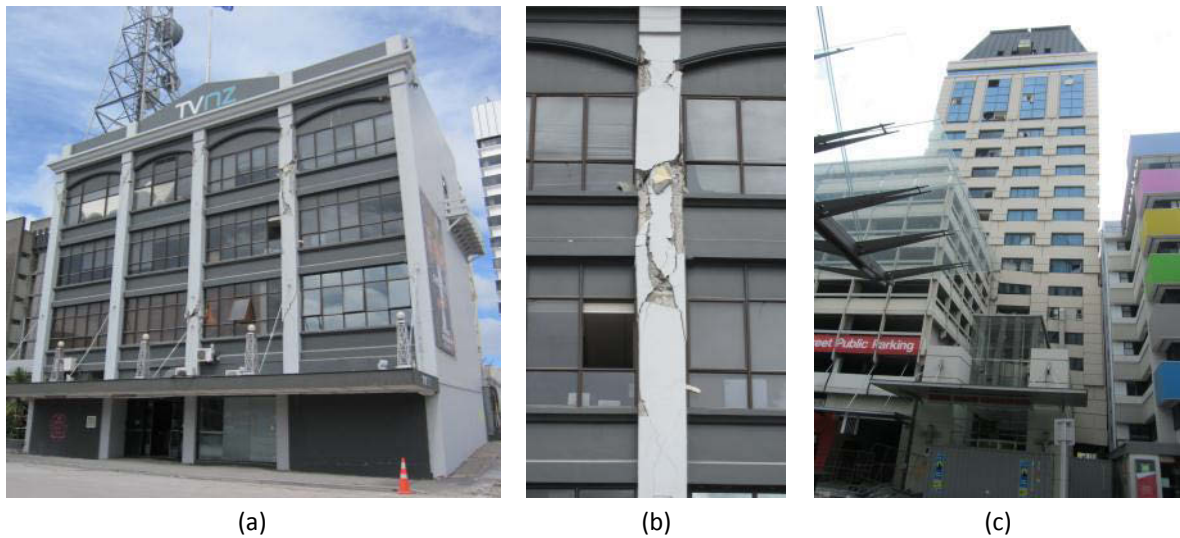
Figure 22 – Problems with structural irregularity. (a) and (b) TVNZ building with open street frontage and infilled frame at rear. (c) Grand Chancellor Hotel building, showing overhang of driveway at ground floor level.
