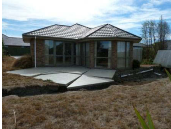
Figure 68 – Lateral spreading in the back yard of a house near the Bexley Wetlands
