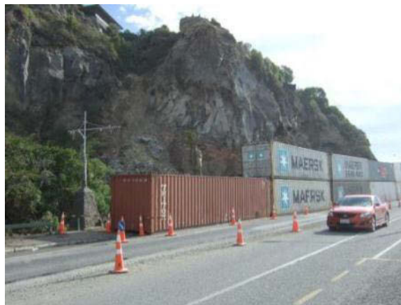
Figure 80 – Cargo containers temporarily placed between the cliff and Main Road to intercept any further falling debris. The rock fall debris obstructed the west bound (left) lane closing it to traffic.
