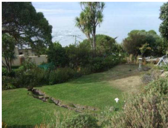
Figure 82 – a wide roughly north-south aligned tension crack (left) opened up in a landscaped garden south of Kinsey Terrace. A continuous GPS station seen in the far right of image was deployed by GeoNet/GNS Science, three days after the event and was sending near-real time slope movement data back to the office for interpretation by experts.
