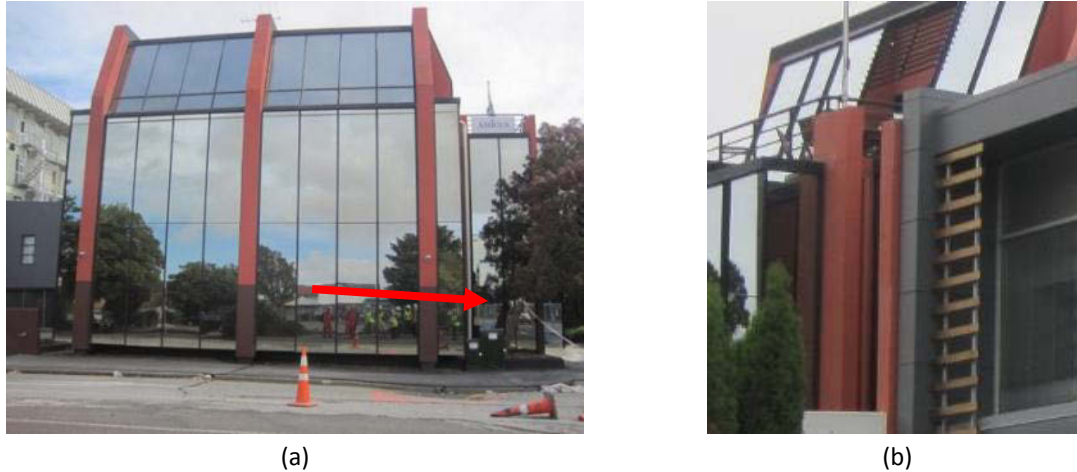
Figure 59 – (a) Building observed to have settled with the ground at one end. (b) Tilt relative to adjacent building. On this particular street, features such as sand boils, pavement compression, voids, and damage to buried services were concentrated near one corner of the building, indicating a localized area of slump (right side of part a).
