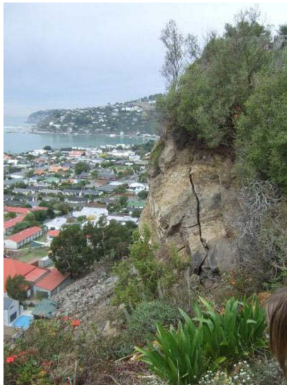
Figure 87 – Cracks along the tops of cliffs at Redcliffs.
