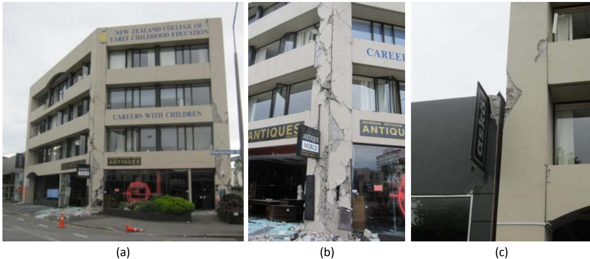
Figure 42 – Heavily damaged commercial RM building on Victoria Street. (a) Irregular layout led to (b) heavy concentration of demand on corner column. (c) Some damage due to pounding with adjacent building was also observed.
