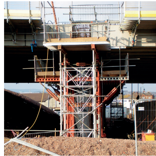
Figure 2 RMD Kwikform Megashor trestle support for precast beams
