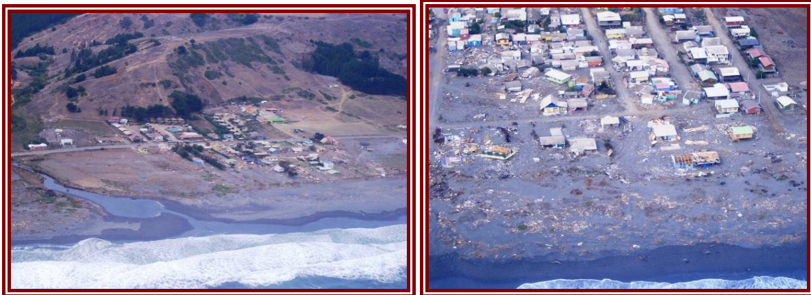
Figure 5-27: Severe damage to villages around Iloca
