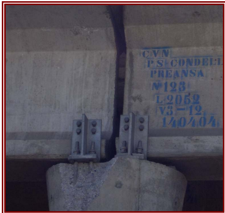
Figure 3-27: Damage to deck restraints. Figure 3-28: Spalling of concrete around holding down bolts
