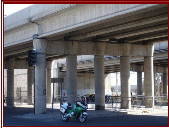
Figure 3-26: The middle set of overpass bridges.
