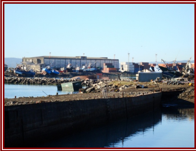
Figure 8-6: Talcahuano Port after the earthquake
