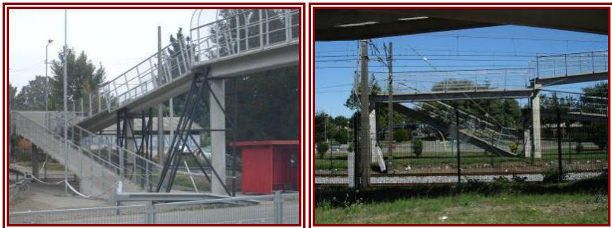
Figure 4-13: Typical footbridge failures
