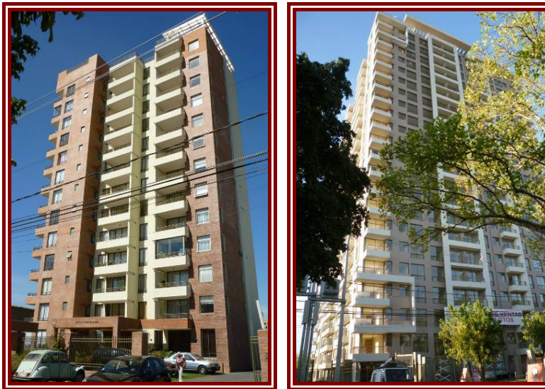
Figure 5-5: Typical undamaged apartment buildings in Talca: Edificio Costa Azul (left) and new building under construction on Av O'Higgins (right).
