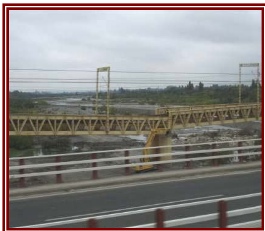
Figure 6-21: Badly damaged railway bridge
