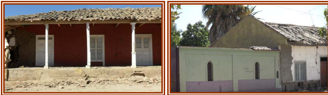
Figure 4-5: Left: Peralillo Adobe house with porch. The scarf joints on the beams are visible over the columns; the porch is connected with horizontal struts to the adobe wall, hence providing some lateral restraint. The central column in the picture has shifted laterally from its support. Right: townhouse with confined masonry end walls. The adobe façade shows vertical cracks and the roof as partially caved in, but is still supported.
