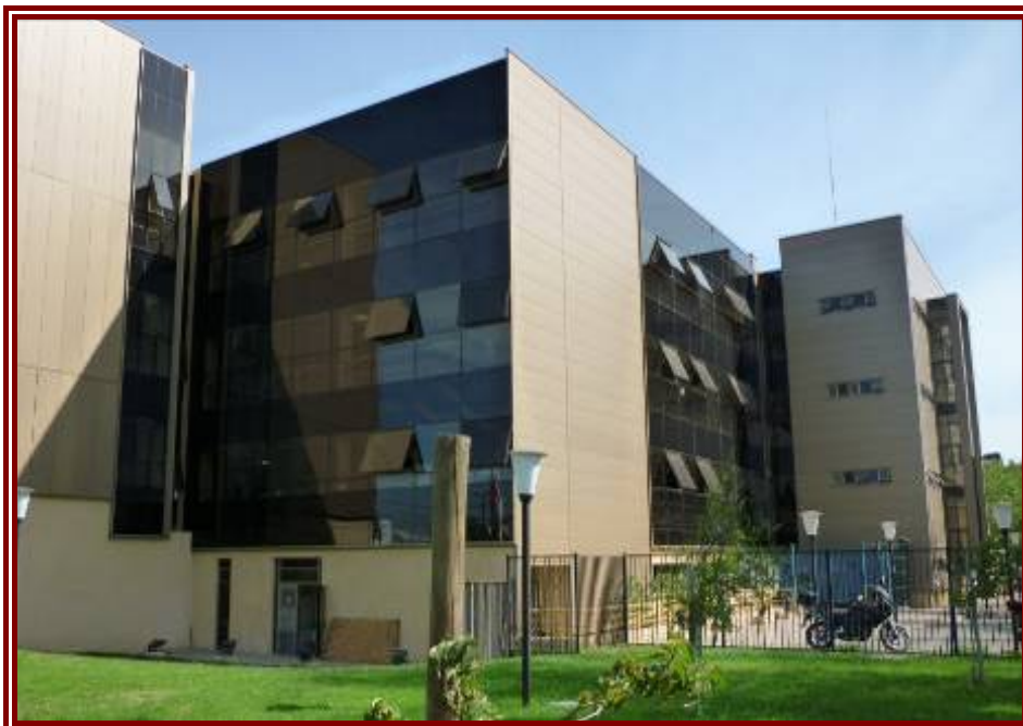
Figure 5-14: Damage to old hospital building and no discernable damage to modern hospital building in Talca
