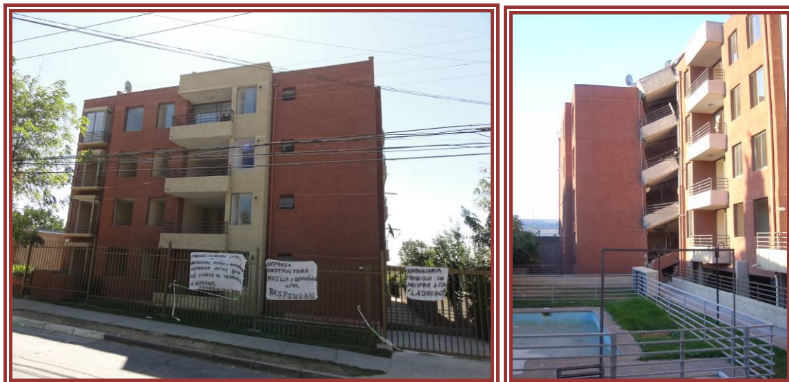
Figure 3-16: Another damaged apartment block in Maipu district, Santiago (general views)
