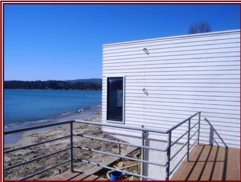
Figure 8-5: Timber top floor survived undamaged despite being completely submerged
