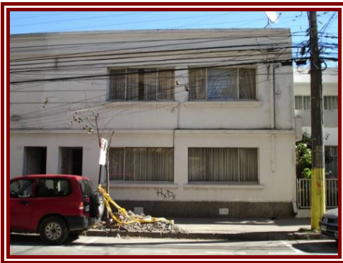
Figure 6-3: Example of rubble left outside a property indicating some level of damage internally but no obvious external damage
