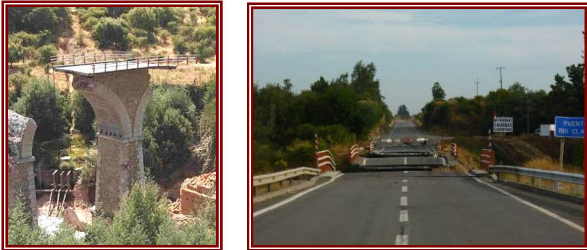
Figure 5-19: Rio Claro Bridge (southbound traffic) collapse
