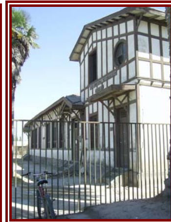
Figure 4-4: Peralillo, town house in adobe confined with wood columns (quincha) and the old school, with similar construction, which did not suffer any damage.
