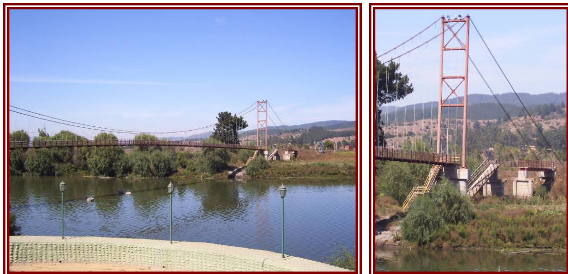
Figure 5-18: Suspension bridge failure, Lincantén
