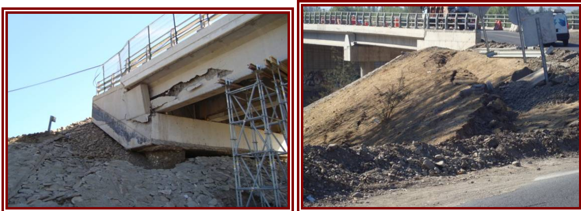
Figure 4-15: a) Bridge; b) Embankment along 5 Sur Road Santiago-San Fernando City
