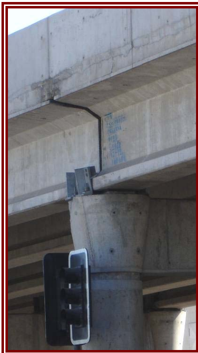
Figure 3-27: Damage to deck restraints. Figure 3-28: Spalling of concrete around holding down bolts
