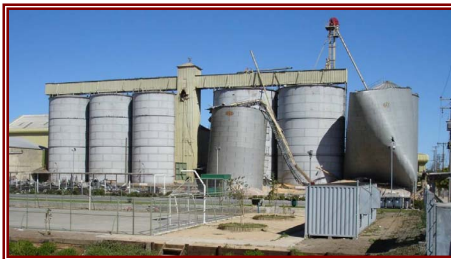
Figure 6-35: Damage to a complex of 14 grain silos showing severe buckling of one of the remaining silos. Differences in the construction of silos are also apparent.
