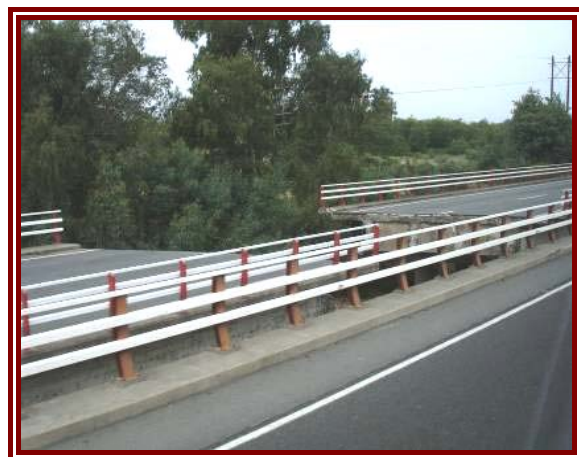
Figure 6-22: Collapsed skew span
