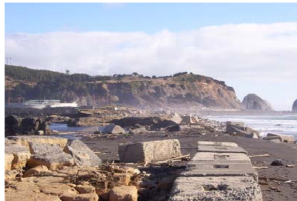
Figure 5-32: Seawall in front of the Auraco plant, before and after tsunami
