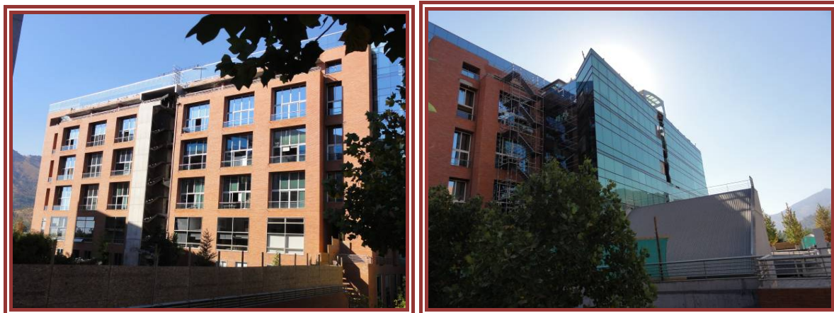
Figure 3-19: Damage to the stair cases and surrounding area in a modern building in Ciudad Empresarial, Santiago (part of stair case has collapsed in the left and similarly the glassy facade on the other side of the building was broken with differential displacement at both sides)
