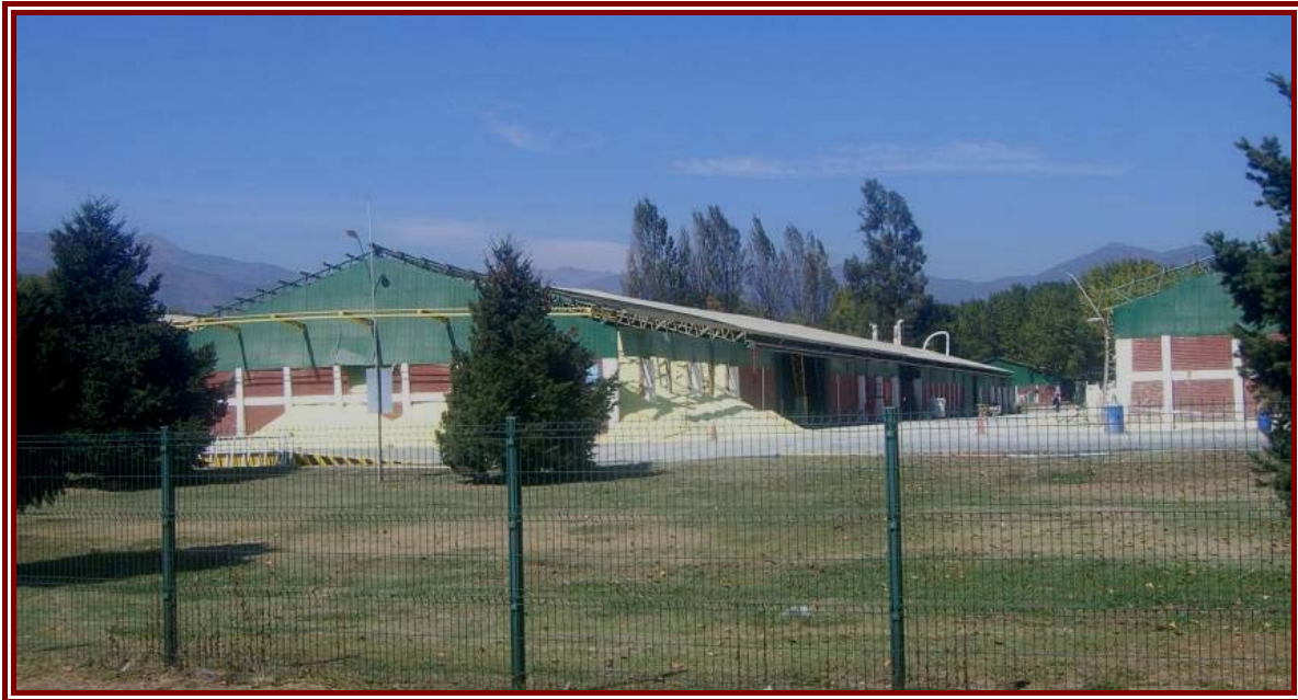
Figure 4-18: Damage to sulphur storage facility south of San Fernando
