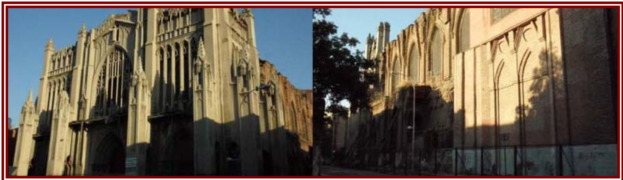
Figure 3-5: Western and southern elevation of the Basilica del Salvador
