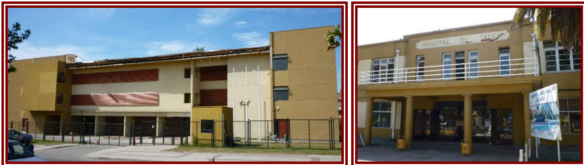
Figure 5-13: Damage to hospital buildings in Talca
