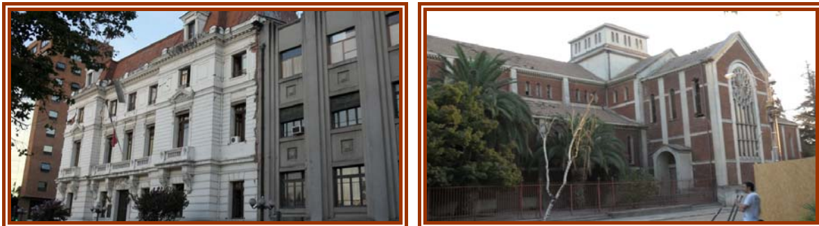
Figure 5-3: Left: example of hammering between to masonry buildings in Plaza mayor and right, Cathedral of Talca
