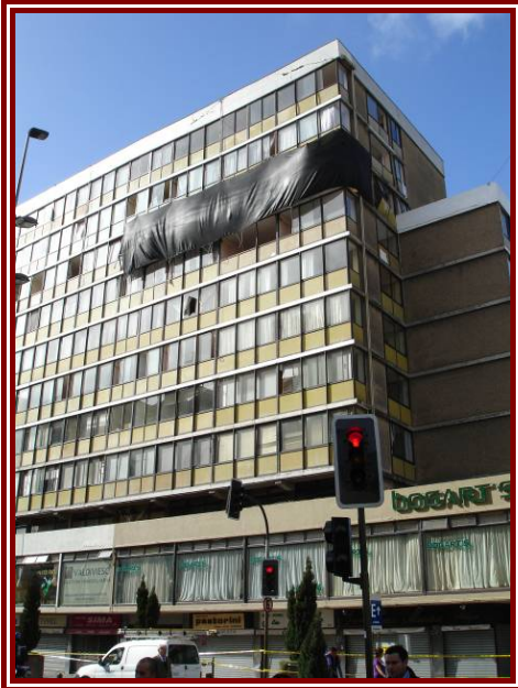
Figure 6-7: Damage to one corner of Caupolican 518
