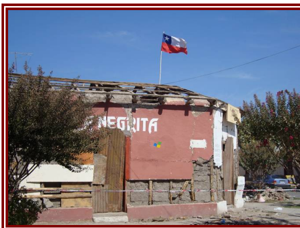
Figure 4-4: Peralillo, town house in adobe confined with wood columns (quincha) and the old school, with similar construction, which did not suffer any damage.
