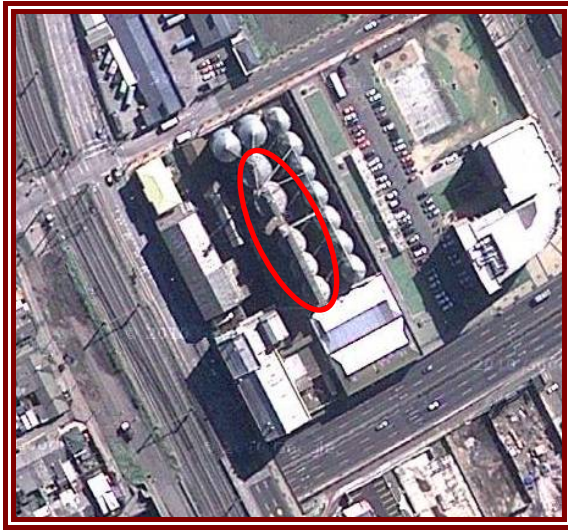
Figure 6-36: Aerial photo of site before earthquake, ringed silos appeared to be original
