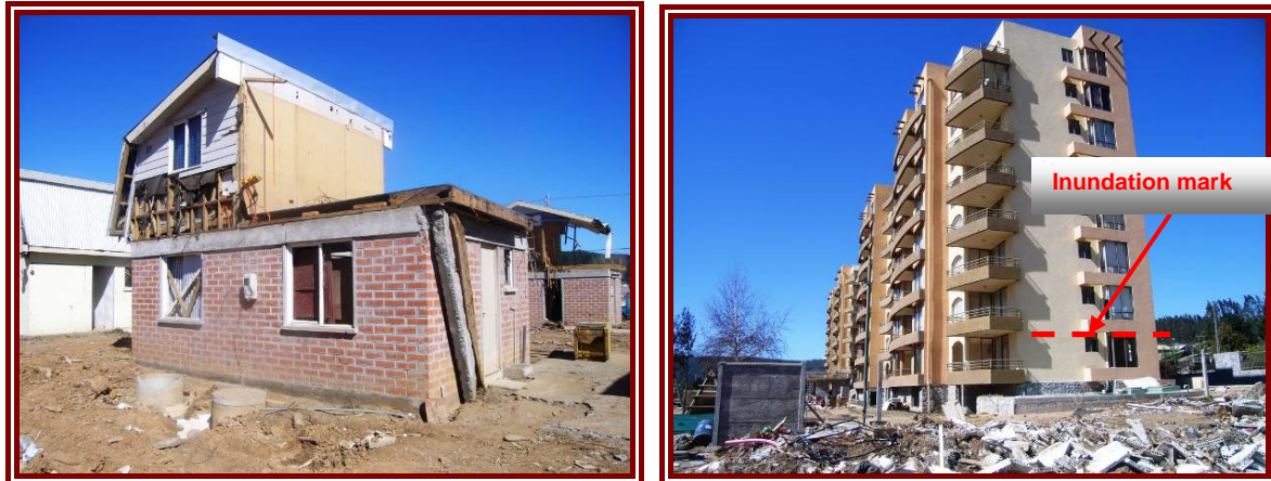
Figure 6-34: Damage to rows of housing, and tall structure, Dichato
