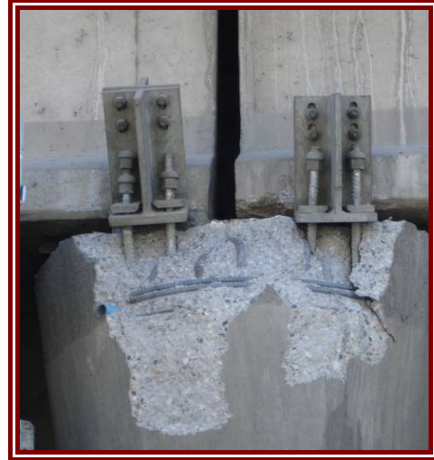
Figure 3-29: The northernmost set of overpass bridges. Figure 3-30: Severe spalling of concrete at holding down bolts
