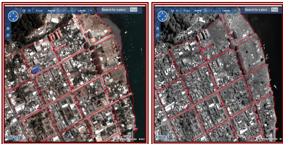
Figure 7-2 Constitución - Pre- and post- event satellite images of the site damaged by tsunami
