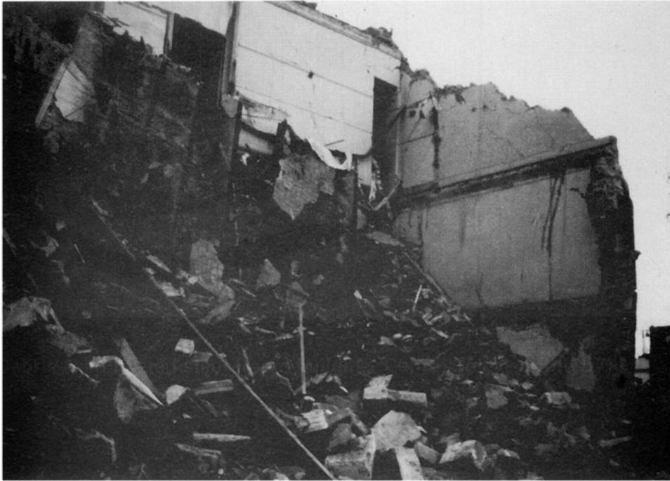
Failure in 3 storey masonry building with steel joists (Site 30)
