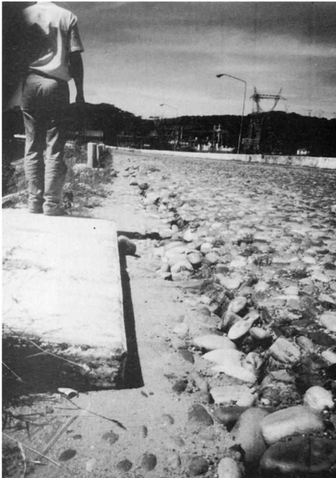
Crest of Jose Maria Morelos Hydro-electric Dam showing longitudinal cracks
