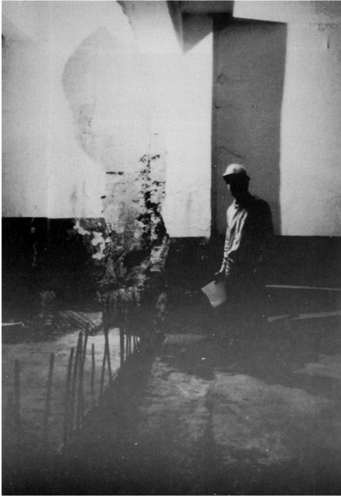
Ground slab joint at junction of eleven and four storey building
