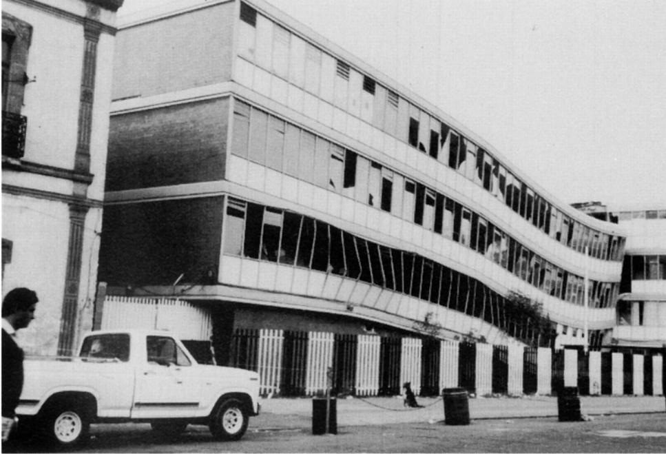
Soft ground floor failure, reinforced concrete building (Site 37)
