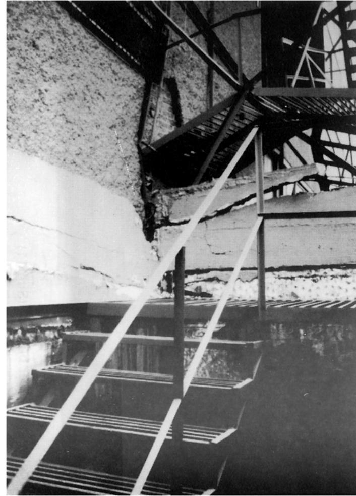
Staircase - Structural damage at joint of eleven and four storey building (Site 87)
