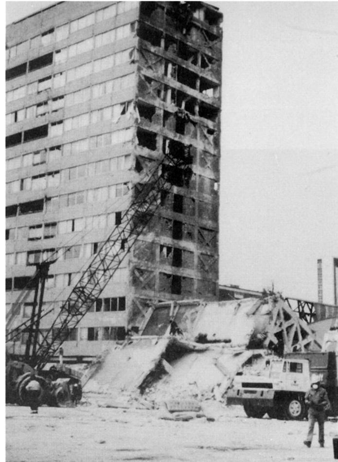
Failure of reinforced concrete x-braced Nuevo Leon Building, Tlatelolco estate (Site 4)
