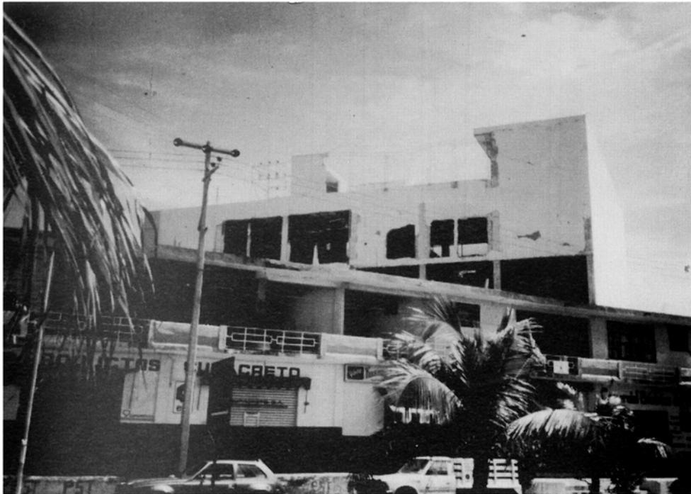
Damage to brick infill in 2 storey domestic structure at Lazaro Cardenas
