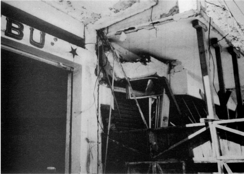
Damage to beam indicating standard of construction of domestic structures in Lazaro Cardenas
