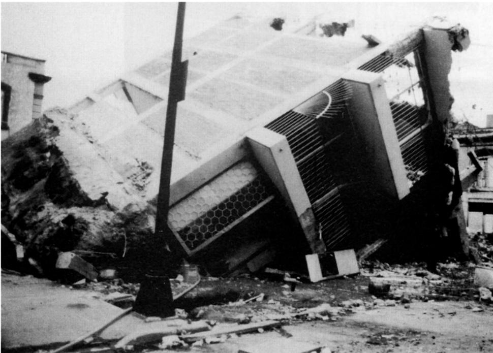
Foundation Failure by Rotation (Site 78)
