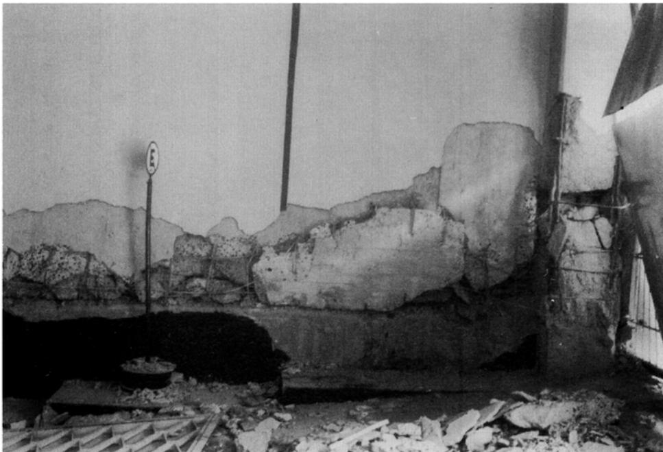
Failure in reinforced concrete shear wall (Site 58)
