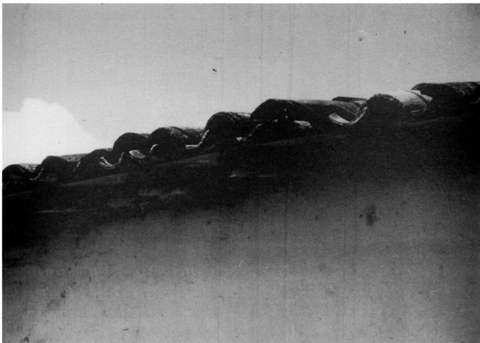
Typical roof construction of adobe building (Site 25)
