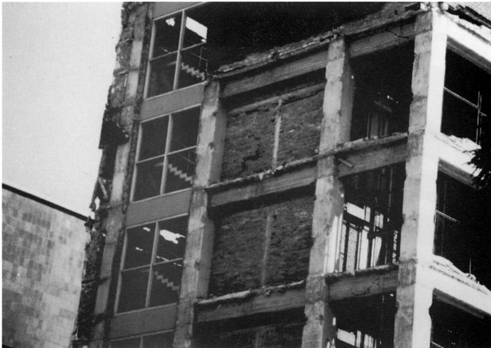
Failed infill with secondary columns and beams, Centro Medico (Site 85) PLATE **3.40**
