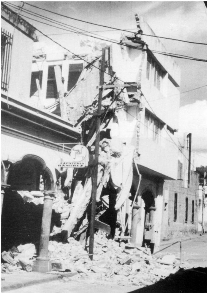
Failure in 3 storey reinforced concrete building (Site 20)
