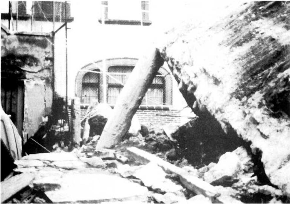
Foundation Failure by Rotation showing extruded pile (Site 78)
