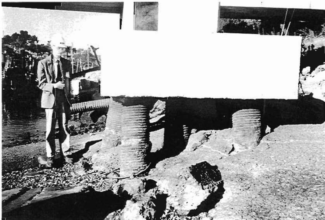
**Plate 5.21 : Murray Street Bridge - Cracking of surface cement slurry**
