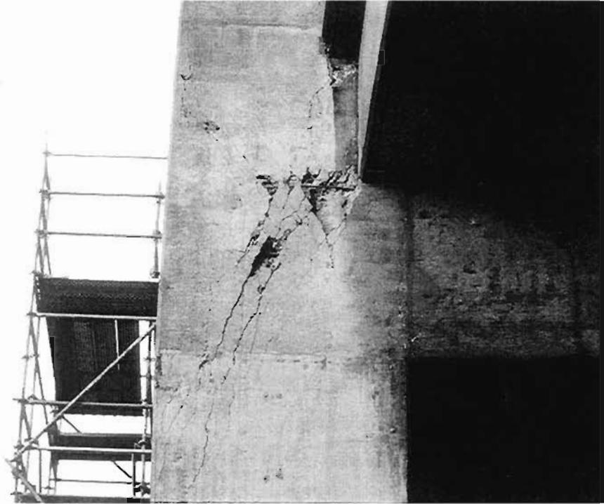
**Plate 5.7 : Embarcadero Viaduct - Concrete spalling at beam/column connection**
