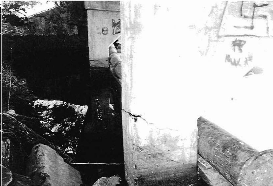
**Plate 5.17 : Cut Bias Bridge - North side column showing crushing and toe of adjacent fill**
