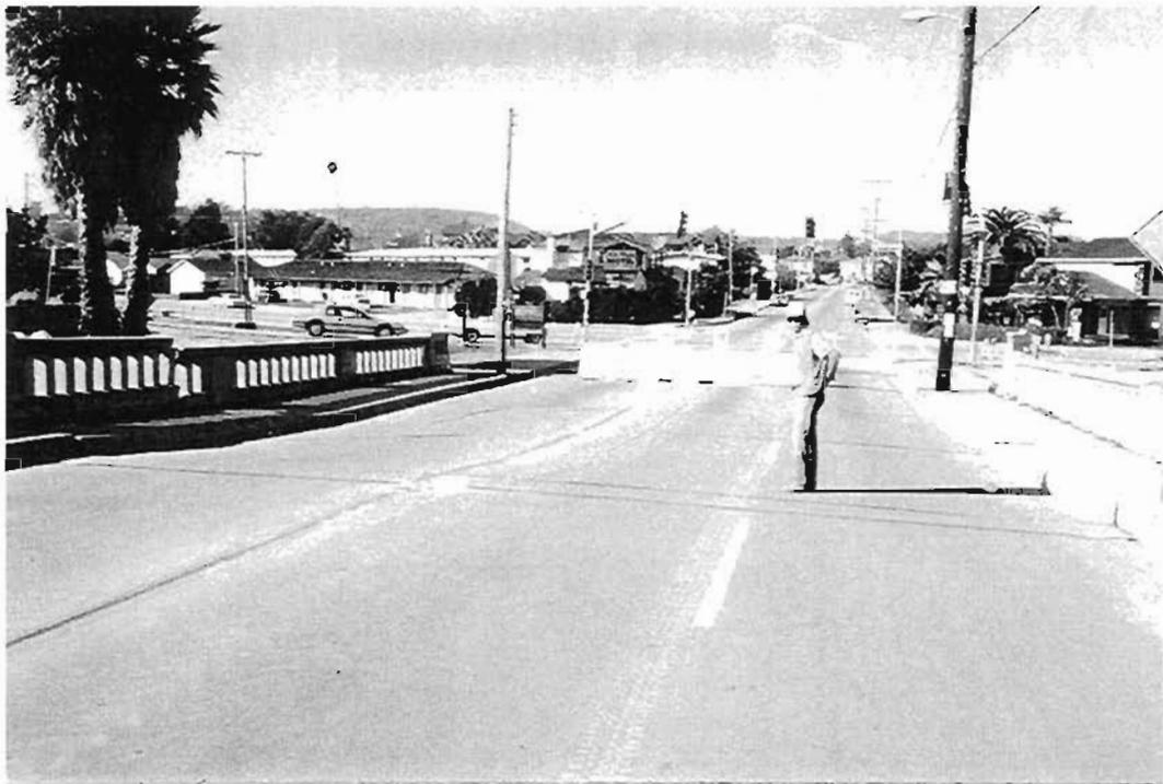
**Plate 5.14 : Riverside Avenue Bridge - Settlement of approach embankment**
