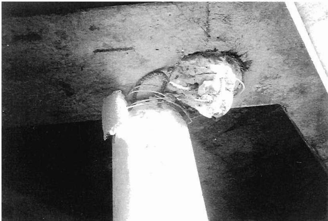
**Plate 5.25 : Struve Slough Bridge - Failed pile/deck joint, note inadequate spiral binding reinforcement**
