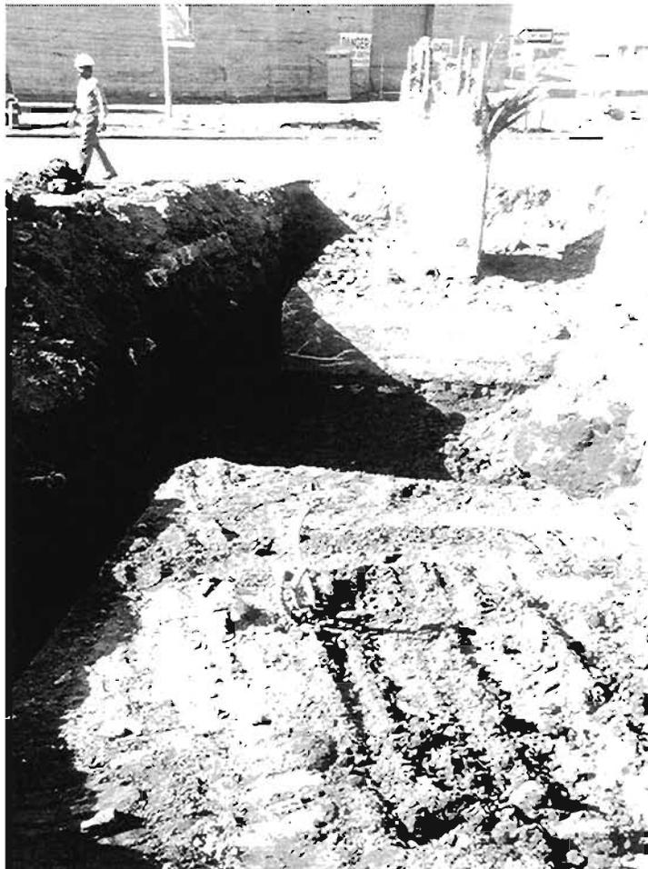
**Plate 7.7 : Excavated pile cap on the Nimitz freeway**
