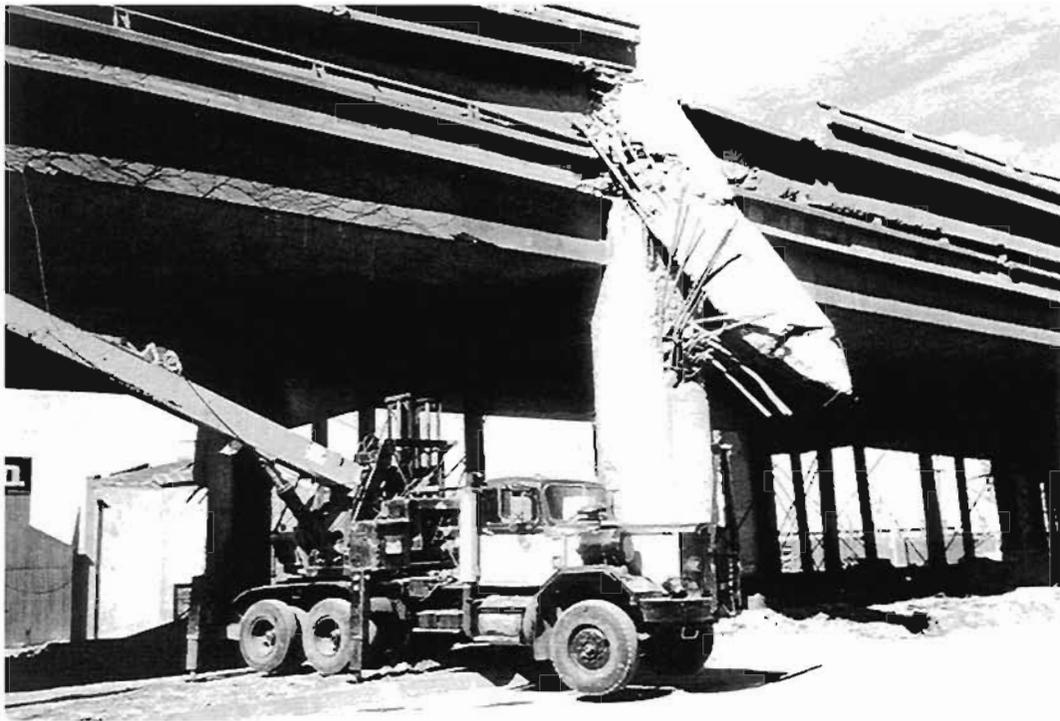
**Plate 5.3 : Cypress Street Viaduct - Typical brittle failure of upper column**
