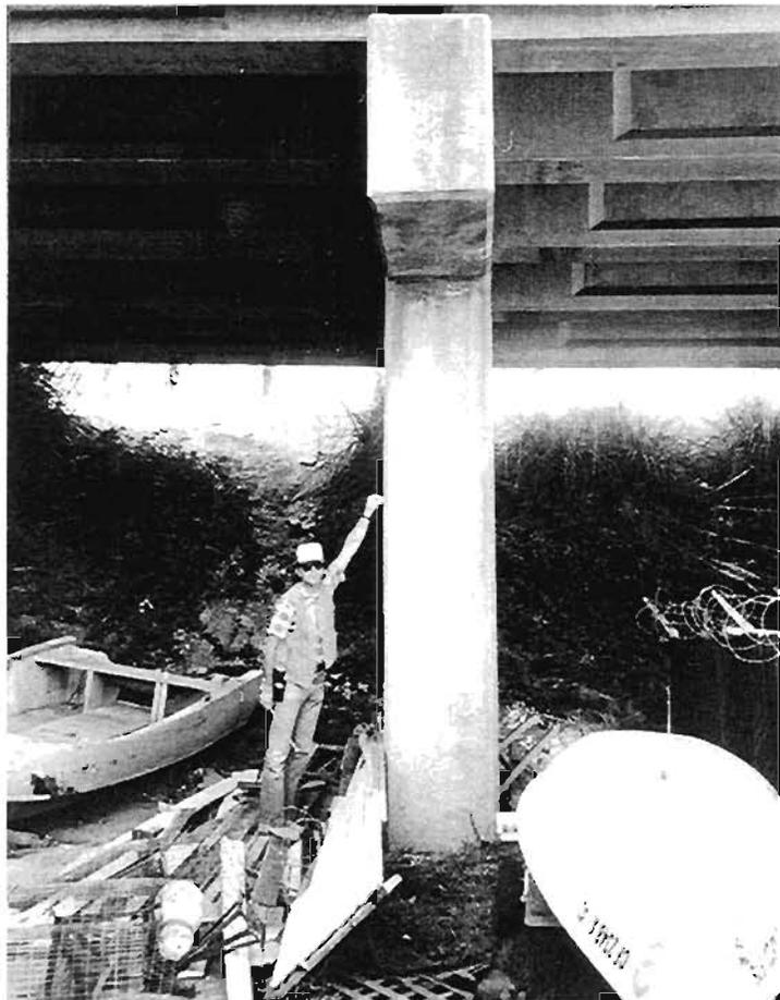
**Plate 5.19 : Murray Street Bridge - West pier showing Brian Evans holding plumb line**
