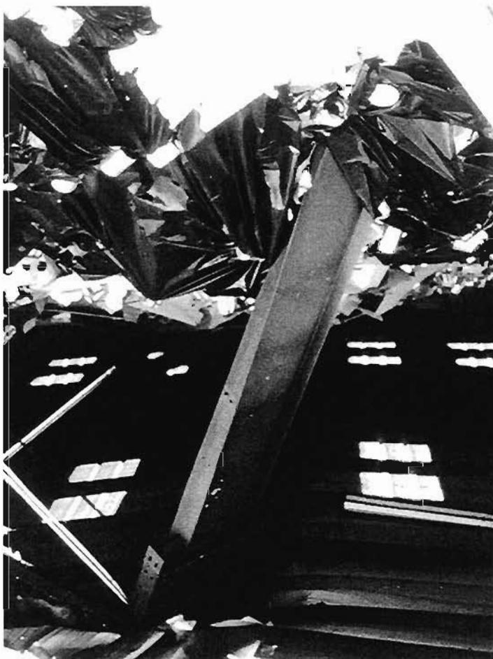
Plate 6.10 : Hollister - Twisted Column on Metalclad Warehouse
