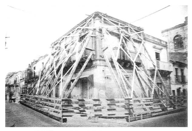
PLATE 5 Temporary shoring and safety barriers around a damaged building
