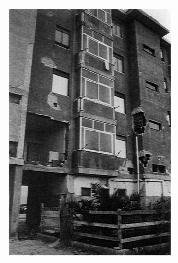
PLATE 15 Failure (out of plane) of reinforced masonary infill panels
