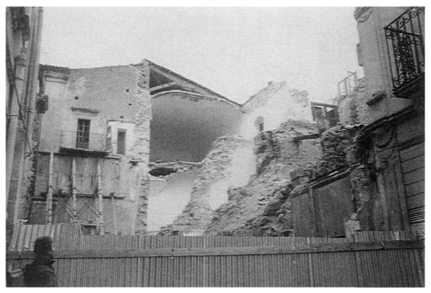
PLATE 7 Out of plane wall failure - Noto
