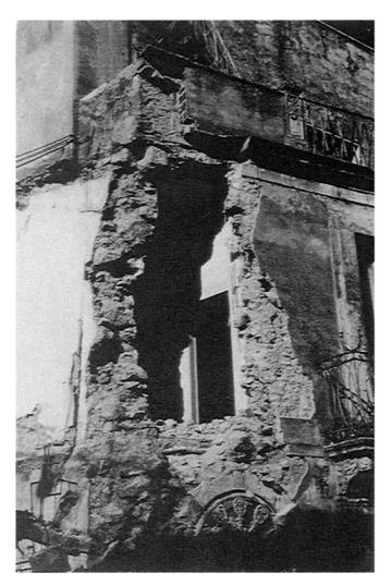
PLATE 8 Typical corner failure - Melilli
