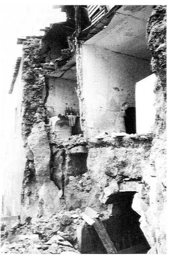
PLATE 6 Out of plane wall failure - Noto
