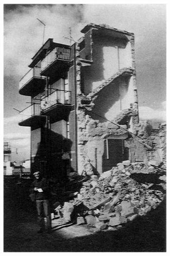
PLATE 13 Collapse of three storey residential building in Carlentini
