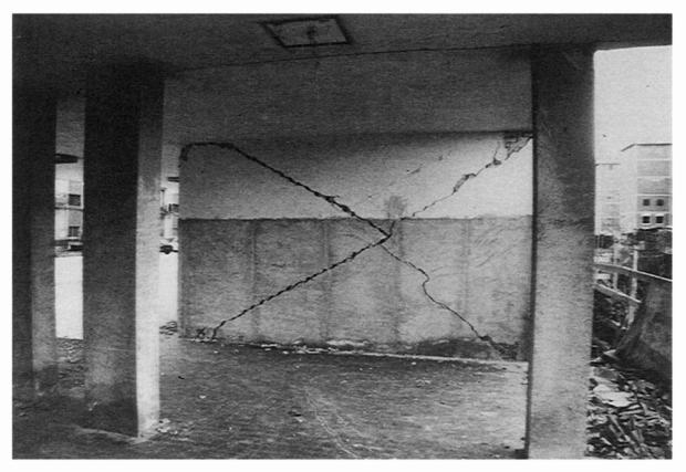
PLATE 16 Shear failure of stairwell at ground level - Augusta
