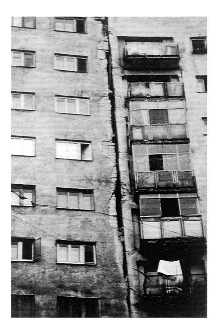
Plate 4: Colentina district, damage down the seismic gap line, due to pounding.
