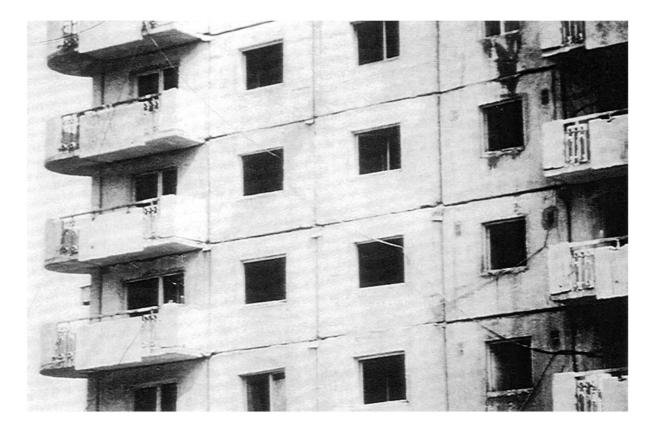
Plate 17: Detail of connections in an RC large panel building under construction.
