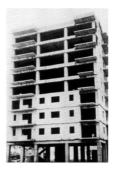
Plate 12: Monolithic RC frame building with RC wall panels instead of infill masonry (Location: Focsani).
