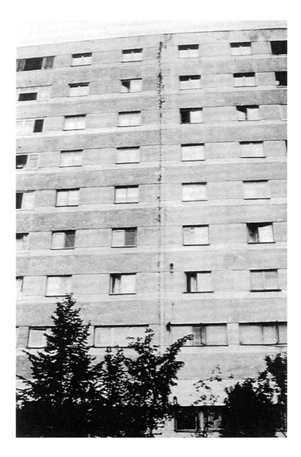
Plate 24: Damage to the expansion joint (Location: Buzau survey).
