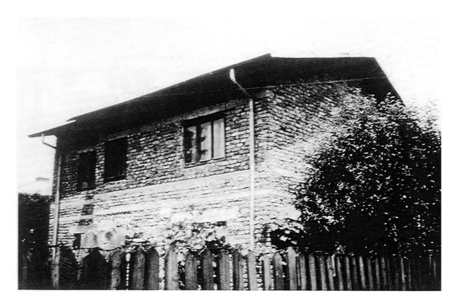
Plate 9: Two storey brick masonry house with RC slab, RC lintels and ring beam in the ground floor.
