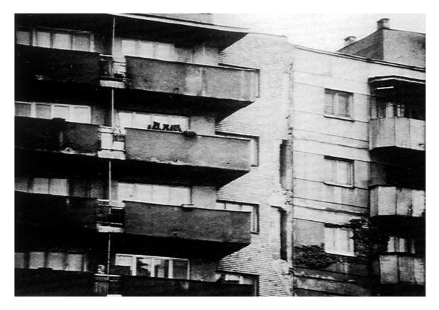
Plate 5: Damage to the expansion joint in another part of Bucharest.
