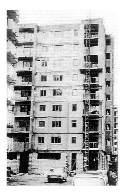
Plate 15: Three types of frame infill in a single building due to material supply shortage (Location: Focsani).
