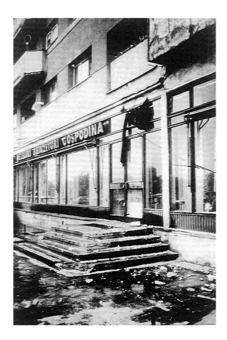
Plate 3: The unfortunate location of the entrance of the store, exactly along the seismic gap line contributed to the death of the two people, who were trying to run out of the building.
