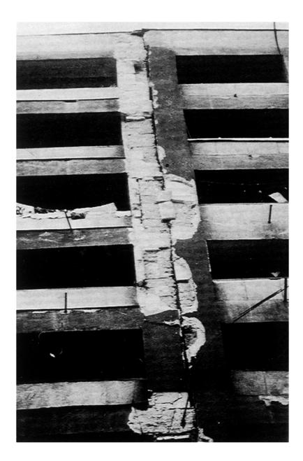
Plate 2: Close view of the collapsed plasterboard along the seismic gap line.
