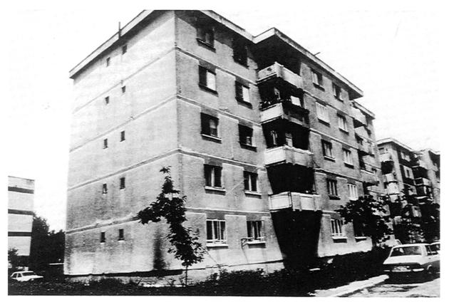
Plate 10: Typical 5 storey confined masonry apartment building, more commonly found in zones of intensity VI and VII.
