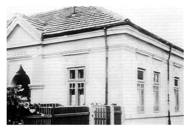
Plate 19: Typical single storey brick masonry building in the Buzau survey.
