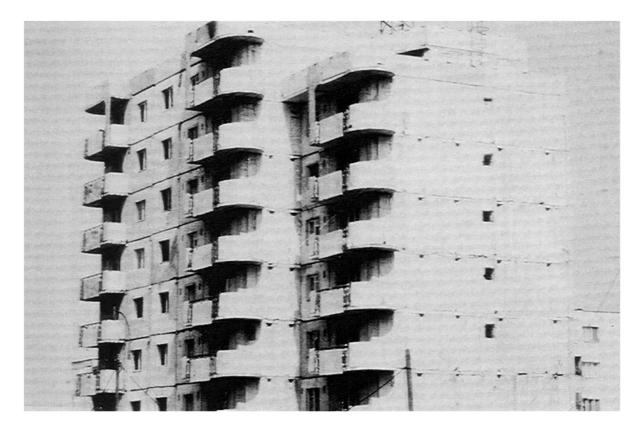
Plate 18: RC large panel construction before plastering. Notice the poor details in the connections.
