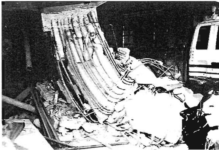
Plate 4.185: Collapsed column initiated by shear failure at base
