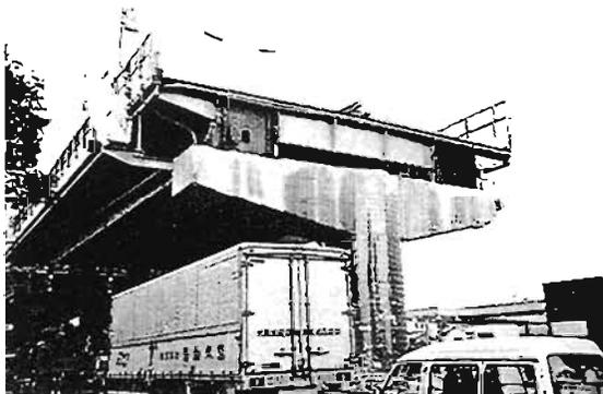
**Plate 6.3** Hanshin Expressway near Nishinomiya: Large movement at joint caused span to slip off bearing shelf. It was here that a tour bus came to a halt overhanging the abyss left by the missing span.
