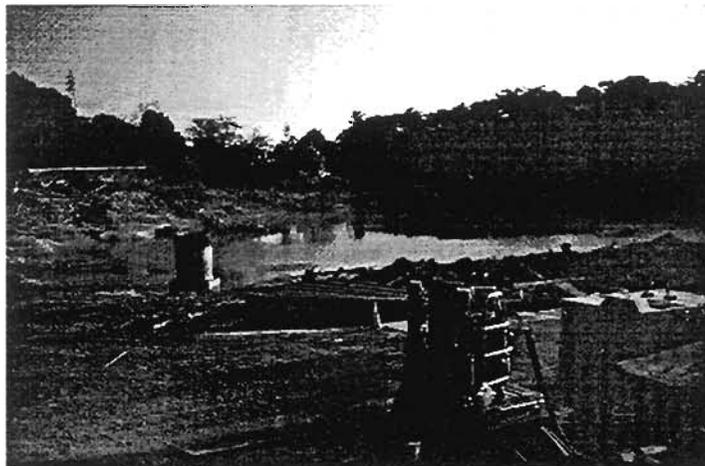
Plate 8.38: Liquefaction failure of the Niteko reservoir
