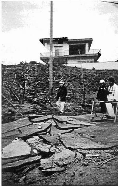
Plate 3.4: Pavement rupture due to the movement of the Nojima fault at Okura, Awaji Island
