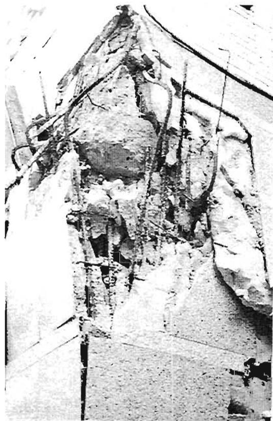
Plate 4.49: Exploded corner column joint
