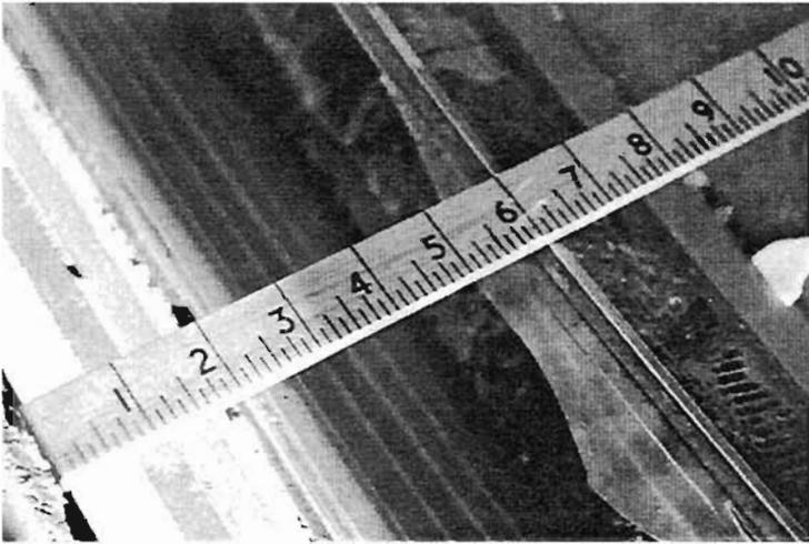
Plate 4.163: Width of seismic joint after earthquake
