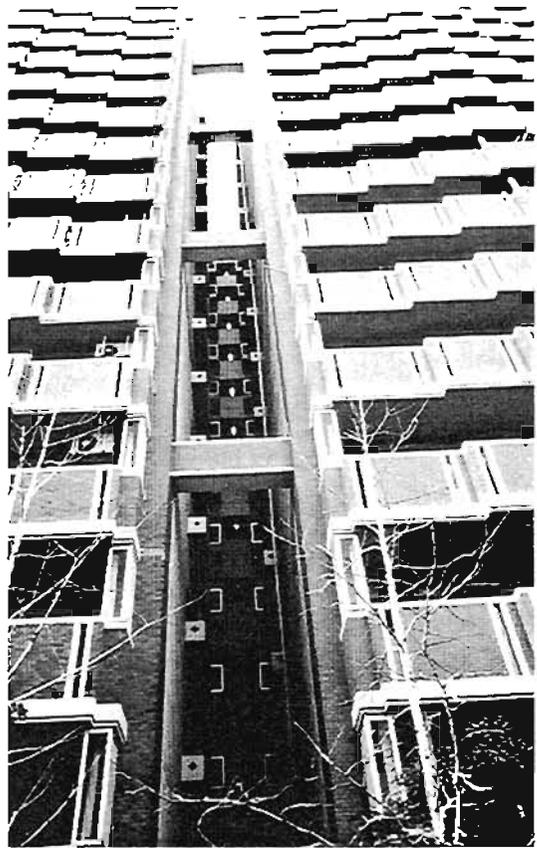
Plate 4.53: Seismic props to prevent diaphragm distortion
