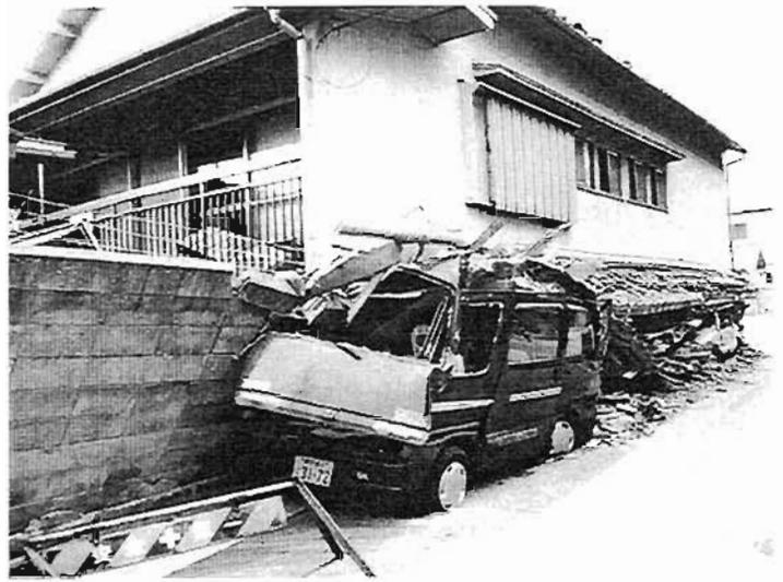
Plate 4.102: Collapse of steel frame building with soft storey
