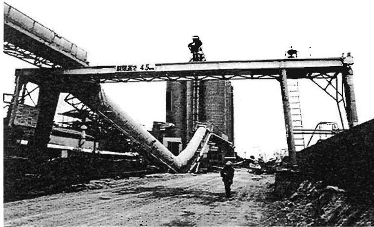
Plate 7.37 Collapsed section of conveyor
