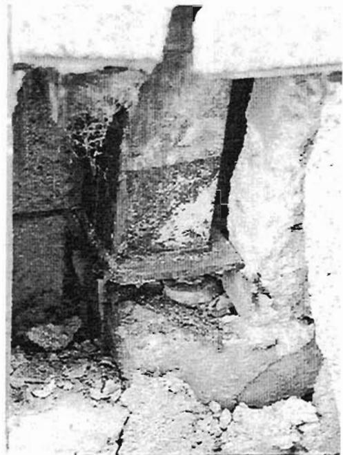
Plate 4.82: Disintegrated plinth of corner column
