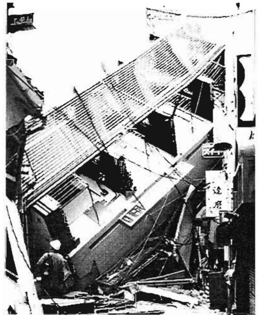
Plate 4.71: Overturning attributable to inadequate HD bolts
