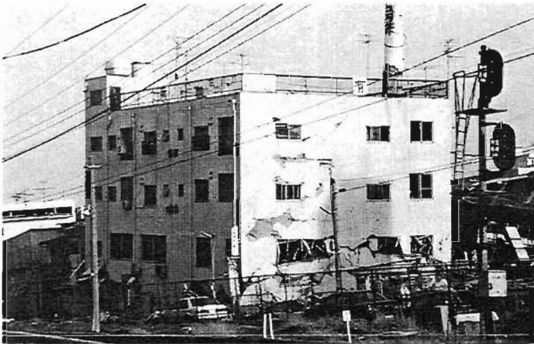
Plate 4.109: Local failure at long 1st floor window of building recessed into sloping site
