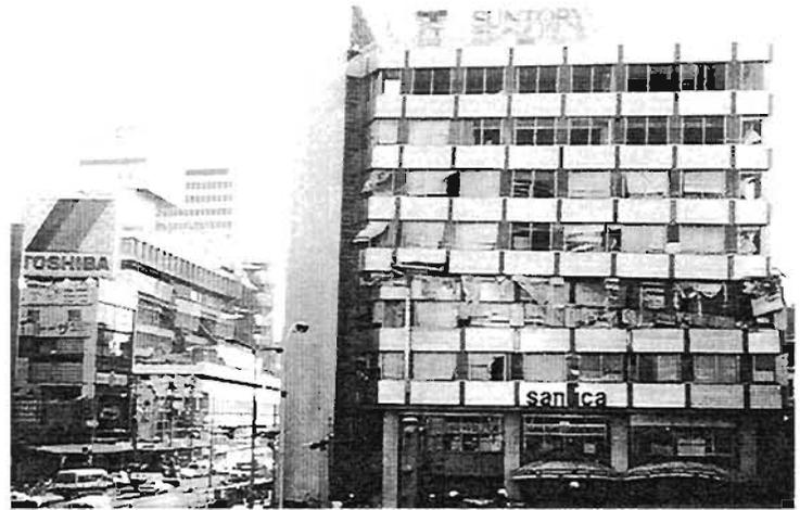
Plate 4.14: 4th and 5th Storey collapse in 9 storey building
