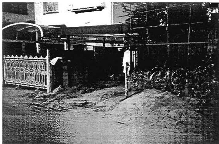
Plate 8.30: No apparent damage to the foundation of a house even large amount of erupted sands
