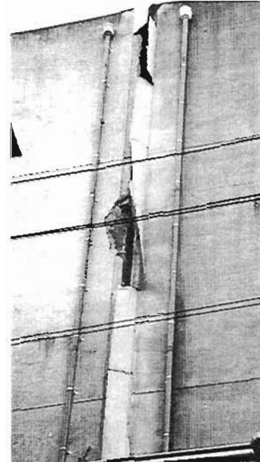
Detail of Plate 4.106 showing damage at expansion joint
