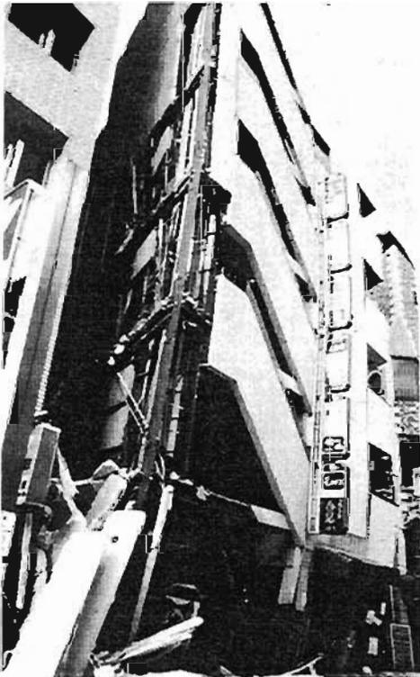
Plate 4.70: Sway after apparent failure
