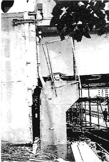
**Plate 6.62** Steel Box Girder Road Bridge over Canal, Kobe Ground either side of canal moved towards canal shortening span. Abutment wall moved forward and buckled flange and web of box girder.
