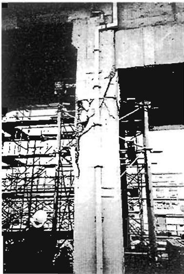
**Plate 6.37** Shinkansen Bullet Train Line Viaduct, near Nishinimoya shear-flexure failure at beam/column connection
