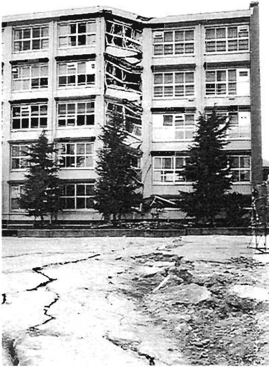
Plate 4.18: Partial storey collapse in 2nd storey
