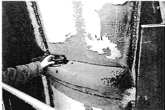
**Plate 6.55** Ramp onto the Hanshin Expressway to the west of Kobe Close-up of damage to column in Plate 6.54 - extensive buckle and rupture of pier wall
