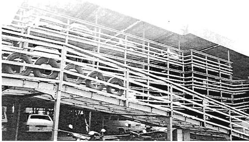
Plate 4.135: Undamaged flimsy and flexible car park
