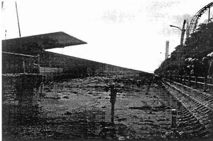
Plate 8.13: Erupted sand deposits found at the boundary between Phase 1 and 2 sections of Port Island
