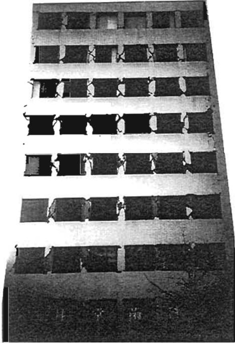
Plate 4.4: Distributed RC mullion damage due to minimal damage in corner mullions
