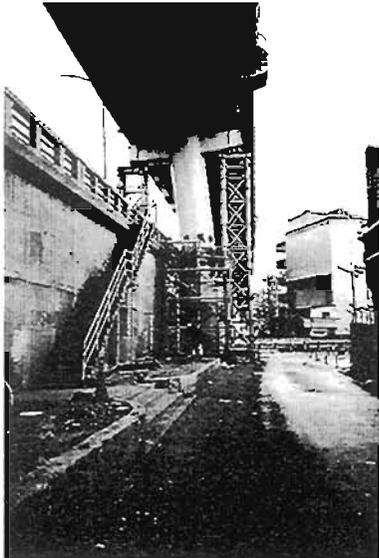
**Plate 6.54** Ramp onto the Hanshin Expressway to the west of Kobe Steel column kinked at change in wall thickness near mid-height. Stabilised by welding on T-section "splints" .
