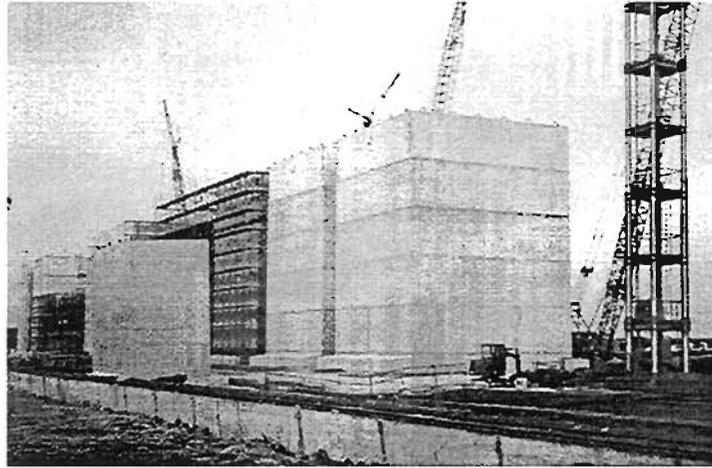
Plate 8.7: Typical concrete caisson walls used for Port Island
