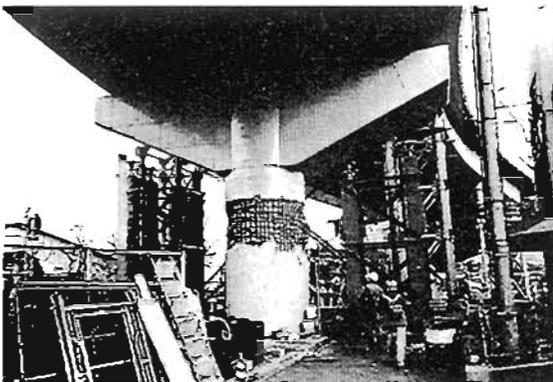
**Plate 6.33** Hanshin Expressway, Kobe: Shear-flexure failure at mid-height where main reinforcement is curtailed
