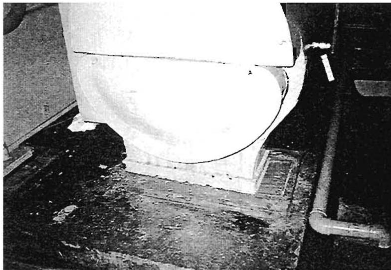
Plate 7.26 Poorly anchored pump, sliding at base
