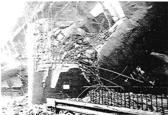
**Plate 6.25** Hanshin Expressway, Kobe Route 3, Fukae-Honcho Section close-up of pier in foreground of Plate 6.22 showing small lateral bars and curtailed longitudinal bars.
