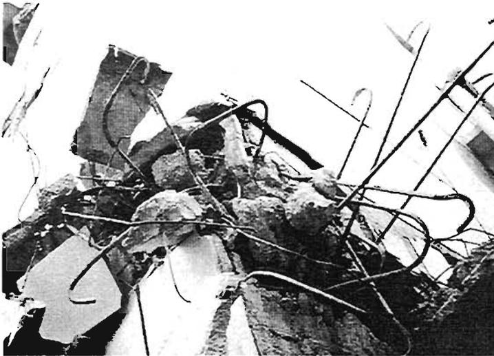
Plate 4.41: Disintegrated corner with reinforced fascia panels
