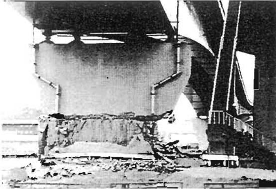
**Plate 6.39** East Pier of the Maya Ohashi Bridge on the Harbour Highway no through-wall ties, simply transverse bars which were lost with the cover. At least the longitudinal reinforcement was continuous.
