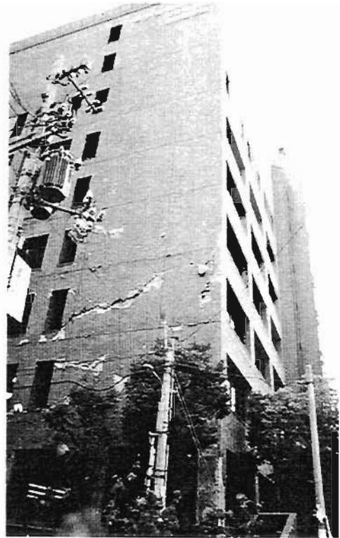
Plate 4.23: Damage to shear walls from separated masonry
