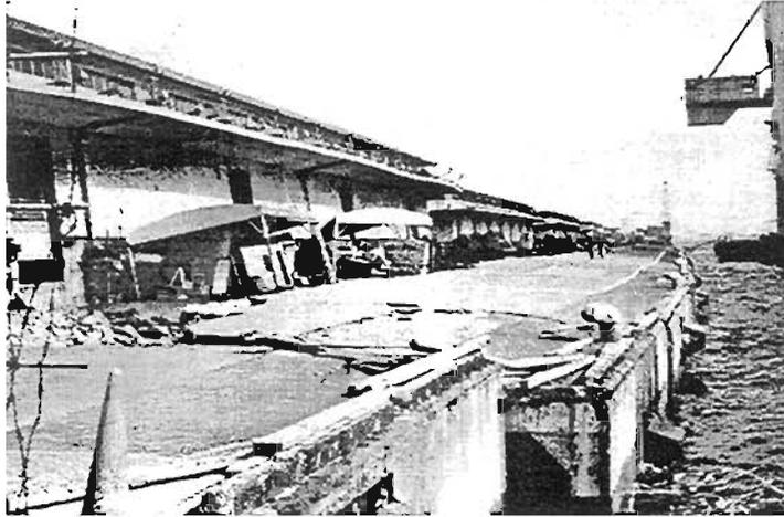
Plate 8.16: Lateral movement of concrete caisson walls at the Shinko Pier in Port Kobe
