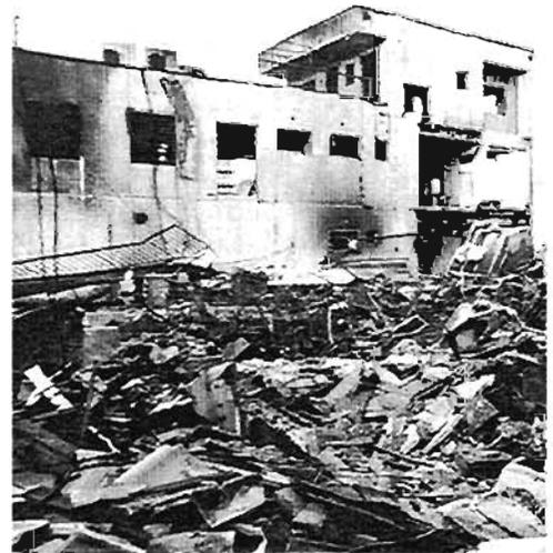
Plate 4.165: Combined fire and earthquake damaged building
