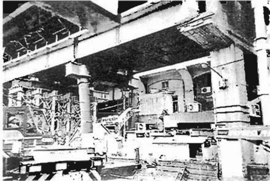
**Plate 6.58** Railway near Centre of Kobe - Damage to Steel Portal Pier centrifugally cast columns lacked ductility
