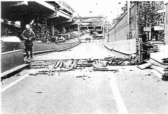
**Plate 6.11** Ramp onto Hanshin Expressway near centre of Kobe: Approximate one metre shift of first ramp span towards the north
