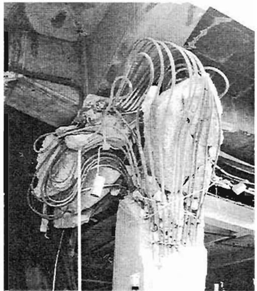
Plate 4.182: Collapsed anvil
