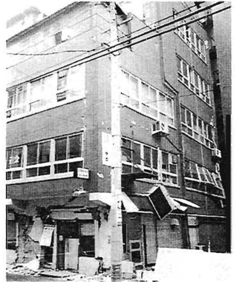
Plate 4.50: Irregular building damaged front and back
