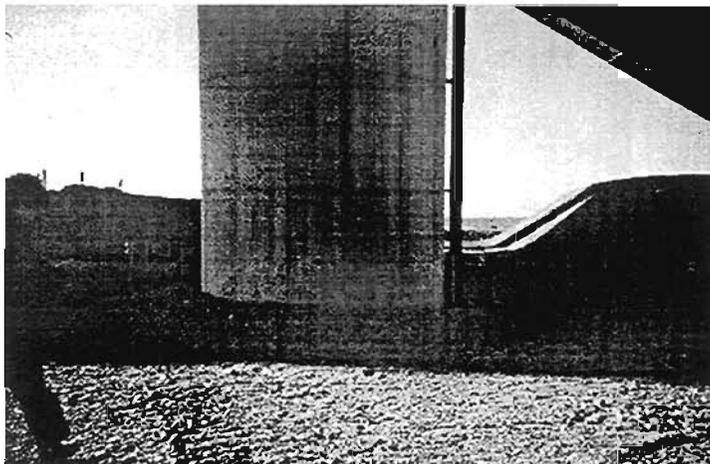
Plate 8.27: Lateral movement of the surface ground pushing the pier of the Nishinomiya Bridge
