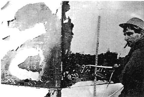
**Plate 6.50** Hanshin Expressway - Damage to Circular Steel Pier Column freshly flaked paint on column near Kobe centre indicates strong north-south cyclic action
