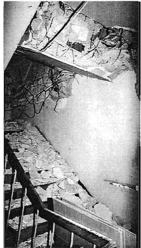
Plate 4.43: Landing beam punched through supporting wall
