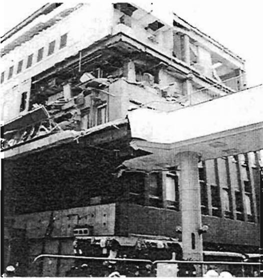
Plate 4.89: SRC building damaged by link bridge
