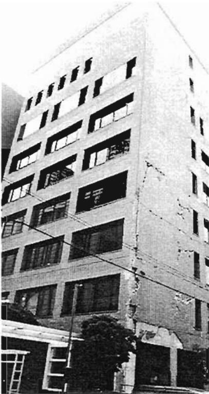
Plate 4.22: Spalling attributable to lack of longitudinal shear walls
