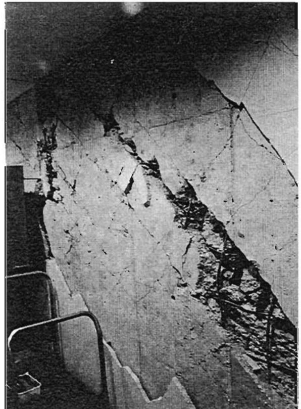
Plate 4.37: Shattered shear wall
