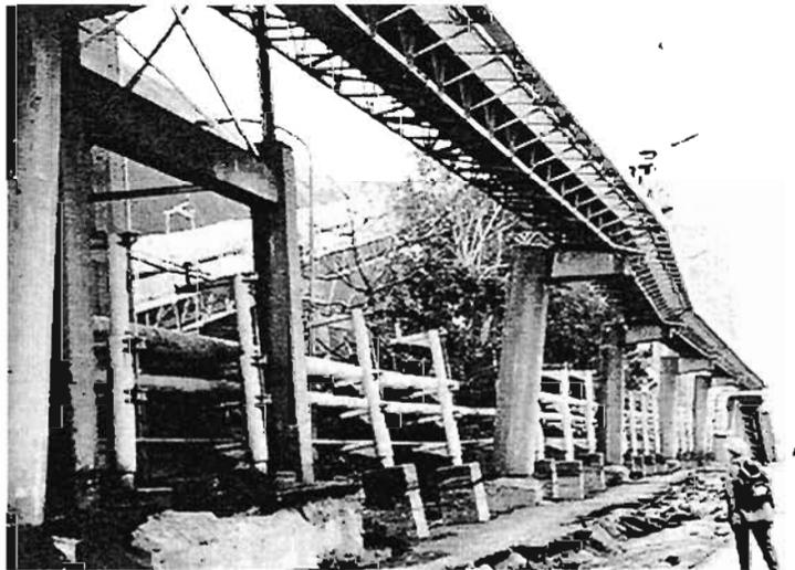
Plate 7.36 Overhead Conveyor with ground settlement
