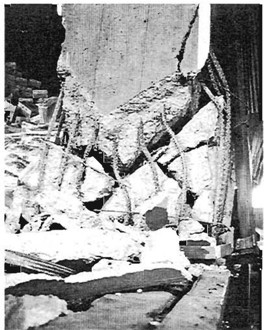
Plate 4.184: Anvil in shear hinge and incipient spreading of column beneath
