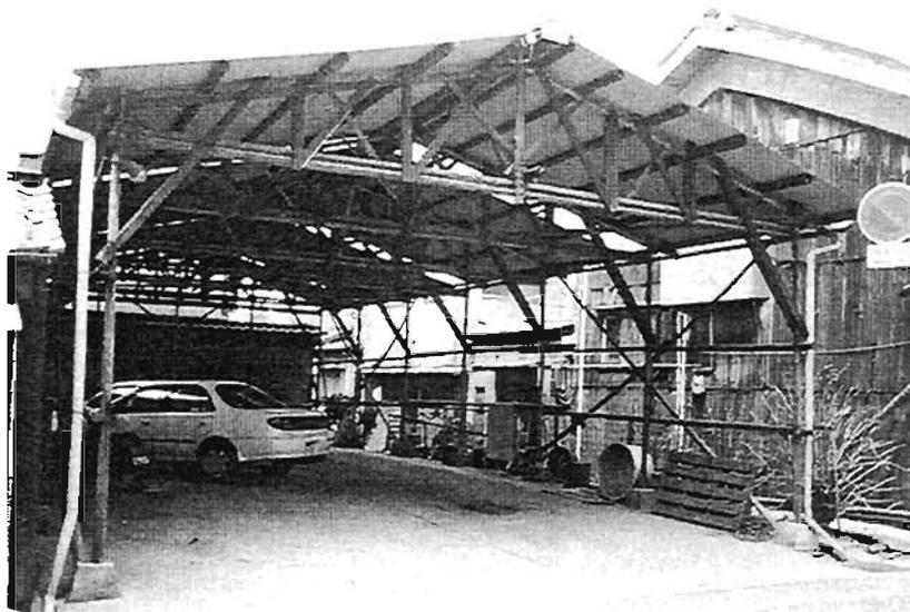
Plate 4.114: Undamaged bamboo portal garage
