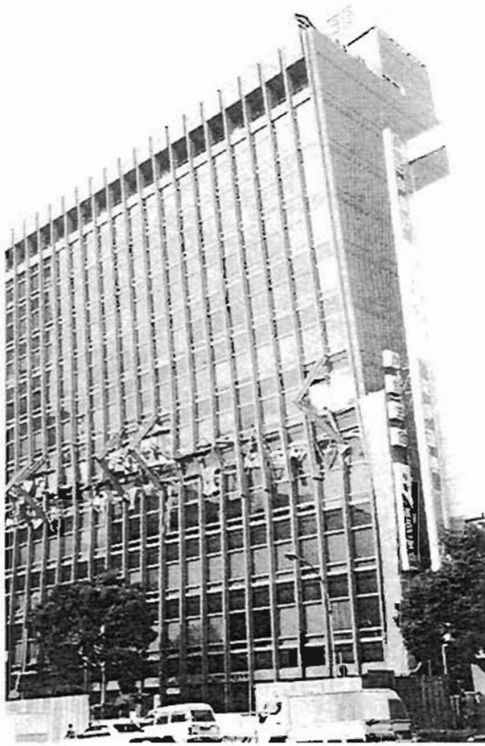
Plate 4.10: Streetwise tilt of 12 storey frame/shear wall structure
