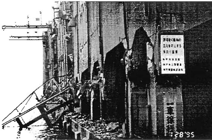
Plate 8.17: Damaged columns of warehouses at the Shinko Pier in Port Kobe
