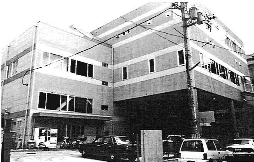
Plate 4.116: Undamaged well designed highly irregular industrial building
