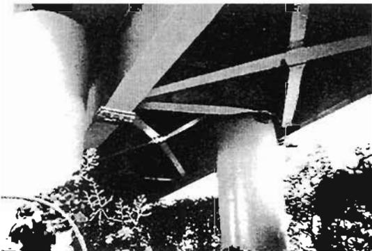
**Plate 6.13** Hanshin Expressway near centre of Kobe: A little higher up same ramp as Plates 6.11 and 6.12, showing girders shifted off column supports and dropped onto deck slab
