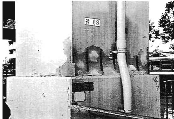
**Plate 6.48** Hanshin Expressway - Damage to Rectangular Steel Pier Column close-up of buckled area of column in Plate 6.47 - internal stiffeners show up as dark lines on exposed orange paint
