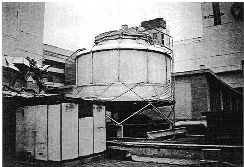
Plate 7.27 Lightly framed Air Handling Unit on roof.
