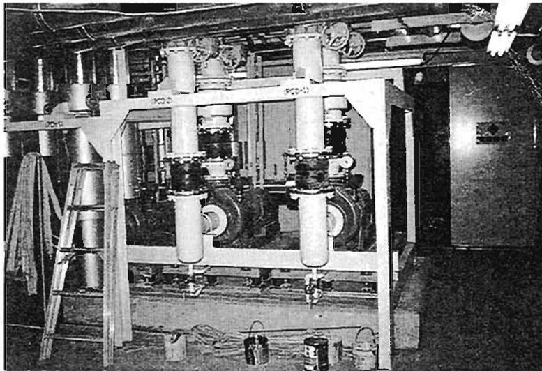
Plate 7.25 Pumps in basement; well anchored
