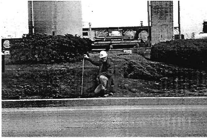
Plate 8.4: Liquefaction settlement observed at a pier of the elevated Portliner railway in Port Island
