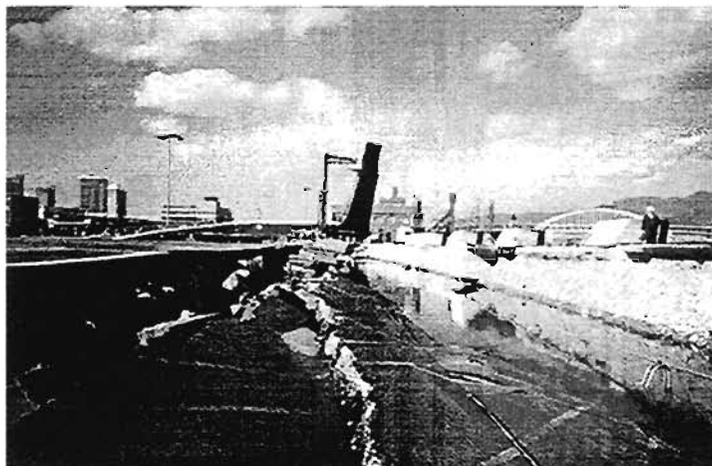
Plate 8.9: Grabens and depressions at the apron slabs behind quay walls
