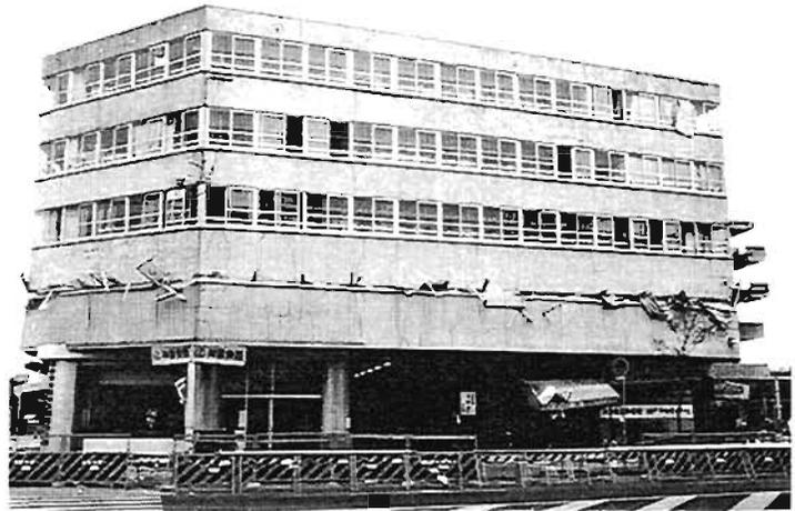
Plate 4.16: 1st Storey collapse due to change in column shape
