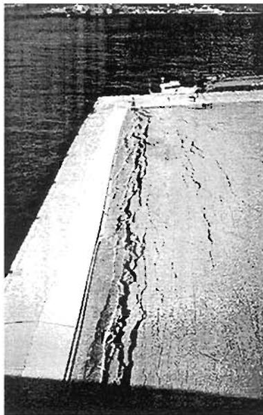
Plate 8.26: Lateral spreading of the ground observed from the Nishinomiya Bridge
