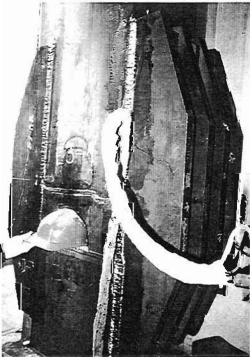
Plate 4.78: Fin strengthening at column fractures
