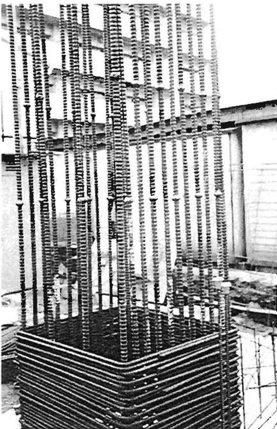
Plate 4.168: Column reinforcement in modern RC construction
