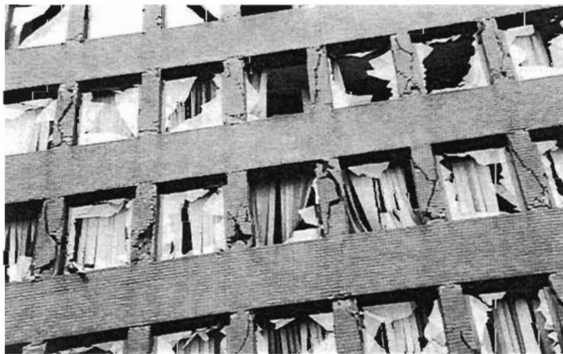
Plate 4.6: Detail of distributed mullion damage in Plate 4.5
