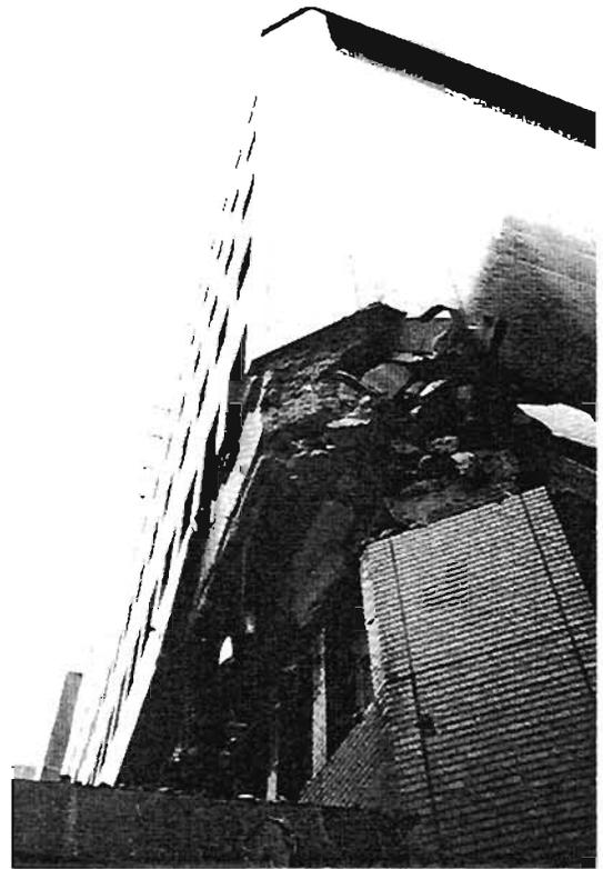
Plate 4.9: Streerwise displacement at adjacent corner
