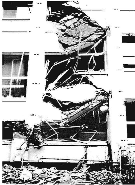
Plate 4.19: Damage where building in 4.18 was torn apart
