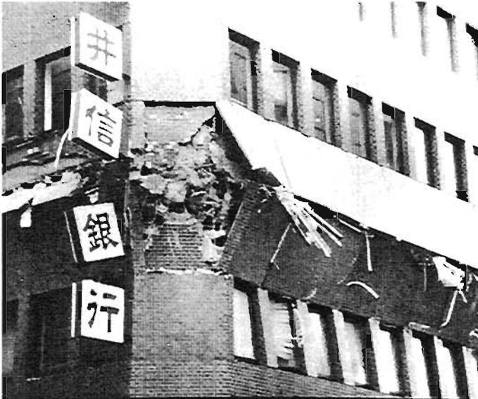
Plate 4.8: Bulging facade at corner where building dropped
