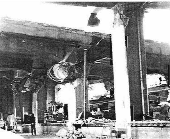
Plate 4.178: Incipient internal transverse hinge
