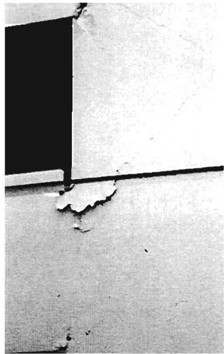
Plate 4.123: Cracking at ends of connecting
