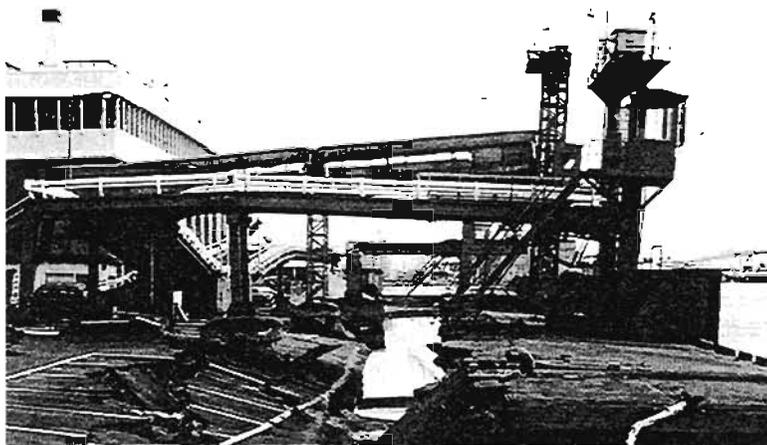
Plate 7.38 Settlement damage to ferry terminal
