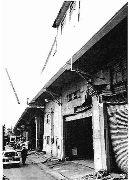
Plate 4.180: Incipient external transverse hinge
