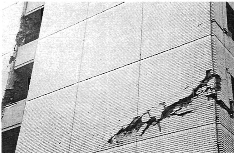
Plate 4.28: Flexural/shear failure in shear wall building
