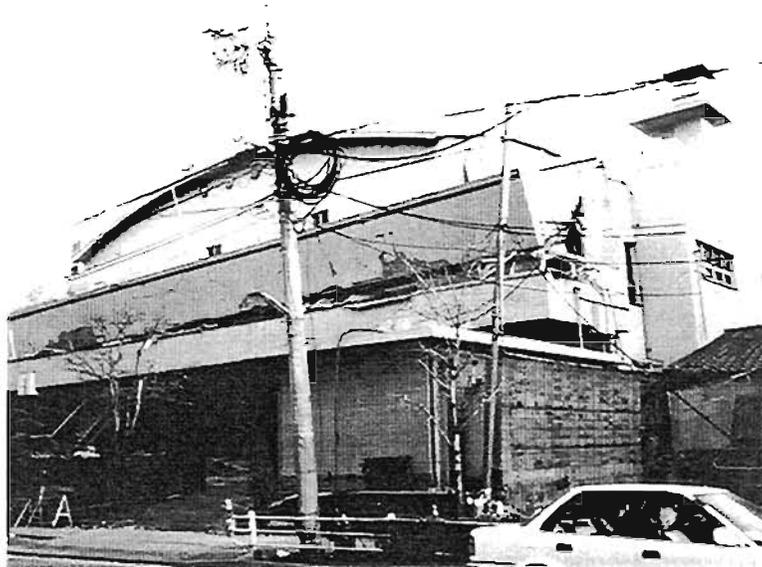
Plate 4.111: Soft storey collapse in domed-roof factory
