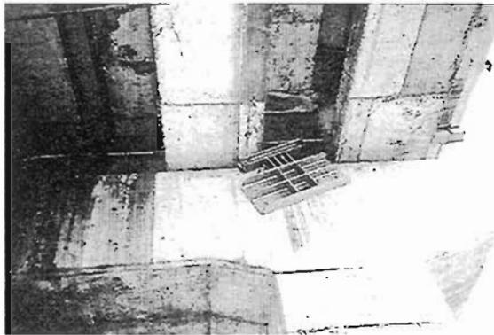
**Plate 6.19** Shinkansen Bullet Train Line, Nishinomiya: Retrofit steel fabrication intended to provide lateral restraint to deck had been twisted out of position.
