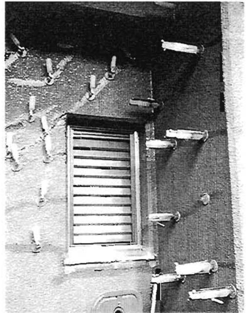
Plate 4.167: Close up of injector and reservoir caps
