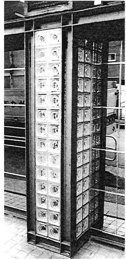
Plate 4.170: Undamaged glass column infill panels in new steel building
