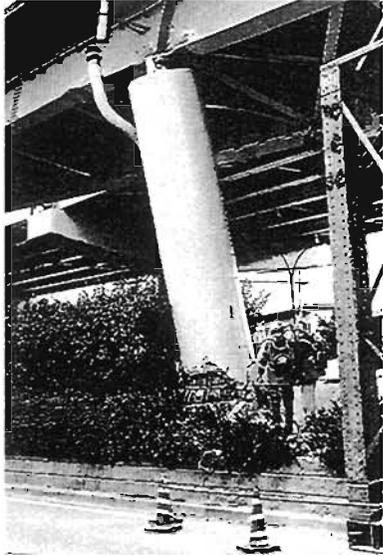
**Plate 6.27** Ramp onto Hanshin Expressway, Kobe: Deck has shifted sideways and taken top of column with it.
