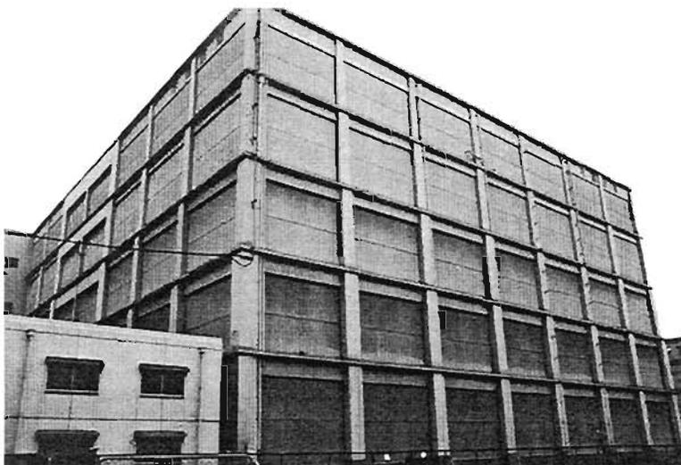
Plate 4.117: Undamaged Japanese framed-wall building
