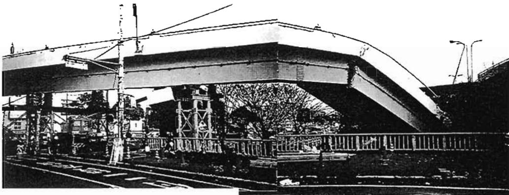
**Plate 6.8** Hanshin Expressway to the west of Kobe centre: Collapse of curved steel box girder ramp due to loss of support at abutment.
