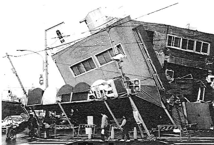
Plate 4.34: Collapsed building with separated shear walls
