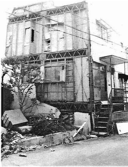
Plate 4.101: Wire bracing in tall panels
