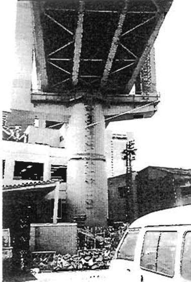
**Plate 6.51** Hanshin Expressway Route 2 near the centre of Kobe- Damage to Circular Steel Pier Column viewed along the line of the structure shows a symmetric buckle at change in wall thickness
