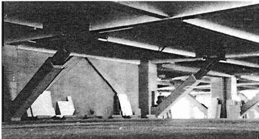
Plate 4.119: Internal bracing
