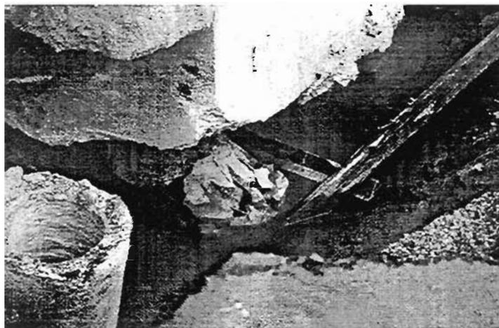
Plate 8.21: Damaged reinforced concrete piles found at Minatojima, Port Island
