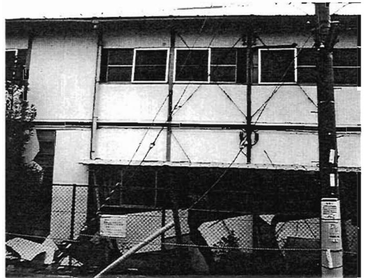
Plate 4.103: Prefabricated building with wire bracing
