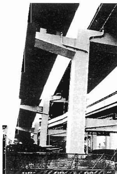
**Plate 6.17** Route 2 near downtown Kobe: Large transverse displacement of deck at movement joint supported on cantilever from portal pier
