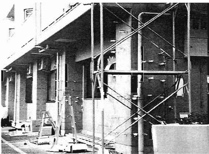
Plate 4.166: Epoxy grouting of columns in lowest floor
