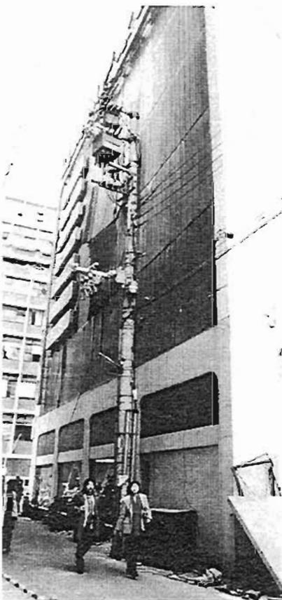
Plate 4.74: Damage to cladding on opposite face
