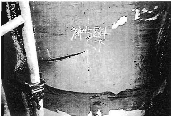
**Plate 6.56** Ramp onto the Hanshin Expressway to the west of Kobe Another view of the tear in the steel wall of the column in Plates 6.55 and 6.56
