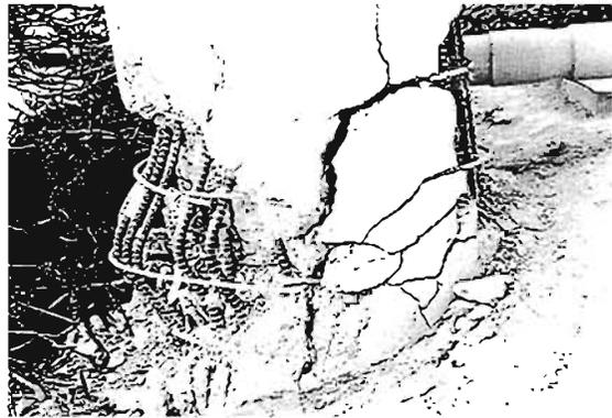
**Plate 6.28** Ramp onto Hanshin Expressway, Kobe: Base of column in Plate 6.27: simple and almost non-existent laps offered no confinement. Failure is at location of curtailment of inner main bars.
