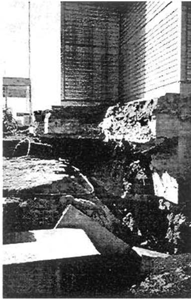
Plate 8.28: Exposed foundation of the KCAT Ferry Terminal building on Port Island
