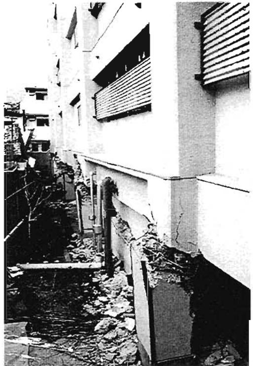
Plate 4.58: Severed shear wall
