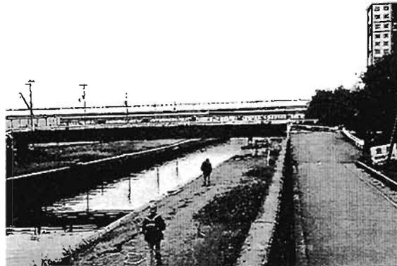
**Plate 6.63** Footbridge over Canal, Kobe lateral spreading caused banks to move inwards, and girder sliced through roadway
