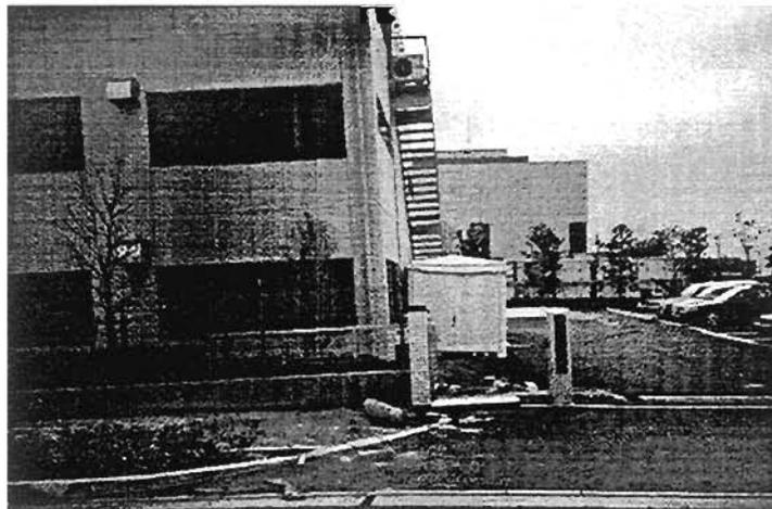
Plate 8.29: Tilting of a three story office building affected by lateral spreads
