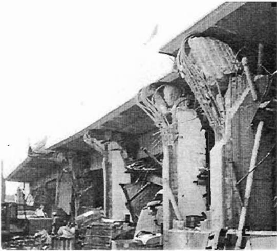
Plate 4.176: Differential drifts between transverse joints
