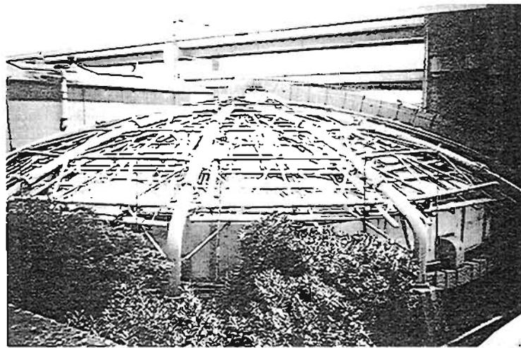
Plate 7.14 Glassfibre panel roof, with temporary supports
