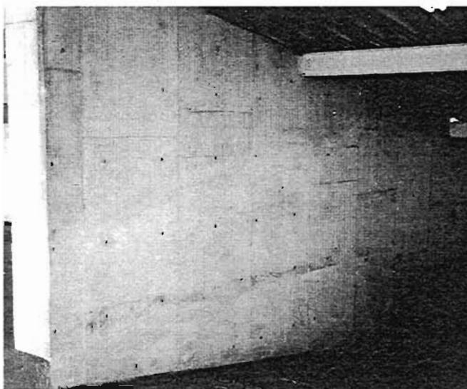
Plate 4.128: Repaired cracks in transverse wall
