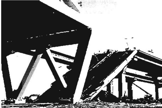
**Plate 6.5** Nishinomiya Harbour Bridge on the Hanshin Bay Expressway Approach span fell due to loss of support as main pier shifted towards main span.
