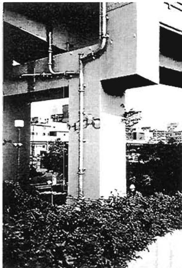
**Plate 6.53** Hanshin Expressway Route 2 near the centre of Kobe- Damage to Rectangular Steel Pier Column change in wall thickness is likely to explain location of buckle in this stiffened box column
