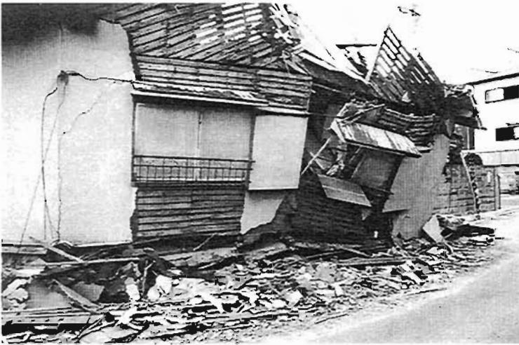
Plate 4.96: Collapsed timber-framed houses
