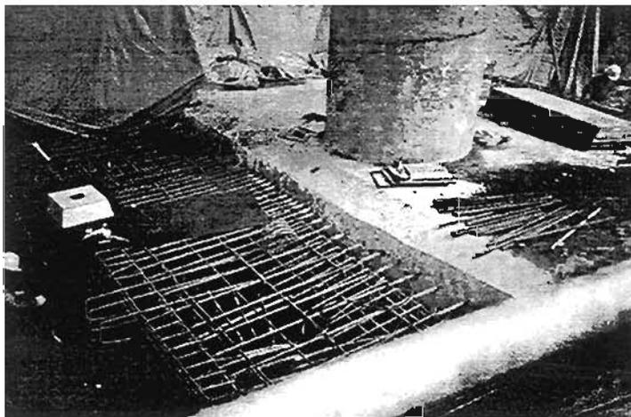
Plate 8.24: Repair works of a pile foundation of the elevated Portliner Railway in Kobe
