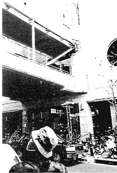
**Plate 6.66** Footbridge Linking Buildings in Kobe Out of phase movements caused buckling of tubular steel members
