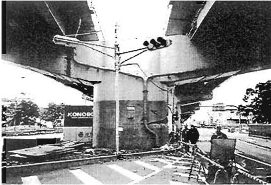
**Plate 6.31** Hanshin Expressway, Kobe: Damage to large pier at level of construction joint and/or curtailment of reinforcement.
