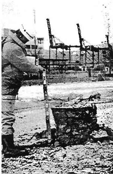
Plate 8.5 : A pile remained in place and the surrounding ground liquefied and settled.
