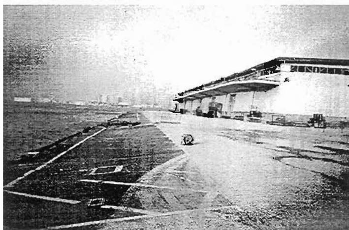
Plate 8.15: Temporary backfilling works of damaged concrete caisson walls on Port Island
