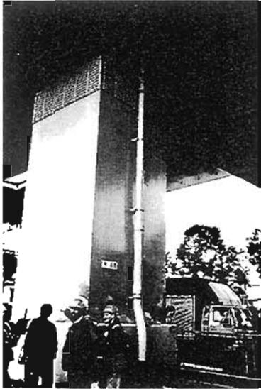
**Plate 6.47** Hanshin Expressway - Damage to Rectangular Steel Pier Column stiffened walls buckled exposing orange coloured primer/undercoat
