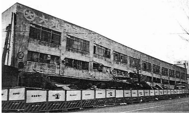
Plate 4.108: Progressive collapse in older 11 bay three storey building
