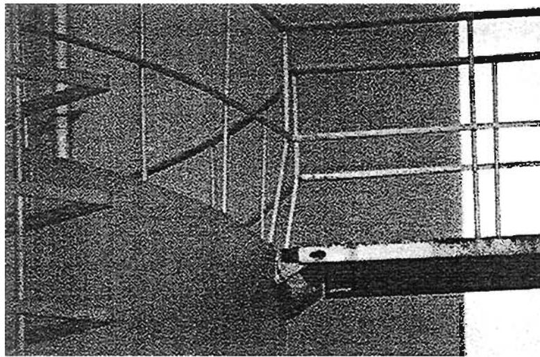
Plate 7.17 Effect of lack of movement joint
