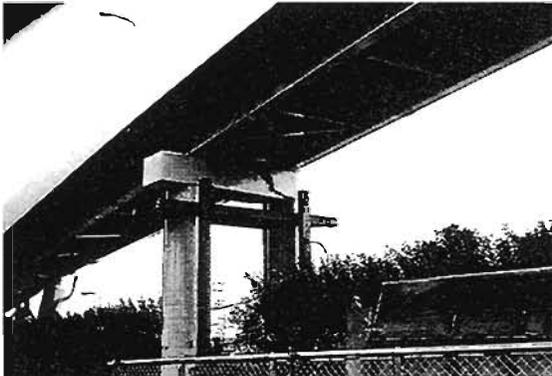
**Plate 6.29** Ramp onto Hanshin Expressway, Kobe: Sideways shift of deck and brittle fracture of portal frame crosshead beam
