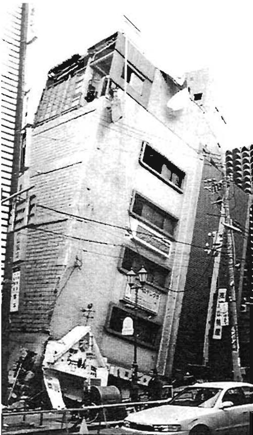
Plate 4.31: Rigid body rotation in one-sided collapse
