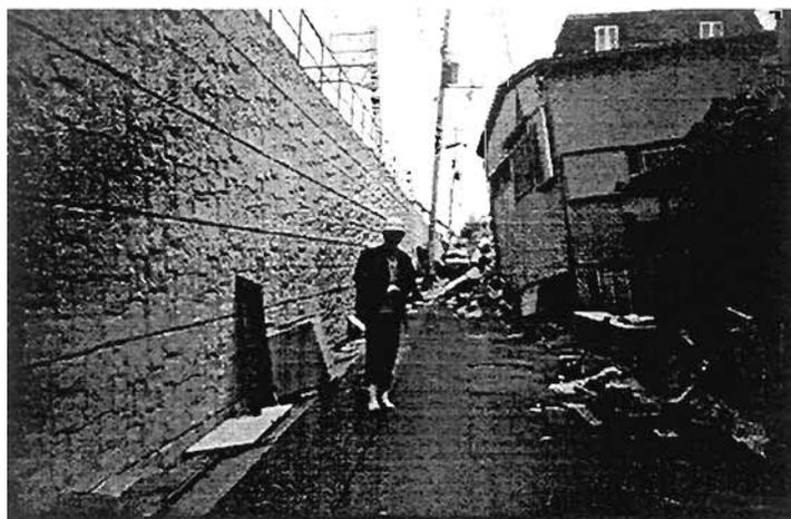
Plate 8.36: Good performance of a reinforced geotextile wall at Tanata
