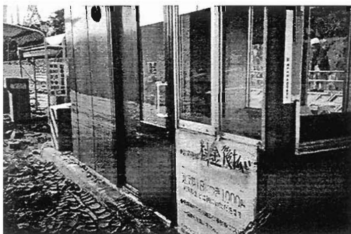
Plate 8.14: A dried water splash marker of liquefied soils found at the toll gate box on Port Island
