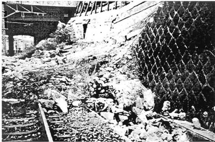
Plate 8.35: Collapse of a masonry stone retaining wall (photo by Prof. J. Koseki)
