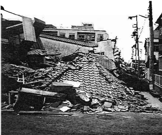
Plate 4.99: Collapse with roof intact
