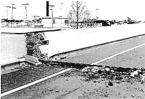
**Plate 6.23** Ramp onto Hanshin Expressway near centre of Kobe: Hammering at joint has damaged deck joint and parapets
