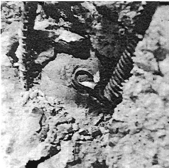
Plate 4.38: Live electrical duct in shear wall
