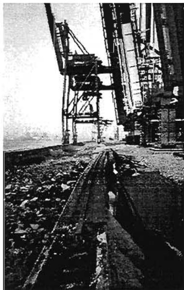
Plate 8.12: Displaced rail tracks by the movement of cranes observed on Port Island
