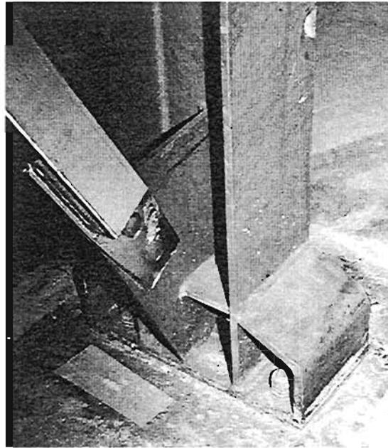
Plate 4.136: Column base/brace connection
