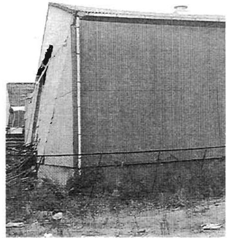
Plate 4.113: Mid-side failure of long steel frame shed
