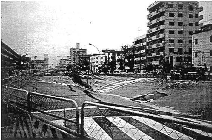
Plate 8.33: Collapse of the Daikai Station
