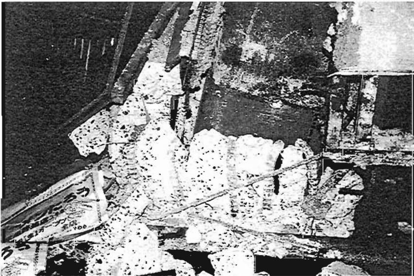
Plate 4.93: Column pulled out of plinth
