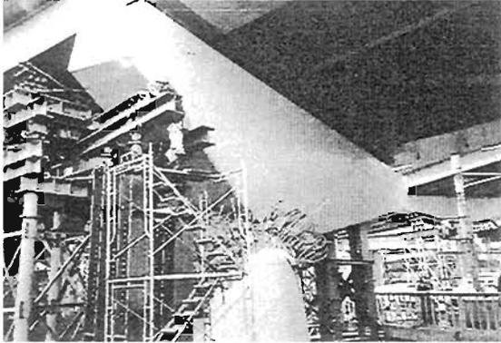
**Plate 6.35** Hanshin Expressway to the west of Kobe centre: Shear-flexure failure at underside of column crosshead - lack of confinement
