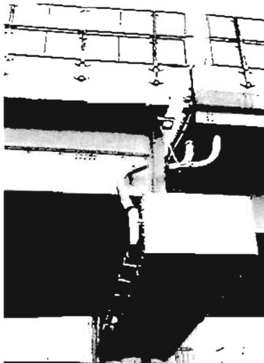
**Plate 6.21** Hanshin Expressway to the east of Kobe: Longitudinal shift of deck has sheared bearing bolts and dislocated drainage
