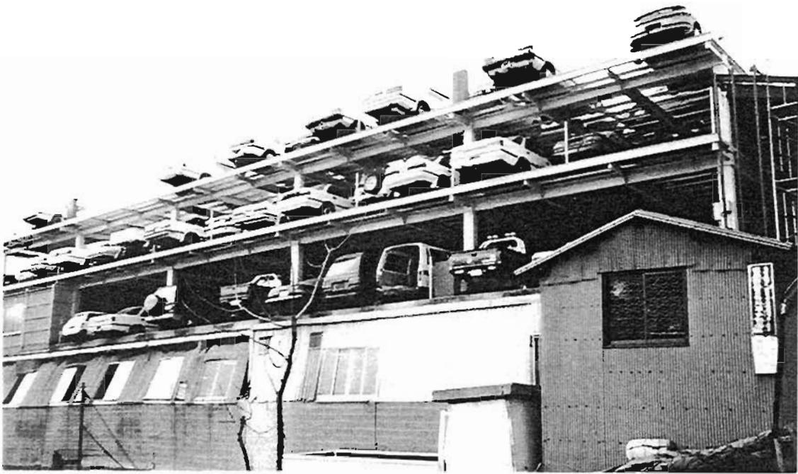
Plate 4.138: Flexible steel car park in port area above damaged ground floor office
