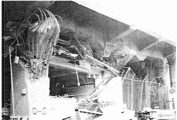
Plate 4.177: Incipient longitudinal hinge and more developed transverse hinges
