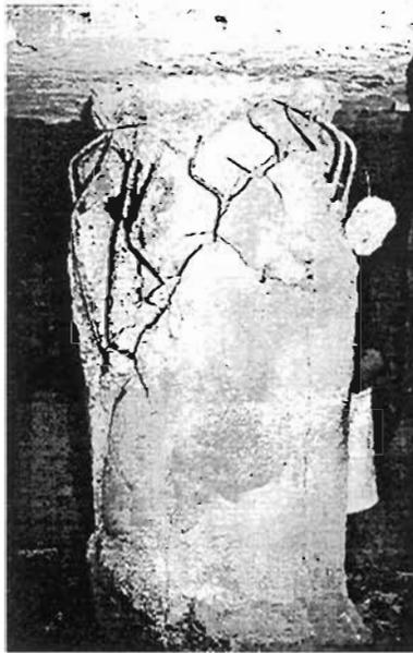
Plate 8.20: Damaged pile foundation due to soil liquefaction (photo by Prof. K. Tokimatsu)
