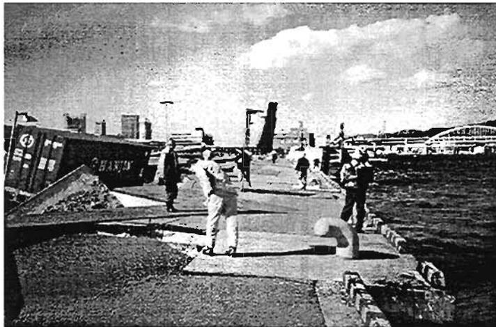
Plate 8.8: Lateral movement of concrete caisson walls in Rokko Island
