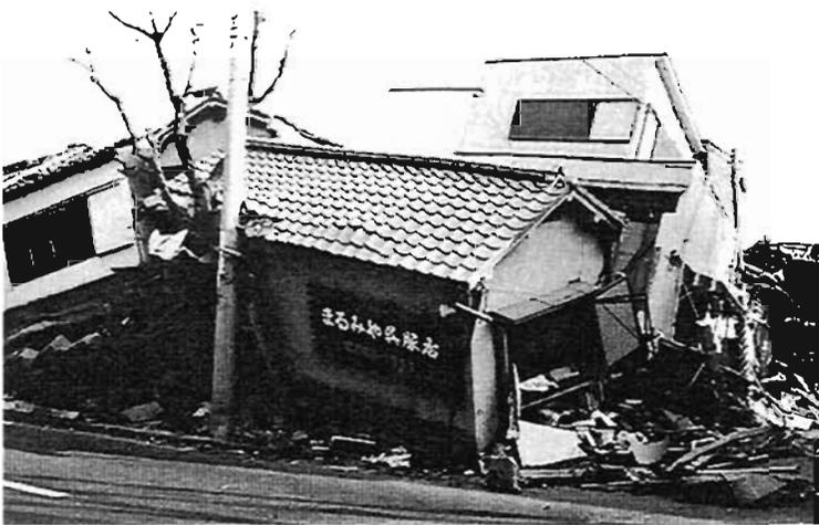
Plate 4.97: Collapsing house stabilised by pole
