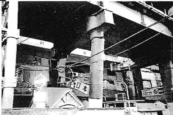
**Plate 6.57** Railway near Centre of Kobe - Damage to Steel Portal Pier centrifugally cast columns lacked ductility
