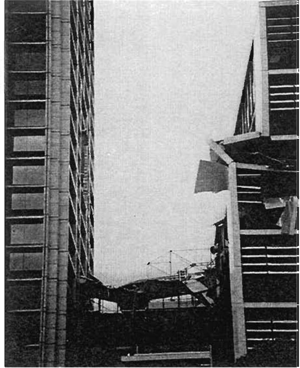
Plate 4.88: Collapsed and surviving link bridges
