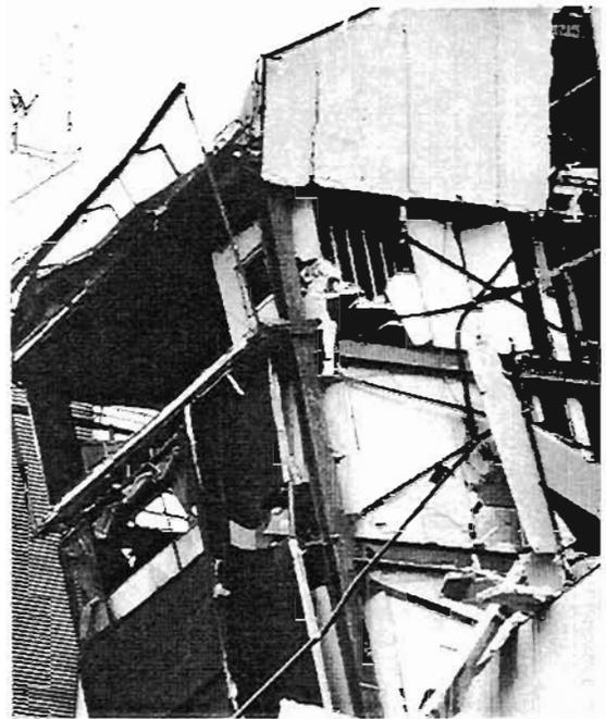
Plate 4.69: Snapped bracing
