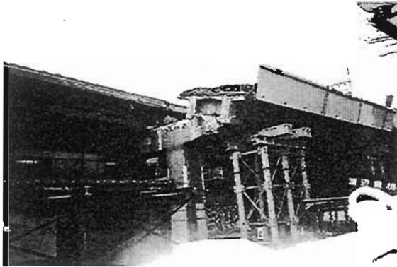
**Plate 6.15** Train Line in Kobe: Narrow twin I-girder carrying one track almost fell off portal pier transversely - the missing one probably did fall off sideways.
