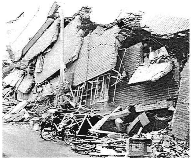
Plate 4.33: Totally collapsed perforated shear wall building
