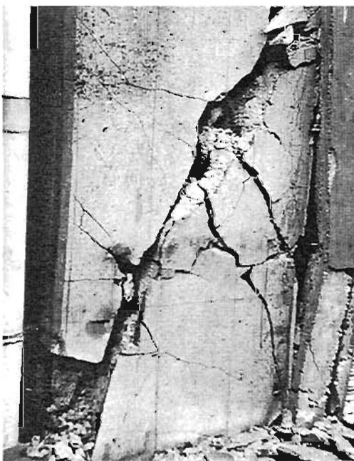
Plate 4.183: Incipient shear failure
