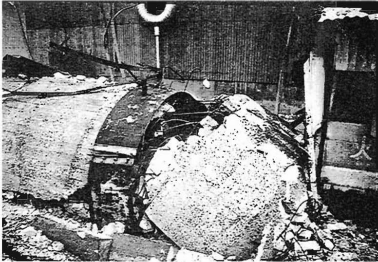
Plate 7.34 Fallen section of RC stack
