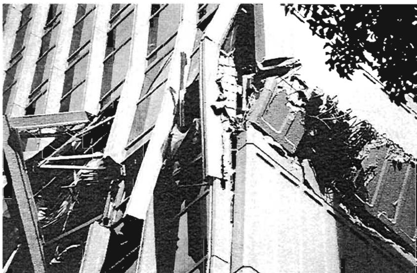
Plate 4.12: Collapsed part of side shear wall
