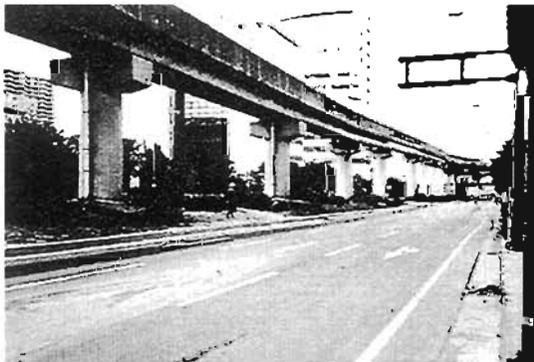
**Plate 6.60** Automatic rail line linking the JR Line and Port Island softening and settlement of ground left blocks of soil above pilecaps projecting above median
