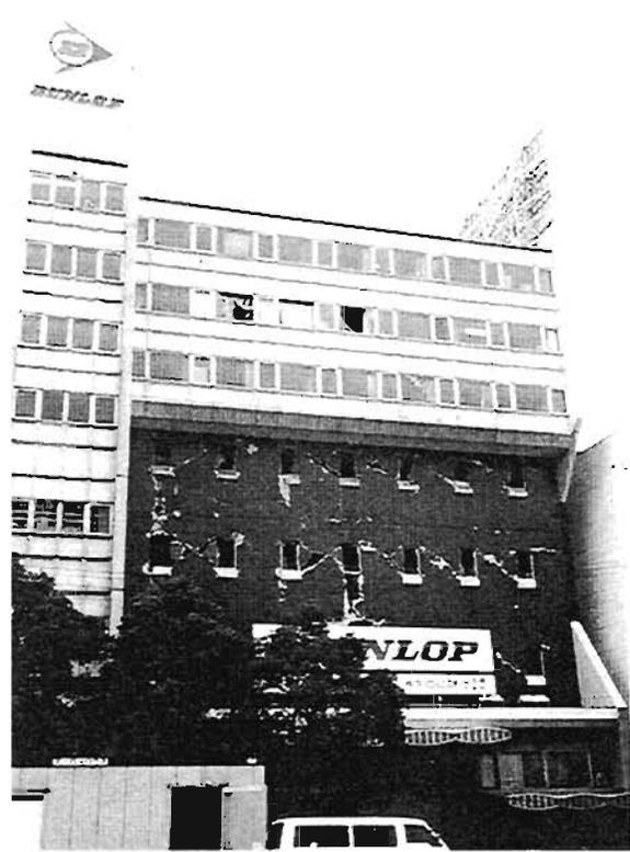
Plate 4.30: Distributed inelasticity in shear wall structure
