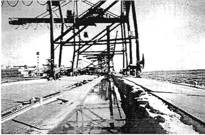
Plate 8.10: Cranes in Rokko Island were pulled apart by the lateral movement of concrete caisson walls
