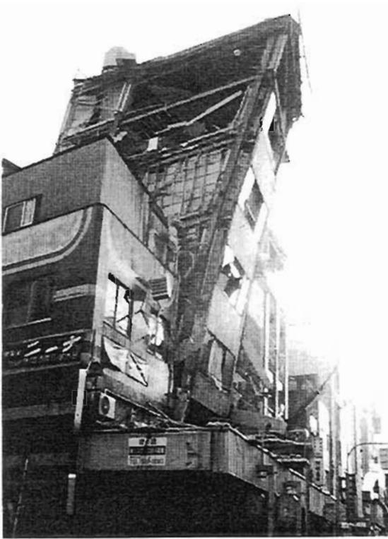
Plate 4.68: Sway after snapping of bracing flats in upper stories
