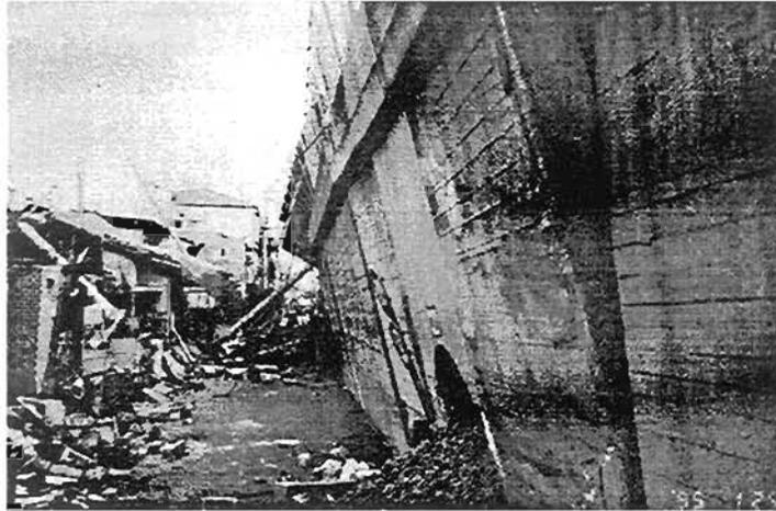
Plate 8.34: Tilt of a concrete gravity retaining wall (photo by Prof. J. Koseki)
