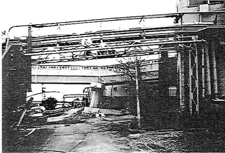
Plate 7.19 Pipebridge damaged by lateral ground spreading
