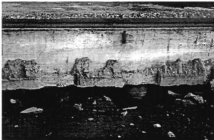
Plate 8.11: Exposed piles under the concrete block foundation of the cranes in Port Island
