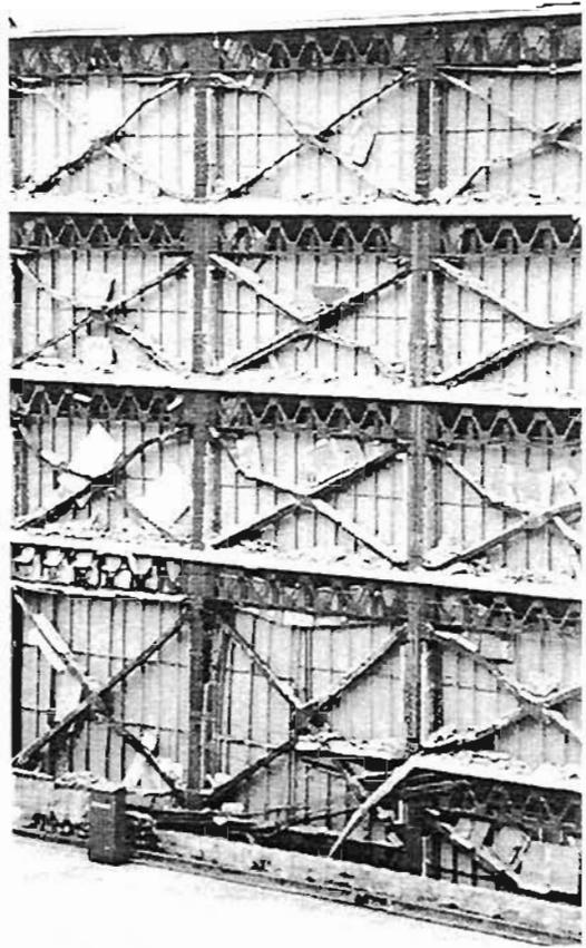
Plate 4.73: In-plane buckling of bracing
