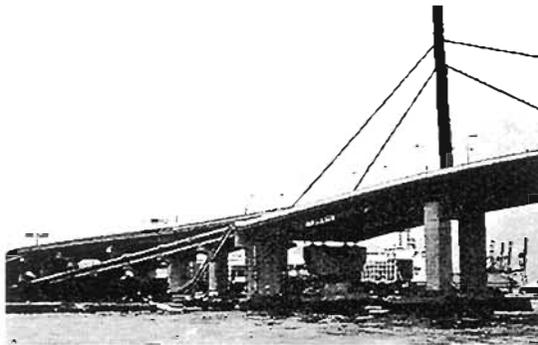
**Plate 6.45** Cable-stayed Bridge alongside the Maya Ohashi Bridge structure was undamaged apart from some minor damage at the top of pedestrian access stair
