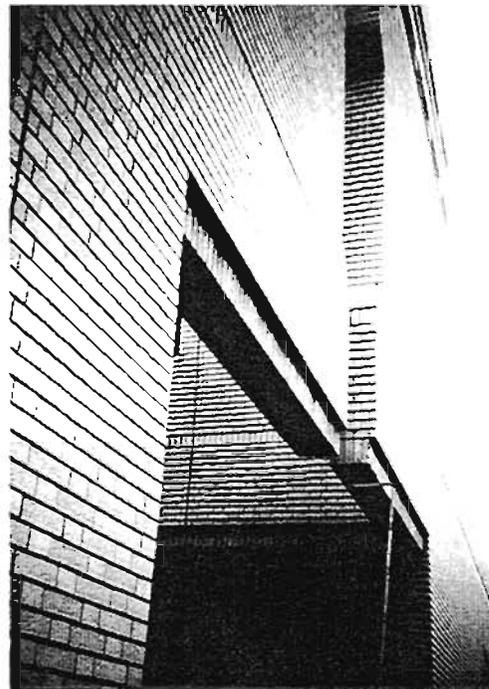
Plate 4.26: Relative displacement between buildings
