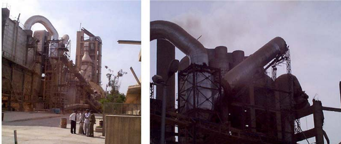
Figures 60 & 61 Sikka Cement Works
