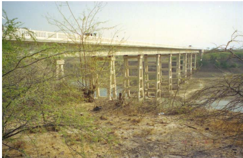
Figure 1 Rudramata (Khari) Bridge – view from north side
