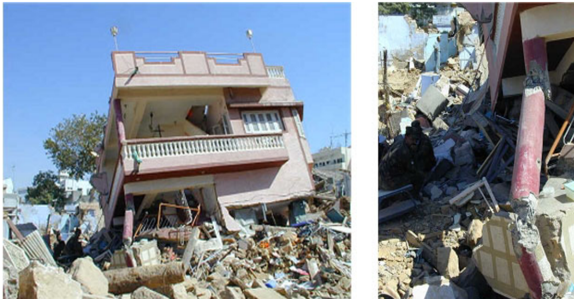
Figure 18 Building Collapse in Bhuj
