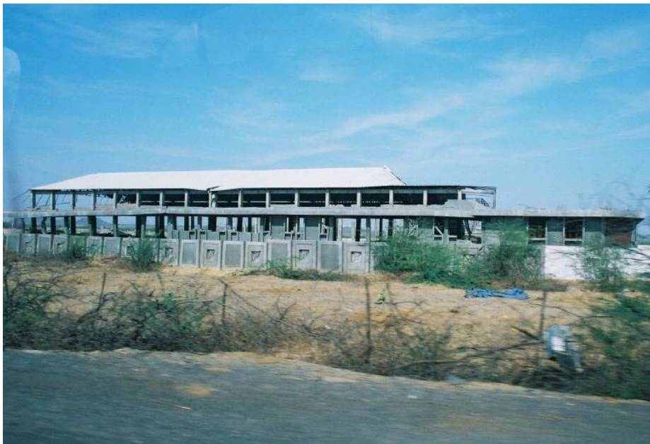
Figure 59 Factory Unit Near Bachau
