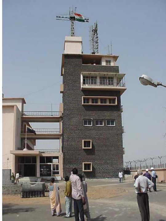
Figure 50 Kandla Port: 6-storey control tower building was inclined by a few degrees towards the water.
