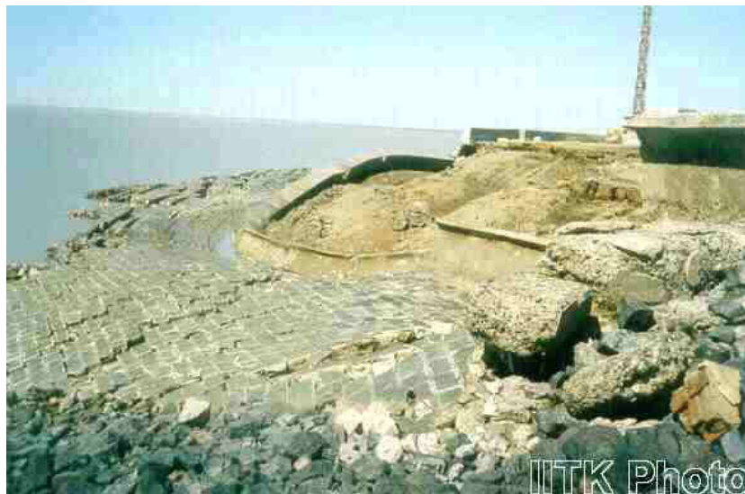
Figure 32 Lateral spreading resulting in damage to sea revetments [courtesy of IIT Kanpur]
