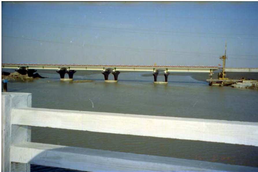
Figure 26 Surajbari New Bridge: 39 spans of 32.2m, prestressed beams on twin leaf r.c. piers and well caisson foundations
