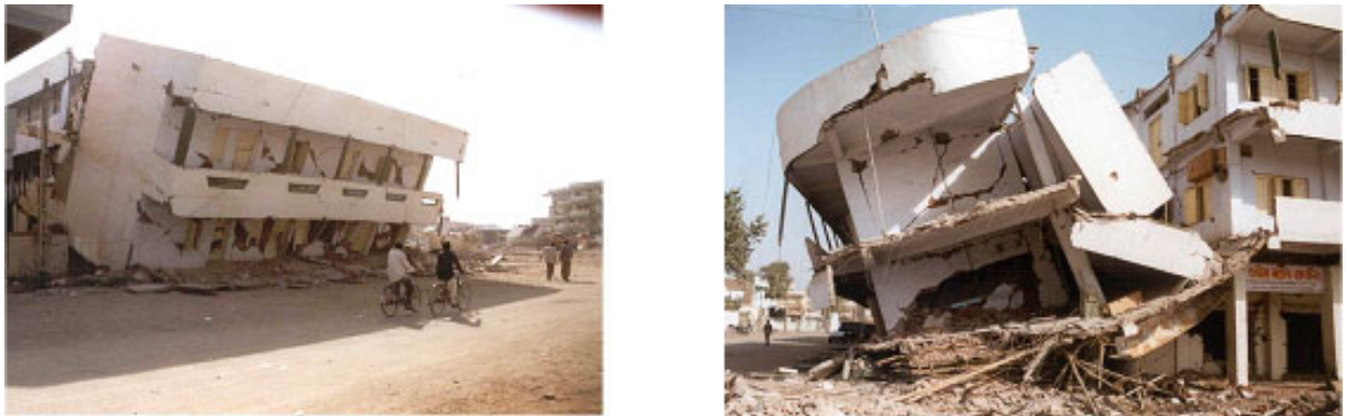
Figure 4 Soft storey failure in Gandhidham
