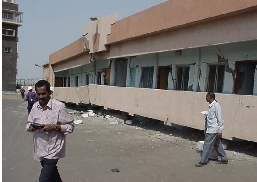
Figure 48 Kandla Port: 2-storey building parallel to the waterfront had lost its lower storey due to soft-storey collapse of the circular columns
