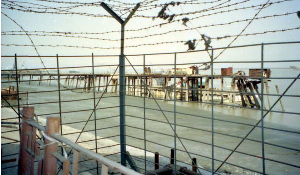
Figure 47 Kandla Port: jetty for small craft to north of the control tower had been badly damaged by the cyclone and then the earthquake. Reinforcement corrosion had already weakened the structure.
