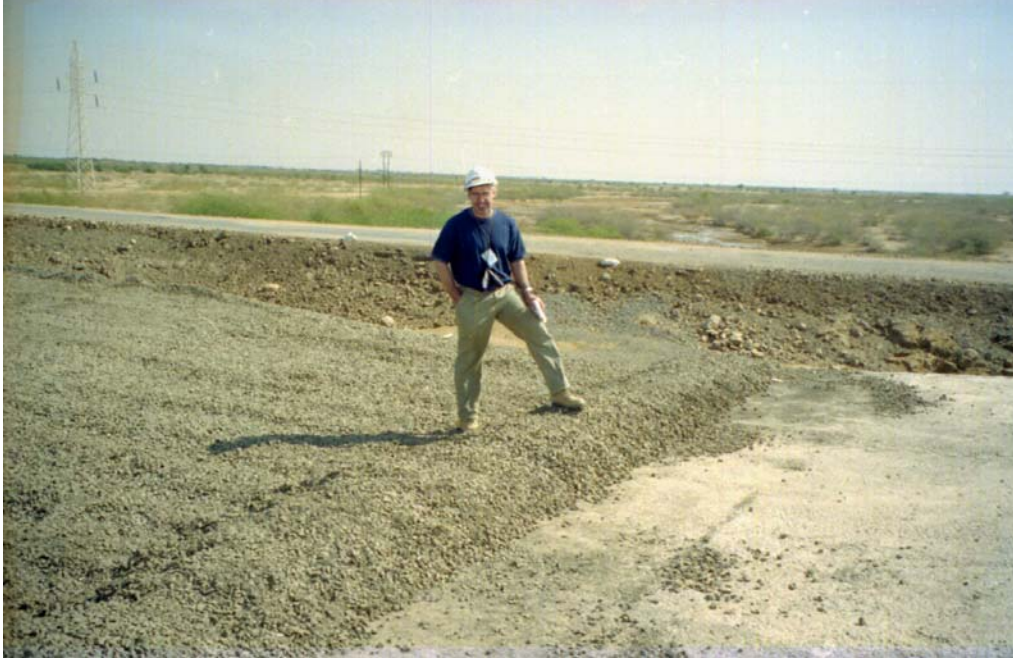
Figure 15 Four-Bridges Site on NH8A, new road bridge: hump of subgrade material at end of approach slab
