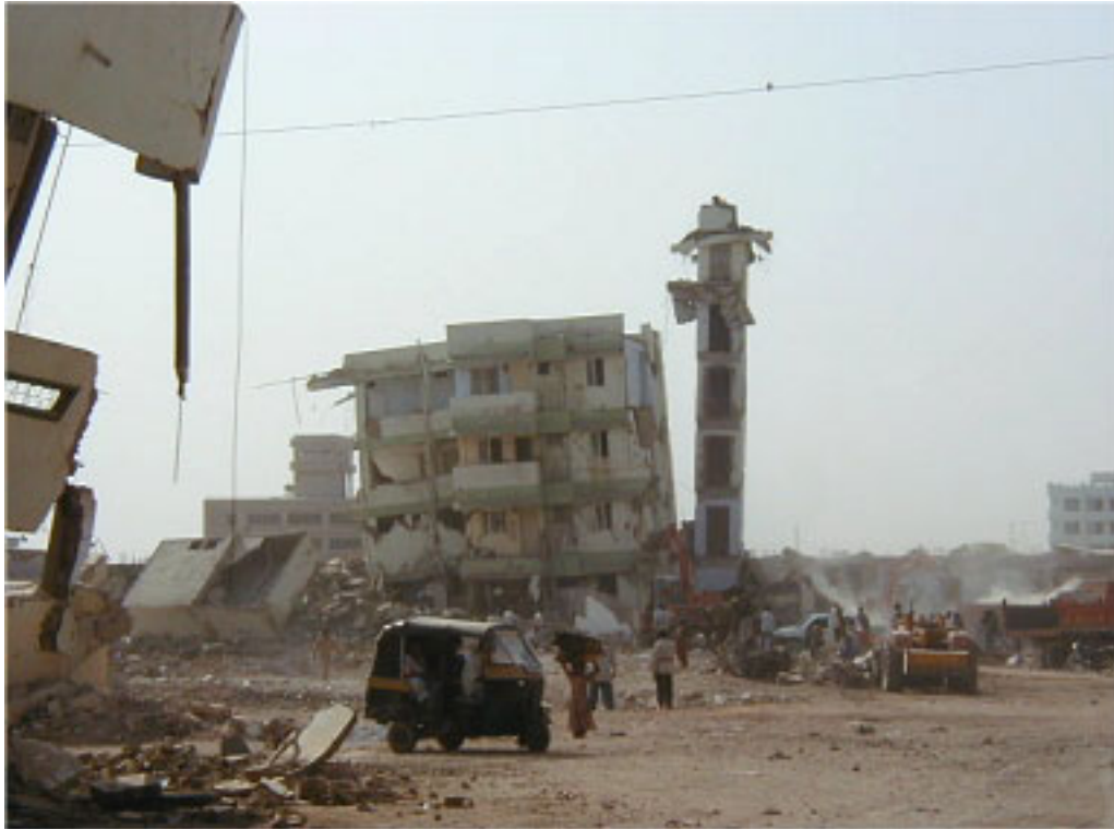
Figure 12 Combination of collapses in Gandhidham
