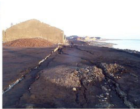
Figure 34 Severe cracking and lateral spreading of the area adjacent to the jetties
