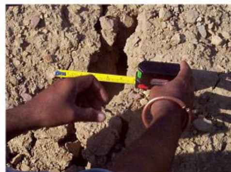
Figure 40 The largest cracks were over 50 mm wide and extended to the core
