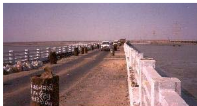
Figure 25 Surajbari Old Bridge: deck displaced vertically and horizontally, horizontal displacement was a maximum of about 1.5m at Pier P15. [Photo courtesy of Mahesh Tandon].
