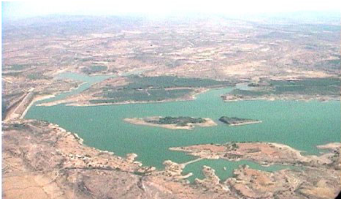
Figure 38 Aerial view of the Rudra Matha dam [courtesy of EERI]
