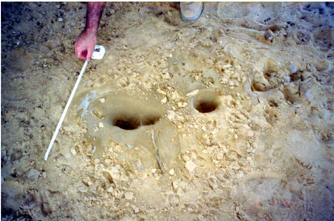
Figure 6 Six Span Bridge near Dudhai – signs of liquefaction in the dry river bed
