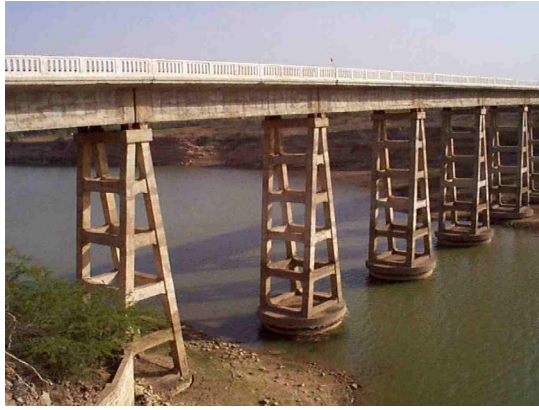
Figure 9 Overview of the Rudra Matha bridge
