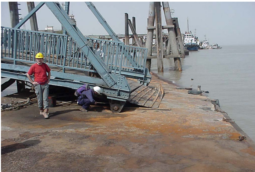
Figure 44 Kandla Port, launch jetty: link span had jumped from its guides and punched into the adjacent deck plates
