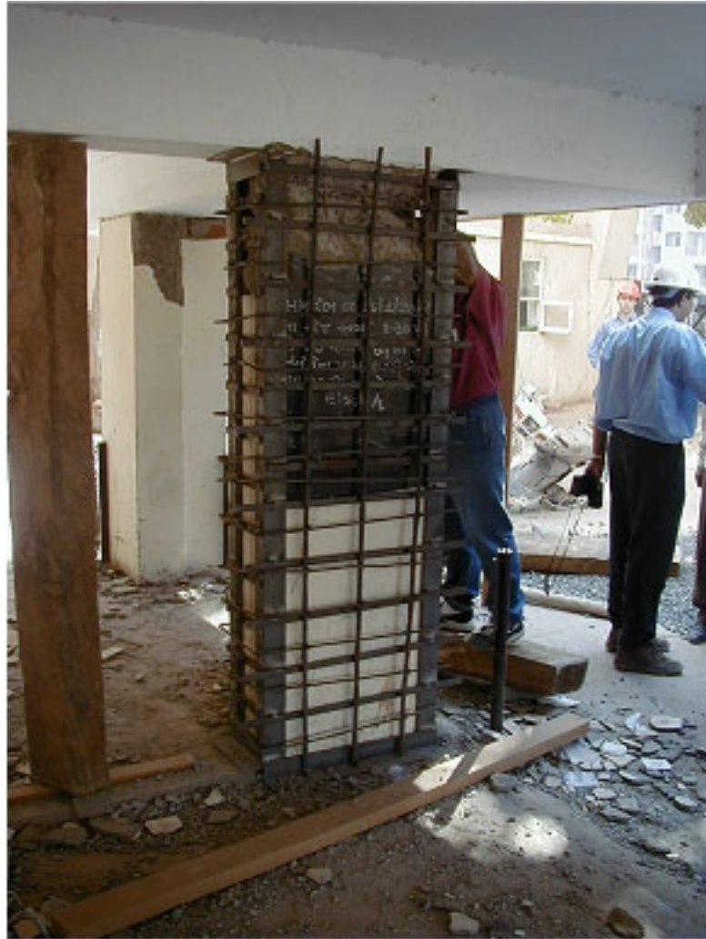
Figure 19 Column repair in Ahmedabad
