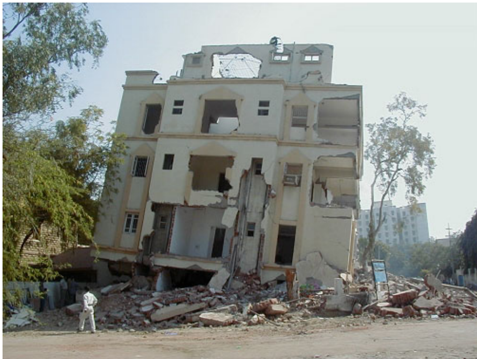
Figure 4 Typical RC framed Type C2 building in Ahmedabad where ground floor columns have failed in a weak storey mechanism. Note the absence of columns along the perimeter of the building.
