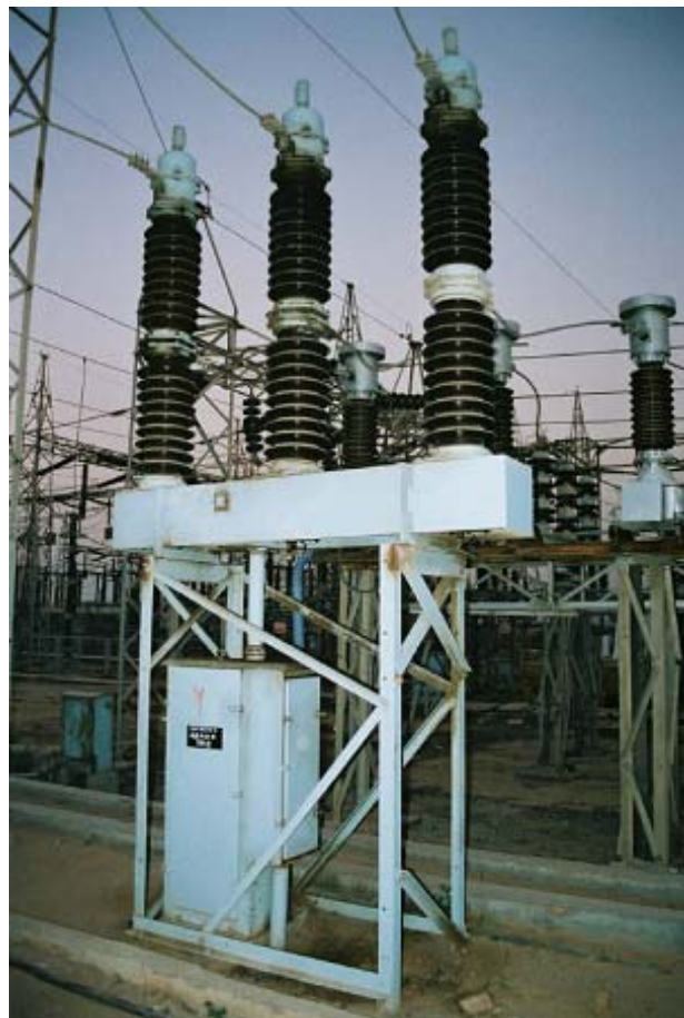
Figure 63 Repaired Circuit Breaker at Anjar Substation
