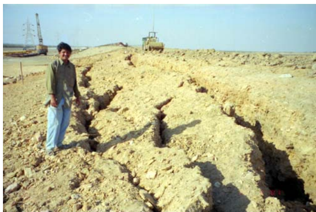
Figure 31 Surajbari New Bridge: liquefaction of the underlying soil caused settlement and cracks in the approach embankments
