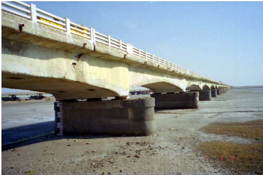
Figure 22 Surajbari Old Bridge: 37 spans of 32.2m, reinforced concrete box girder supported on r.c. piers and well caissons
