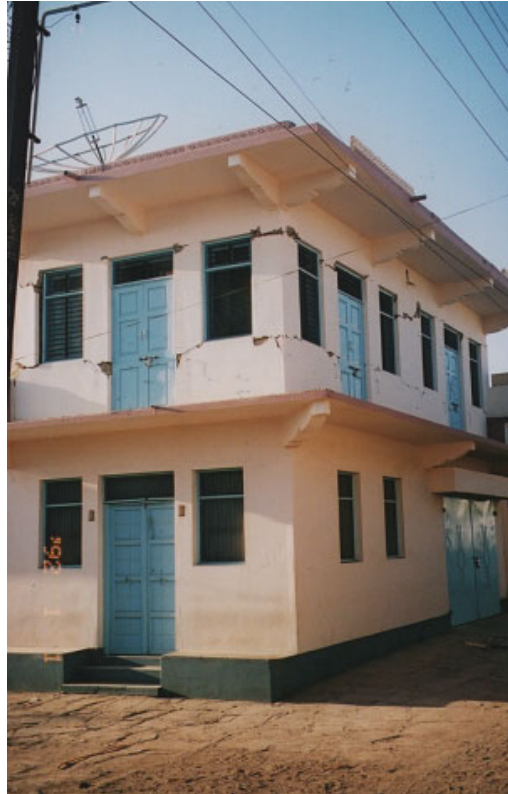
Figure 3 Typical coursed stone with concrete diaphragms Type C1 building suffering moderate damage in the masonry piers.
