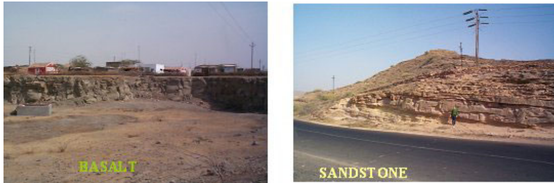
Figure 2 Excavation and highway cuttings confirm the presence of Igneous Basalt and Sandstone formations in Kachchh
