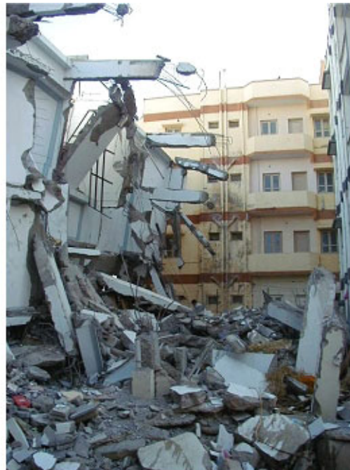
Figure 11 Overturned building in Bhuj
