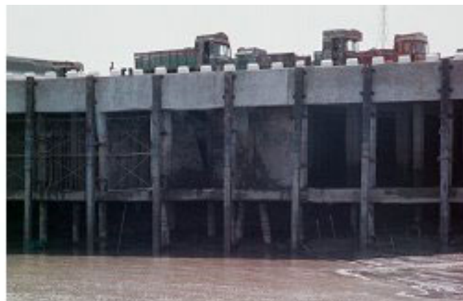
Figure 22 A view of the old jetties at Kandla Port
