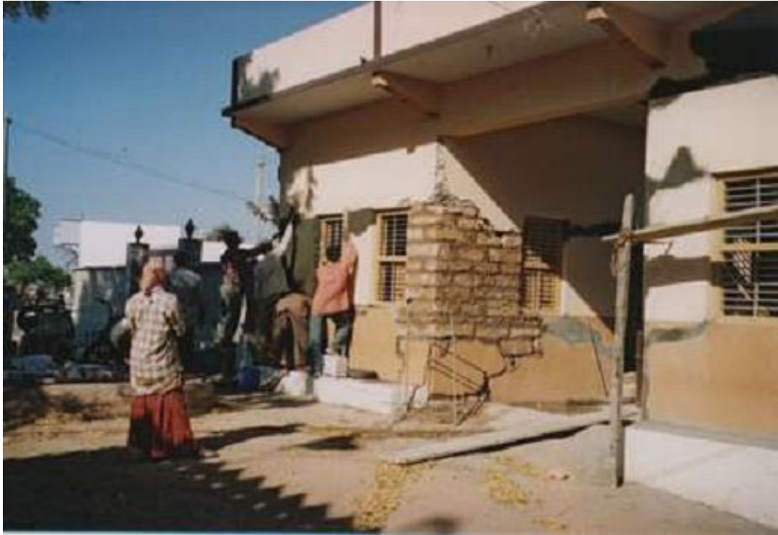
Figure 9: Making good of damaged masonry corner.
