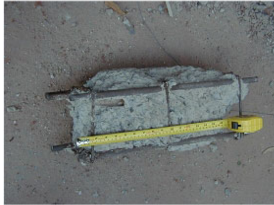
Figure 14 Burst concrete cover
