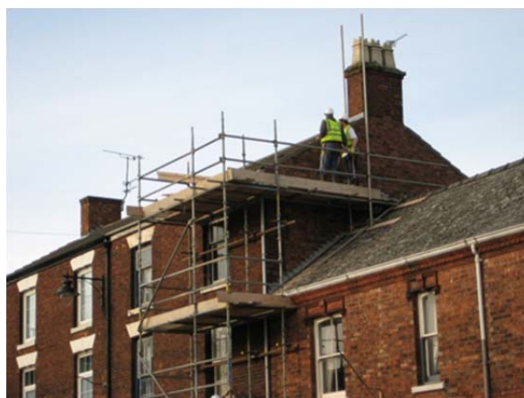
Figure 5: Roof and chimney repairs being undertaken two days after the event.
