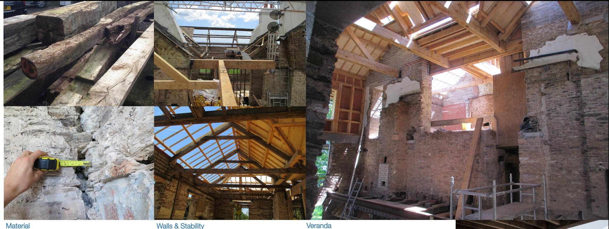
The new structure is mostly timber with a few visible reinforced concrete elements. Large exposed oak beams and posts with traditional joints are used to support the floors, walls and roofs. The use of long span oak beams has meant that limiting long term creep deflection and moisture movement has been a key design consideration. Specification of well-seasoned oak, together with limits on the strength grade, moisture content and growth ring orientation has been critical.
