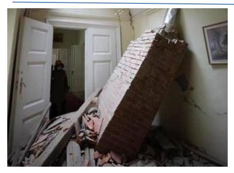
Figure 5-1 Damage of chimney falling indoor Source: City of Zagreb
