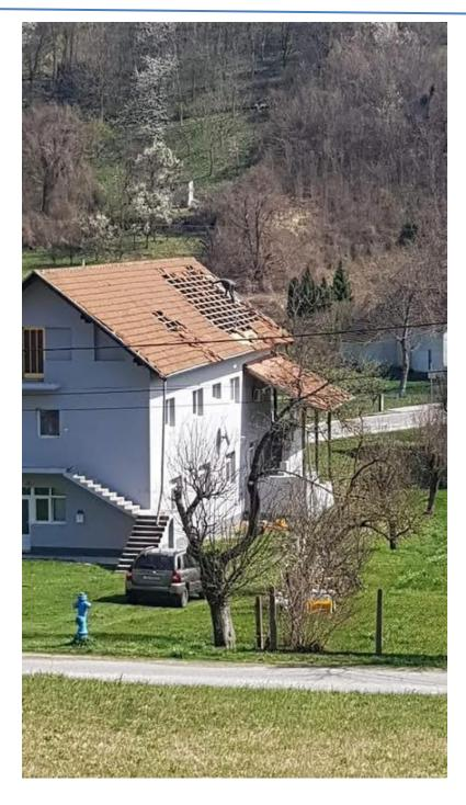
Figure 5-14 – Roof damage, credits to Dolores Rogic
