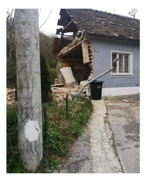
Figure 5-13 – Collapse of the whole facade – credits to Dolores Rogic
