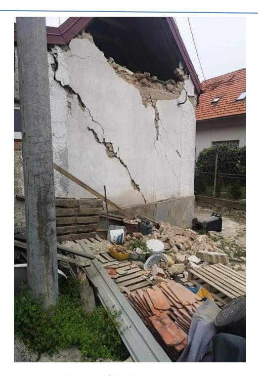
Figure 5-15 - Gable failure, credits to Dolores Rogic
