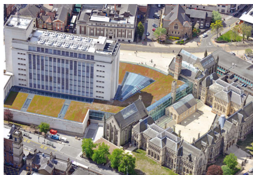
↓ FIGURE 9: Transformation of existing buildings at Nottingham Trent University
