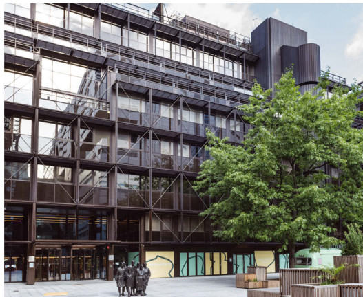
FIGURE 4: 1 Finsbury Avenue, London
