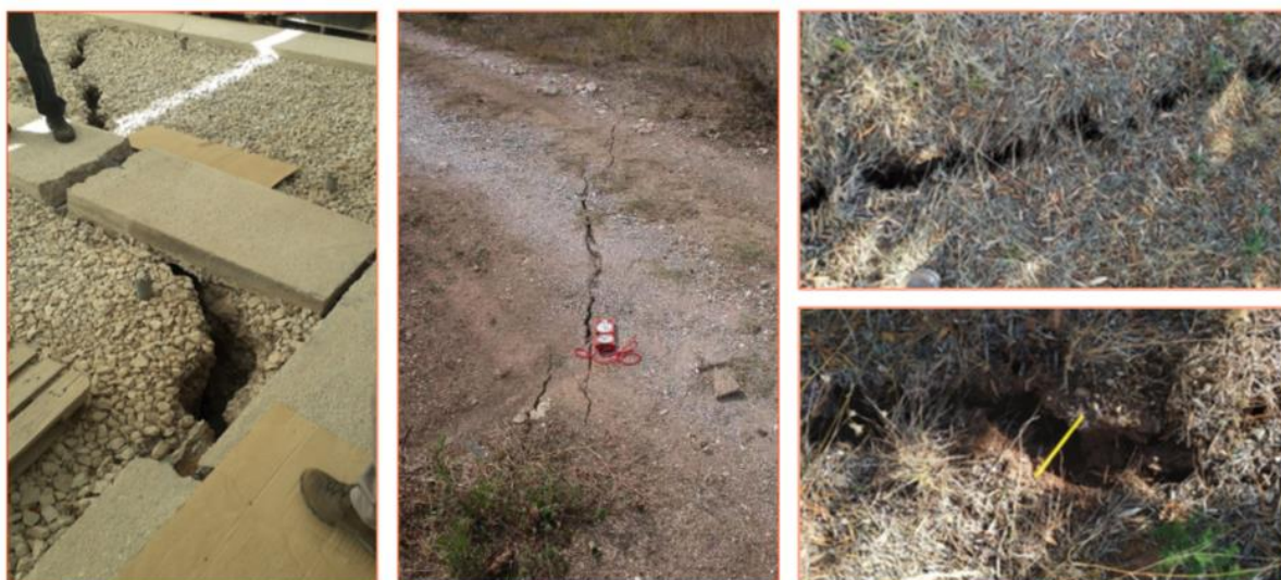
Figure 11: Photographs from Lekkas et al. (2020) illustrating surface rupturing in the Agios Nikolaos area in NW Samos.
