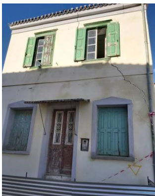
Figure 66: Diagonal shear cracks to the walls with different widths.
