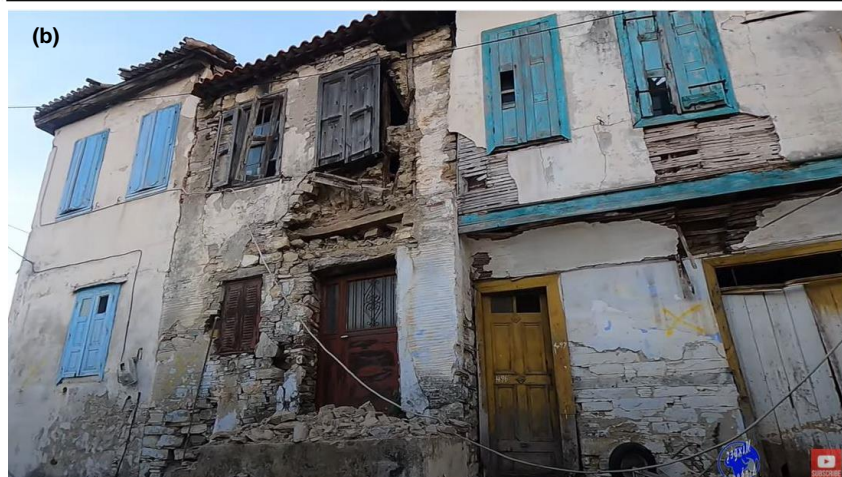
Figure 92: (a) Schematic representation of a timber frame (after Diri, 2010) and (b) two buildings with stone infill (the building in the middle) and bağdadi cladding (the building on the right) (from "Mikres diadromes" youtube channel)
