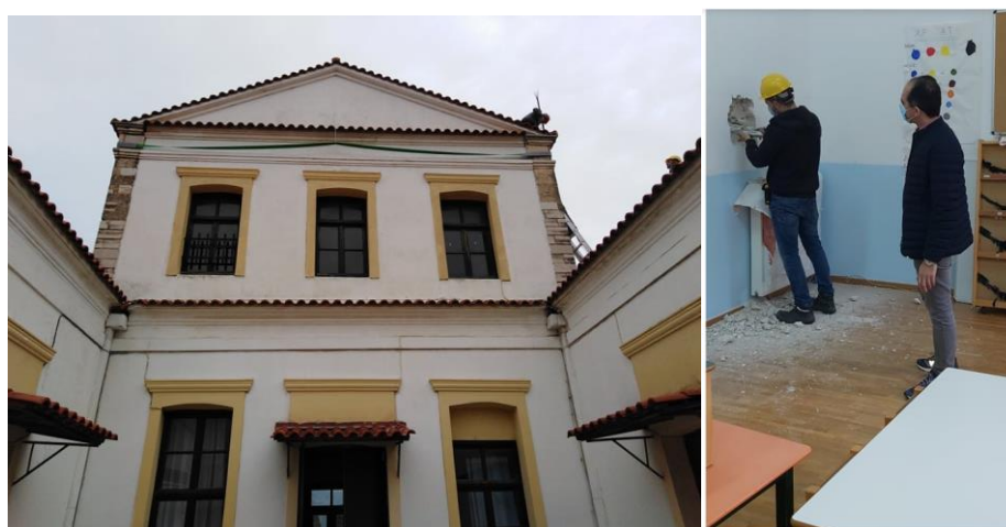
Figure 123: Primary school of Mitilinioi, confinement of the walls with external straps (left); repair works at Agios Konstantinos Primary School, so that their function can be resumed (Municipality of Eastern Samos Facebook page, 16.01.20)
