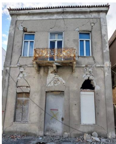
Figure 67: (a) In plane cracks to spandrels and piers, (b) out of plane wall failure
