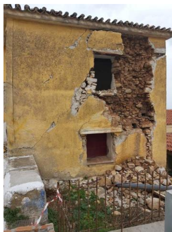
Figure 67: (a) In plane cracks to spandrels and piers, (b) out of plane wall failure
