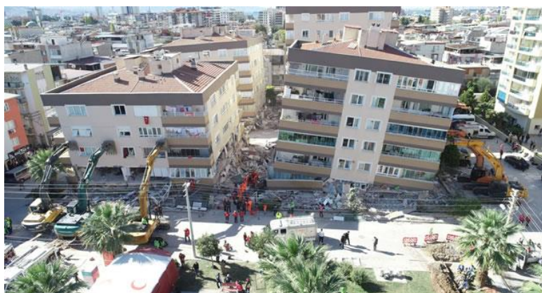
Figure 88: Barış Sitesi Apartments ( https://www.egetelgraf.com/izmirdeki-depremde-hayatini-kaybeden-nurcan-hicyilmaz-tosun-topraga-verildi/ )
