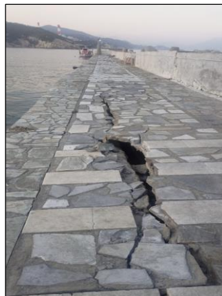
Figure 42: Significant damage was observed on Karlovasi ports of Samos.
