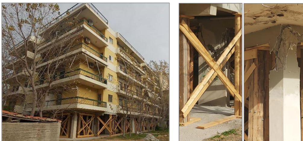
Figure 61: Five-storey building with soft first storey (pilotis) failure at the ground level in Karlovasi (Samos)
