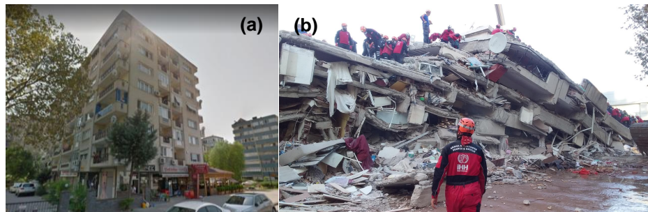
Figure 84: Doğanlar apartment: (a) before (Google Maps) and (b) after the earthquake (photo courtesy of Mauricio Morales-Beltran)
