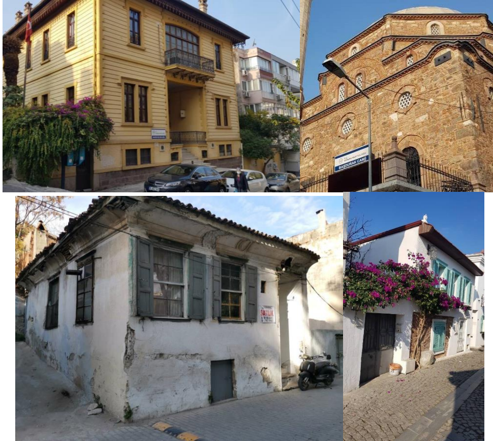
Figure 89: Good response of masonry buildings: (top row) monumental examples in central Izmir; (bottom row) vernacular typologies in Seferihisar
