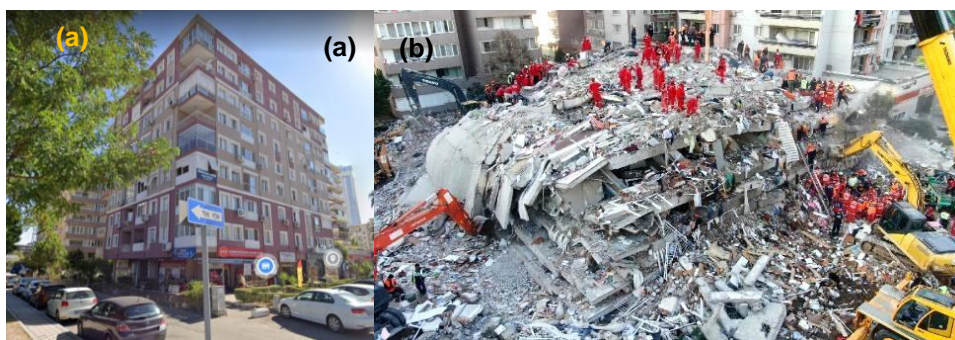
Figure 85: Riza Bey Apartments: (a) before (Google Maps) and (b) after the earthquake ( https://www.haberler.com/riza-bey-apartmani-nerede-riza-bey-apartmani-13705665-haber/ )
