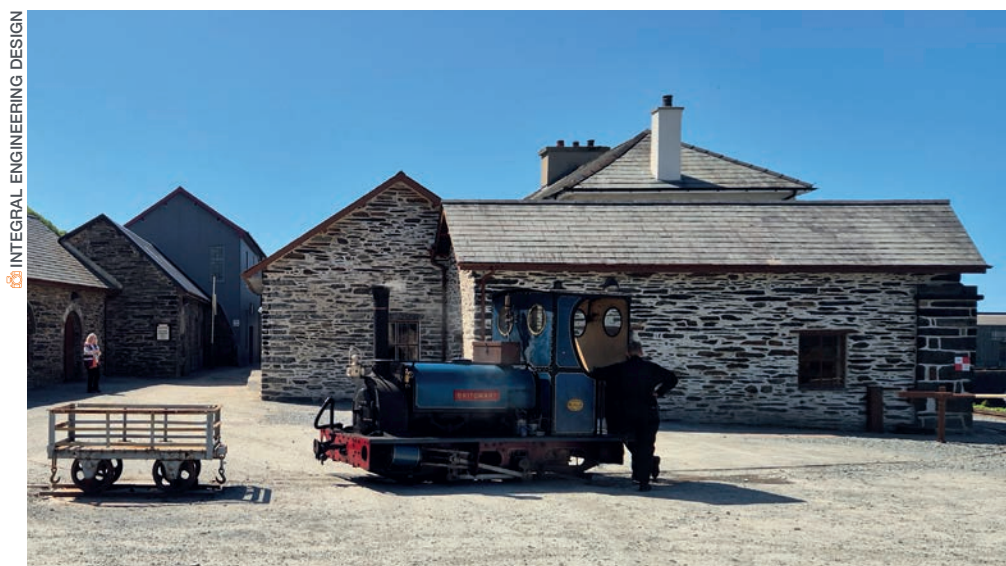
FIGURE 3: Boston Lodge Works for the Ffestiniog and Welsh Highland Railways is a recent highlight in which clever thinking was central to reducing embodied carbon
