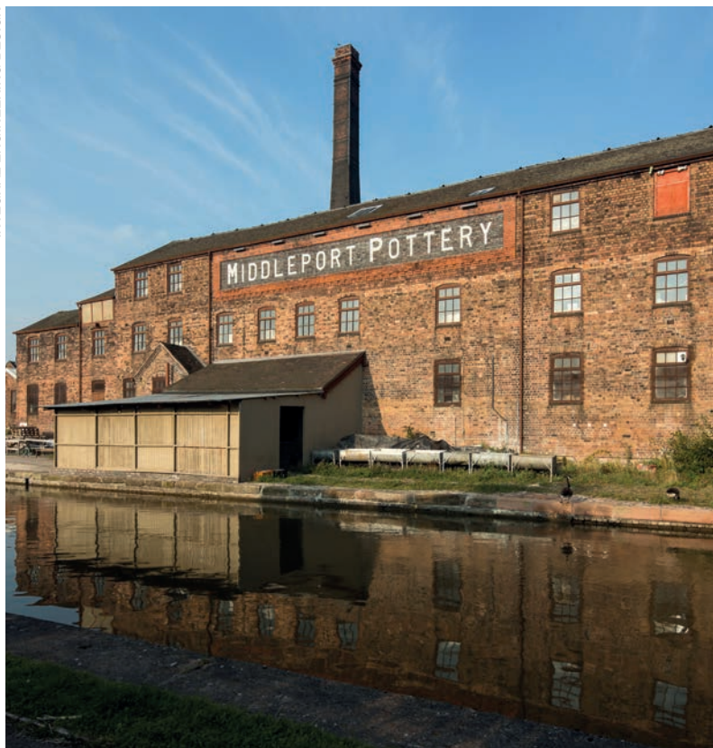
FIGURE 2: Middleport Pottery was another significant conservation project that helped to establish Cooke's reputation
