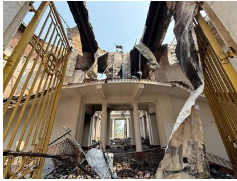
Figure 5.3.2. Earthquake and fire damage to Mandalay University (a) and collapsed ground story at Technological University Kyaukse (b) (Source: Popular News Journal (a); student group via Facebook (b)).
