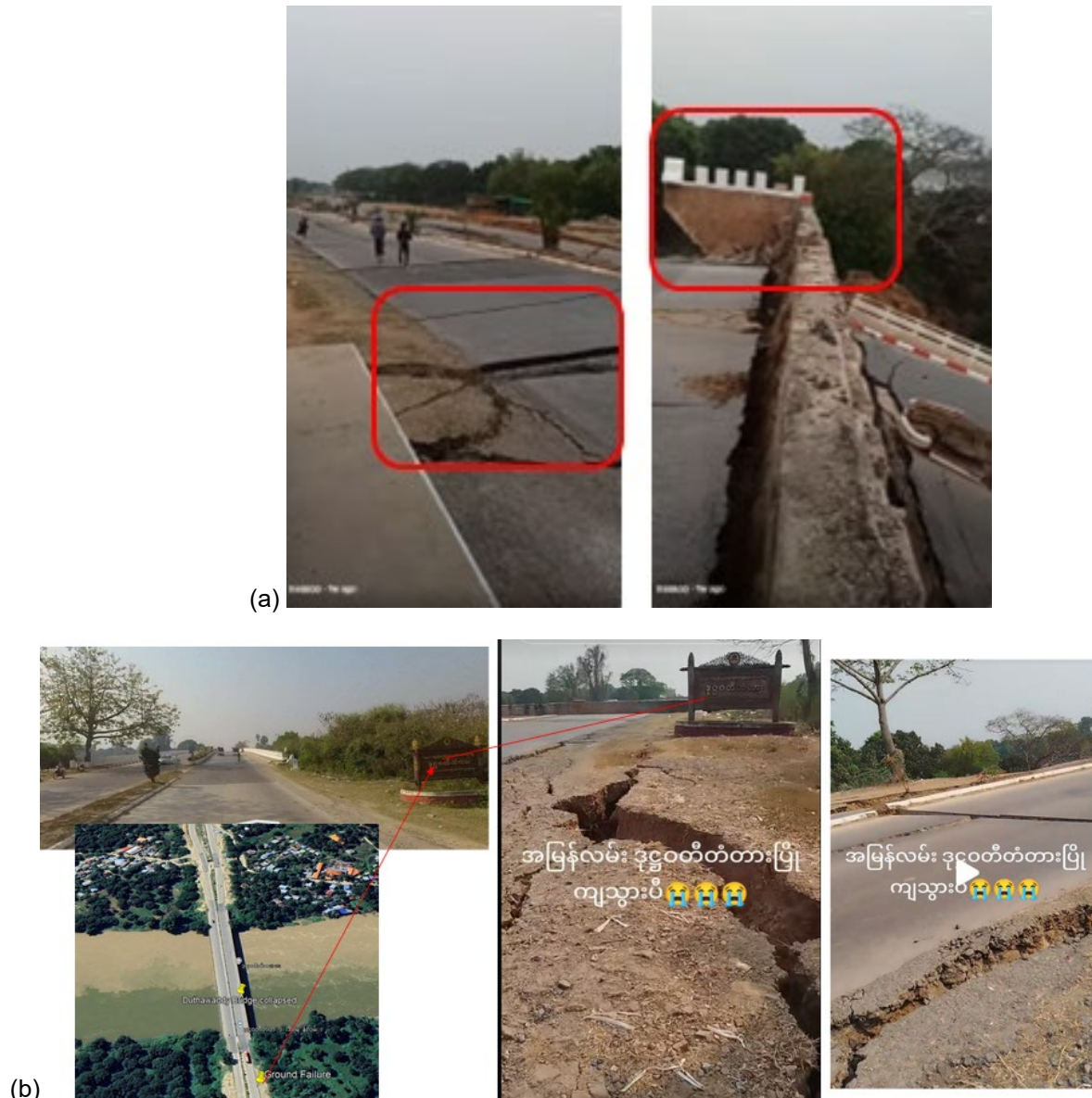
Figure 6.2.4. Dutthawaddy (U Man Lay) Bridge crossing Myitnge River: (a) roadway and abutment damage (Source: Extracted from video from @fri4800 on TikTok ); (b) approach and shoulder road failure with wide separation (Source: Extracted from video from @aungsl1 on TikTok ).
