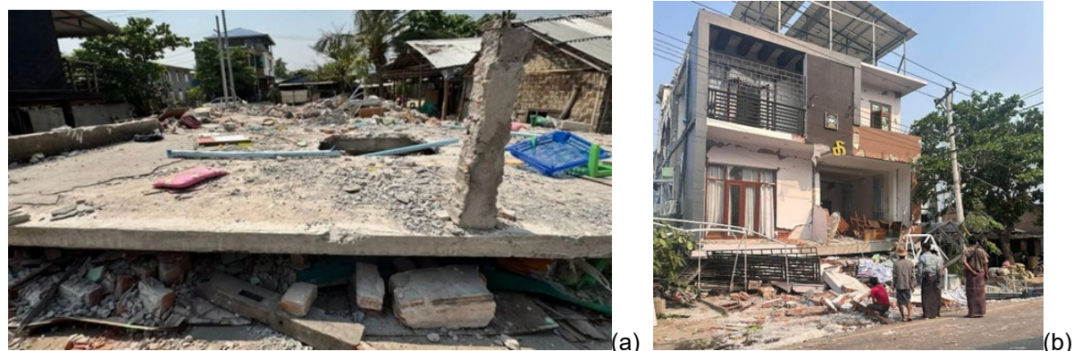
Figure 5.3.1. Collapsed reinforced concrete frames of private schools in Kyaukse (a) and Sagaing (b) (Source: Htet Naing Zaw, BBC Burmese (a); BBC Burmese (b)).
