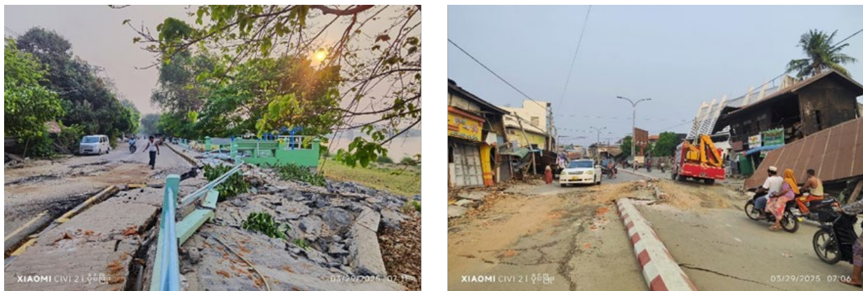
Figure 2.15. Roadways with offset of several feet (21°52'49.27"N, 95°59'5.57"E) (Source: HMSon @heungburma on X ).
