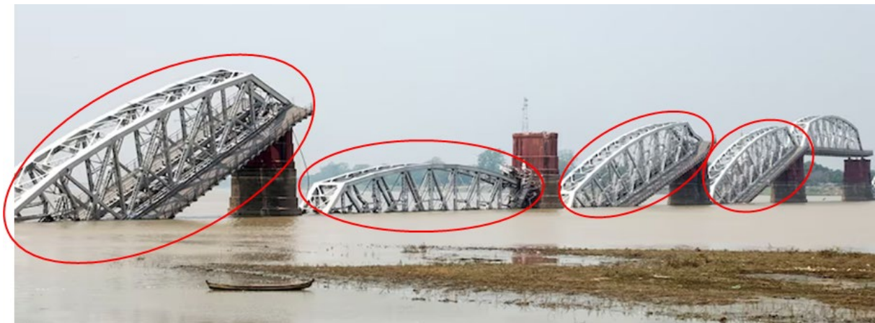
Figure 6.2.2. Unseated bridge decks of the Ava Bridge, noting undamaged piers and fully intact bridge deck sections (Deliso 2025).
