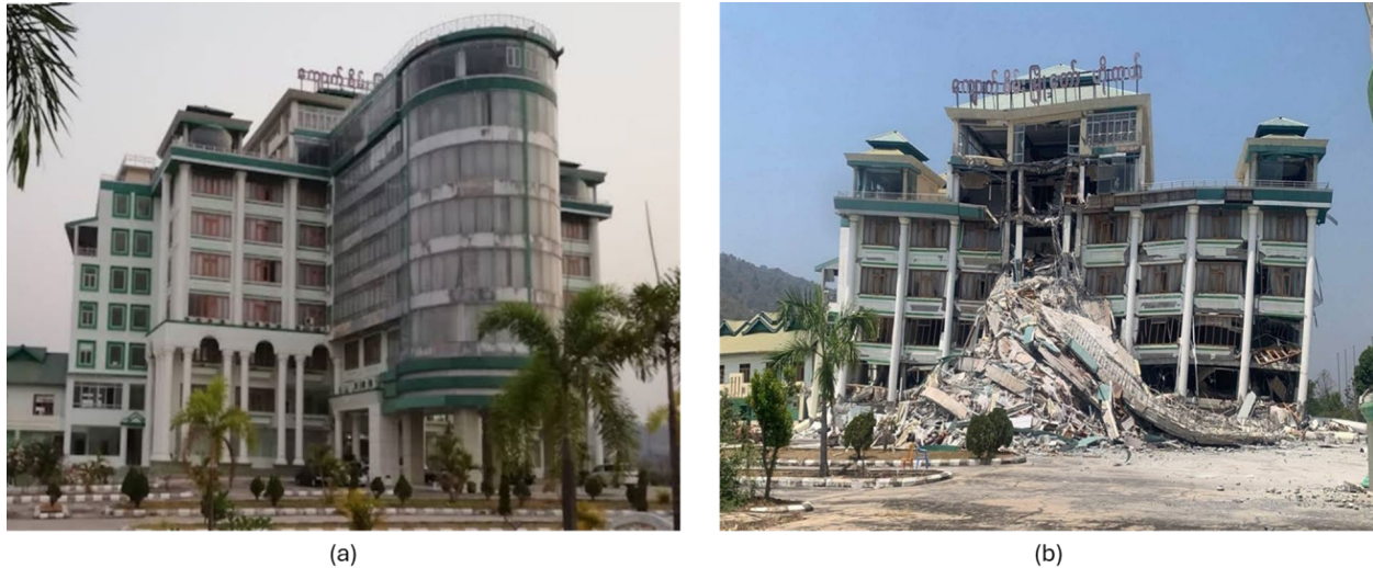
Figure 5.1.5. Jade City Hotel, Nay Pyi Taw, Myanmar [Coordinates: 19.88025,96.15184] (a) before and (b) after the earthquake (Sources: (a) Google Maps ; (b) SiThu Maung on Facebook ).
