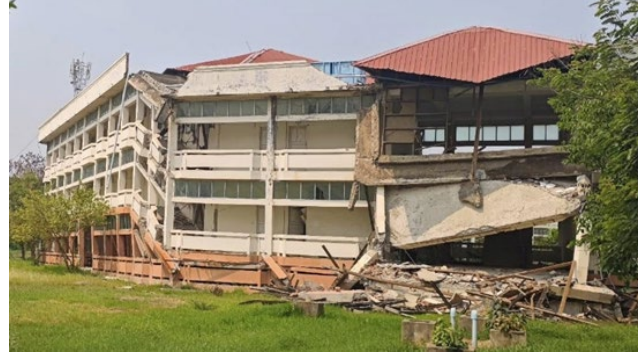
Figure 5.3.2. Earthquake and fire damage to Mandalay University (a) and collapsed ground story at Technological University Kyaukse (b) (Source: Popular News Journal (a); student group via Facebook (b)).
