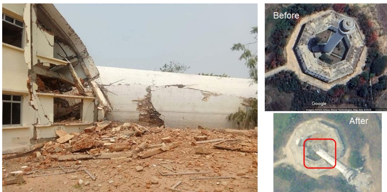
Figure 6.2.7. Collapsed airport control tower of the Nay Pyi Taw airport due to biaxial bending resulting from combined effect of horizontal ground motion components (Source: @heungburma on X ), with aerial imagery of condition before and after earthquake (Sources: before, Airbus, Maxar Technologies; after, Maxar Technologies).
