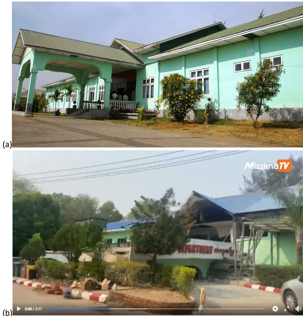
Figure 5.2.2. Nay Pyi Taw General Hospital: (a) back view of the building shows one of the typical reinforced concrete entrance canopies before the earthquake; (b) canopy collapsed at the Emergency Department (Sources: (a) Wikimedia Commons , (b) Mazzina Myanmar , 2025).
