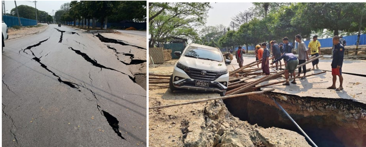
Figure 4.3.3. Extension in pavements along Myo Patt Road [Approximate Location 21.9260, 96.0546] (Credit: ZoMung Thawng).
