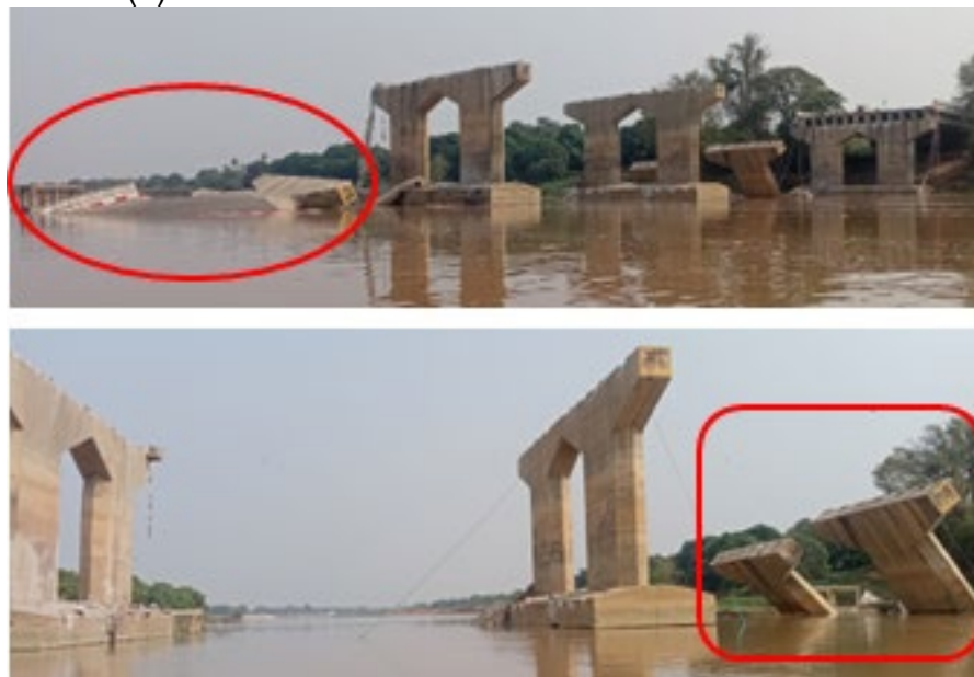
Figure 6.2.3. Dutthawaddy (U Man Lay) Bridge crossing Myitnge River: (a) satellite images before (top) and after (bottom) the earthquake (Credit: Gansu Data and Application Center for High-Resolution Earth Observation System); (b) unseated bridge decks and overturned piers (Source: Khit Thit Media on Facebook ).
