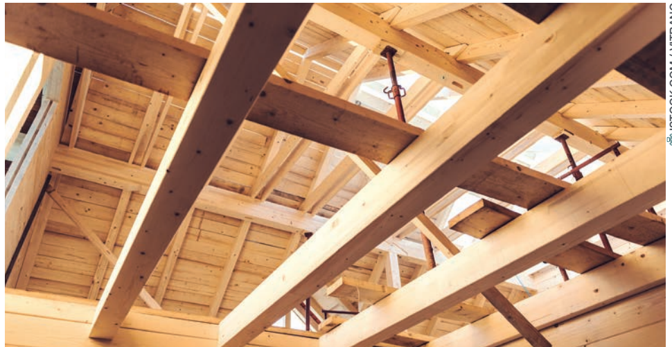
➤ Stock image of timber framed building under construction
