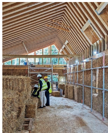
➤ To protect the straw bales from the weather, the roof was constructed first on temporary supports
