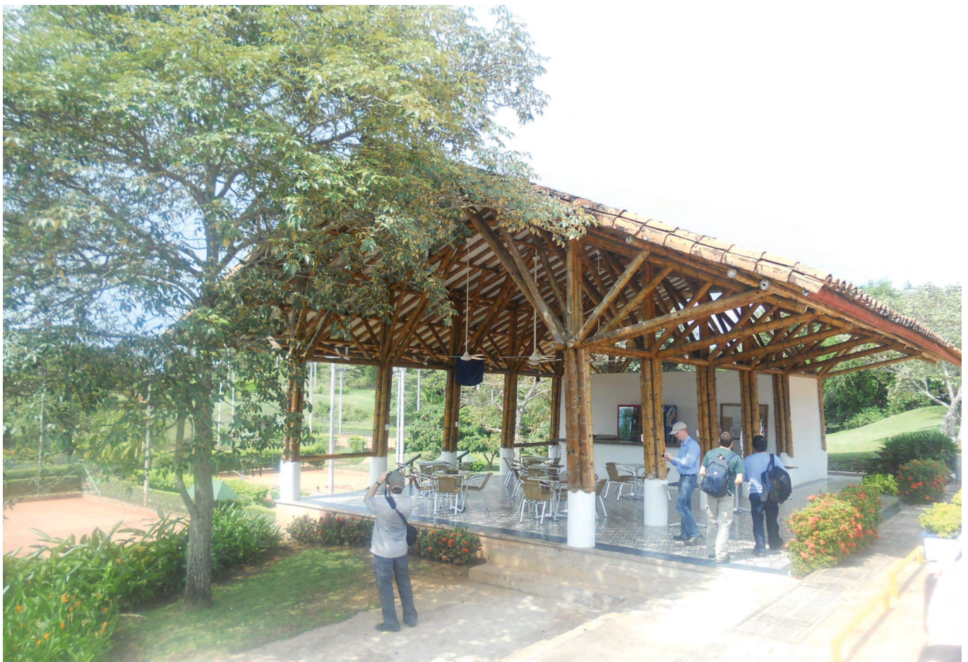
Figure 4.1: Fan-shaped roof truss
