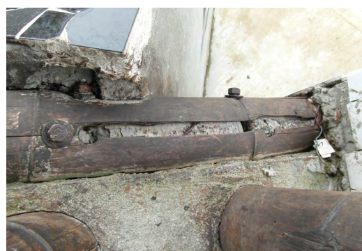
b) Rotten bamboo chord of a bridge, where a bolt hole allowed driving rain to enter; use of mortar infill and surround helped to maintain a moisture-laden environment
