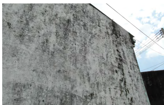
e) Dampness to external wall of modern bamboo house lacking a roof overhang
