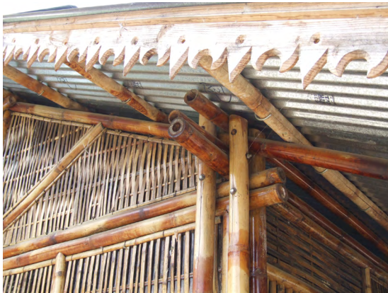
a) Four-culm corner column supporting perpendicular roof truss and rafter
