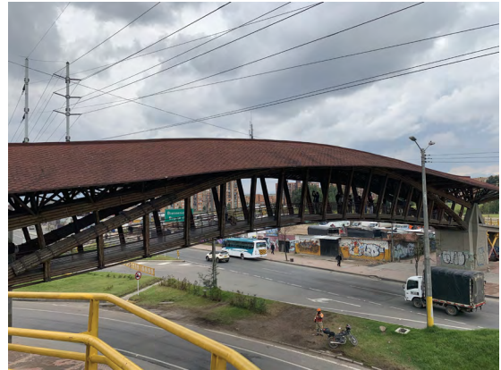
b) Compression members (main arch, arch ribs and roof supports)
