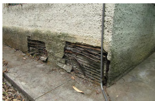
f) Rot to internal bamboo frame of modern bamboo house lacking an upstand and damp-proof membrane; extent of damp region is evident from discolouration
