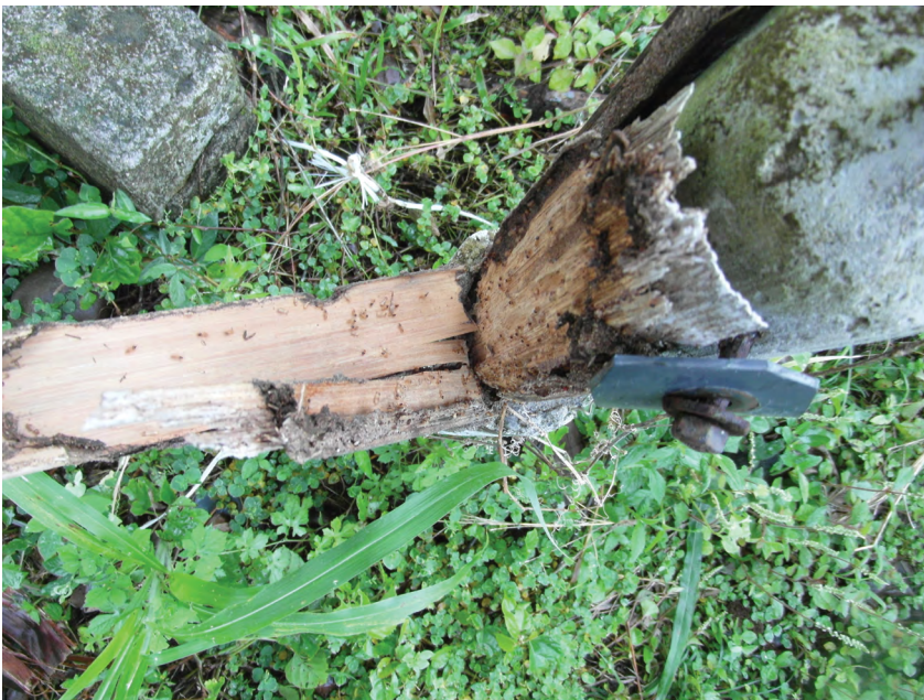
Figure A5.3: Significant termite damage to bamboo columns
