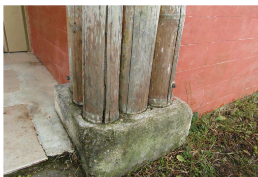
a) Rotten bamboo columns exposed to driving rain
