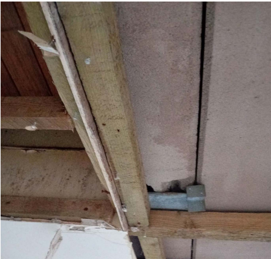
Appendix 1 – 5 Builderswork trimmings around skylights / roof hatches
