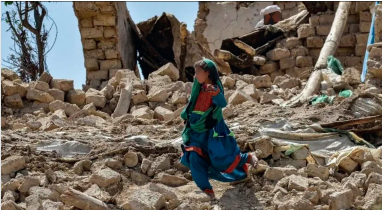
Fig. 5.17: Damaged adobe houses. Unidentified village (BBC News, Getty Image https://tinyurl.com/yc3e8xma )
