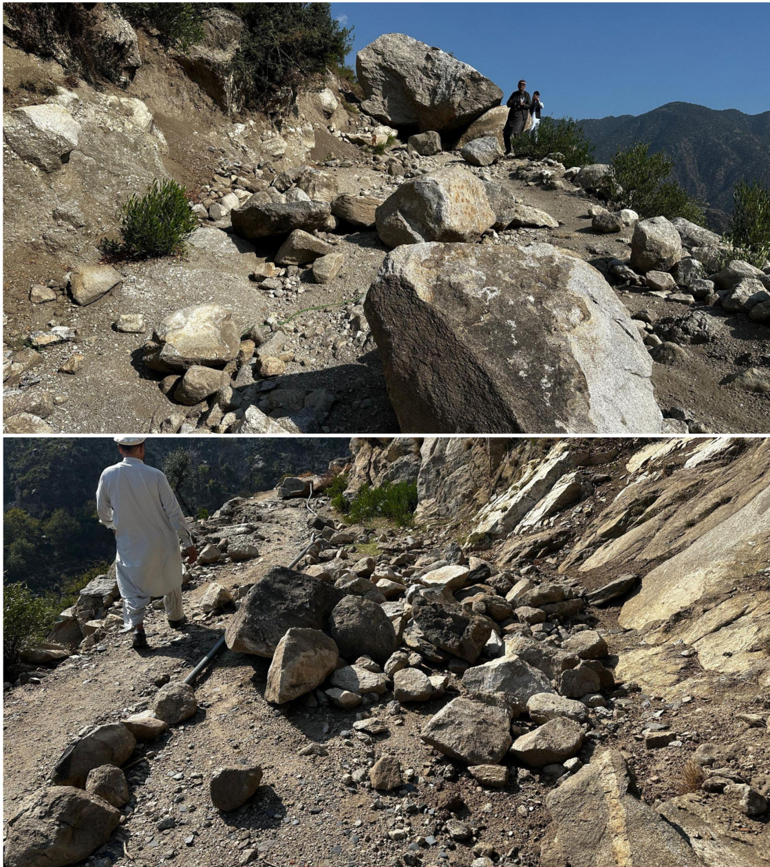
Figure 6.11: Examples of road passage blocking due to rockfalls
