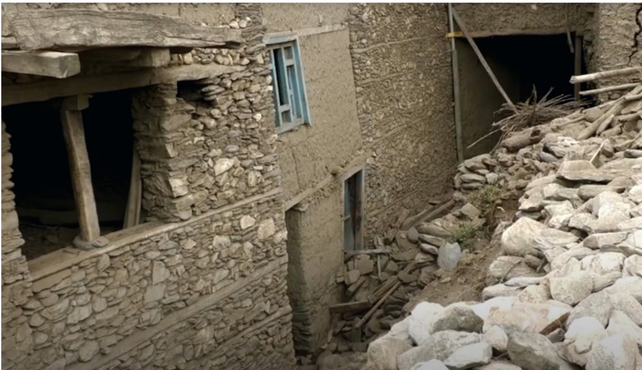
Figure 5.14: Stone and timber structure beside cob construction (Youtube, NewsX World channel https://tinyurl.com/58sbnt8b )
