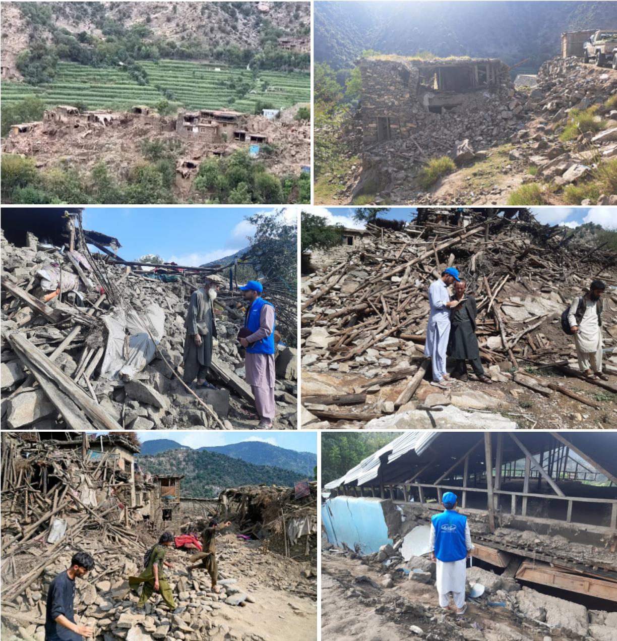
Figure B.3: Earthquake damaged stone masonry buildings in Kunar
