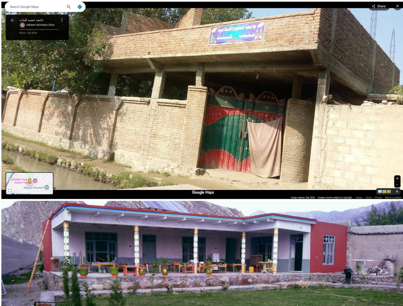
Figure 5.8: Kunar Valley. Top: typical RC and masonry construction; Bottom: RC, masonry and steel
