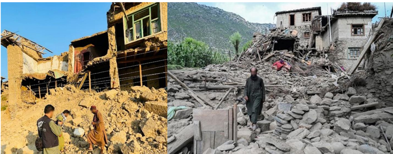
Figure 5.22: Cob walls. The lines marking the interfaces between layers can be clearly distinguished – this technique can be used in the whole structure (credit: NCRO [left]) or on top of a stone masonry ground floor (AFP via Getty Images)
