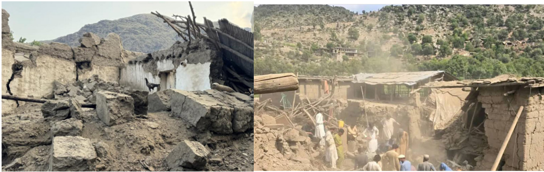
Figure 6.10: Structural devastation of associated industrial infrastructure (UN News, 2025)
