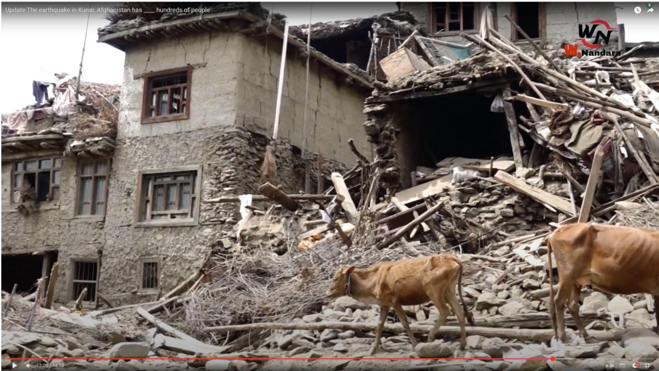
Figure 5.23: Cob wall built on top of a stone wall (YouTube, Watan Nandara channel https://tinyurl.com/yxnchrbsb )
