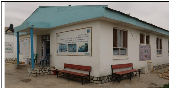
Hazrat Sultan district's health clinic (source: WBA https://www.facebook.com/WorldBankAfghanistan/posts/established-40-years-ago-as-a-health-outpost-and-converted-to-a-health-center-in/896694510758773/ )
