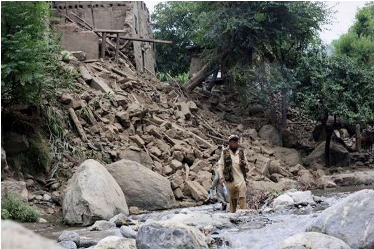
Figure 5.26: Heavy damage to a house sited on sloped ground in Mazar Dara, Kunar province (Associated Press, 2025b)
