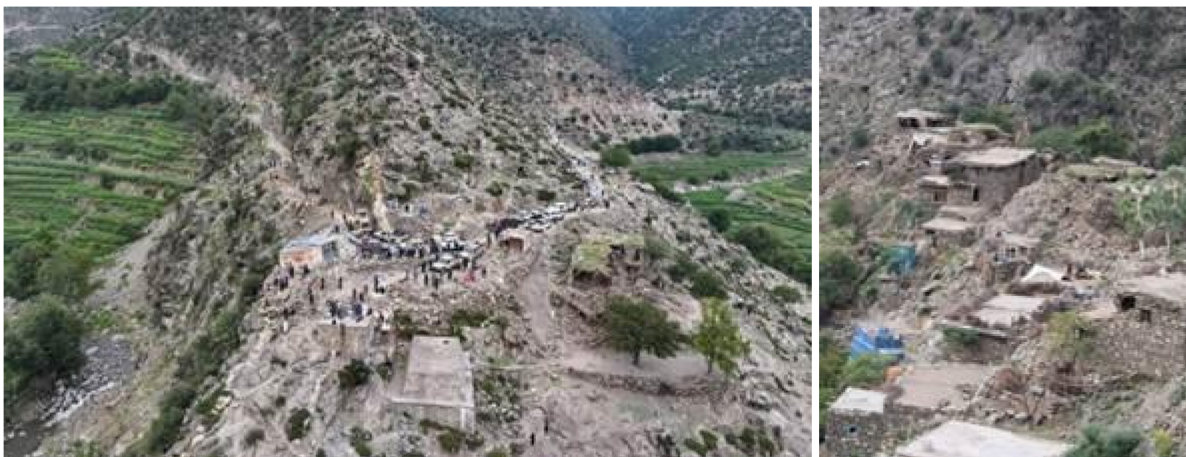
Figure 4.8: Devastation of villages sited on sloping terrain aggravated by landslides (Left: Tareq, 2025; Right: Islamicreliefau, 2025)
