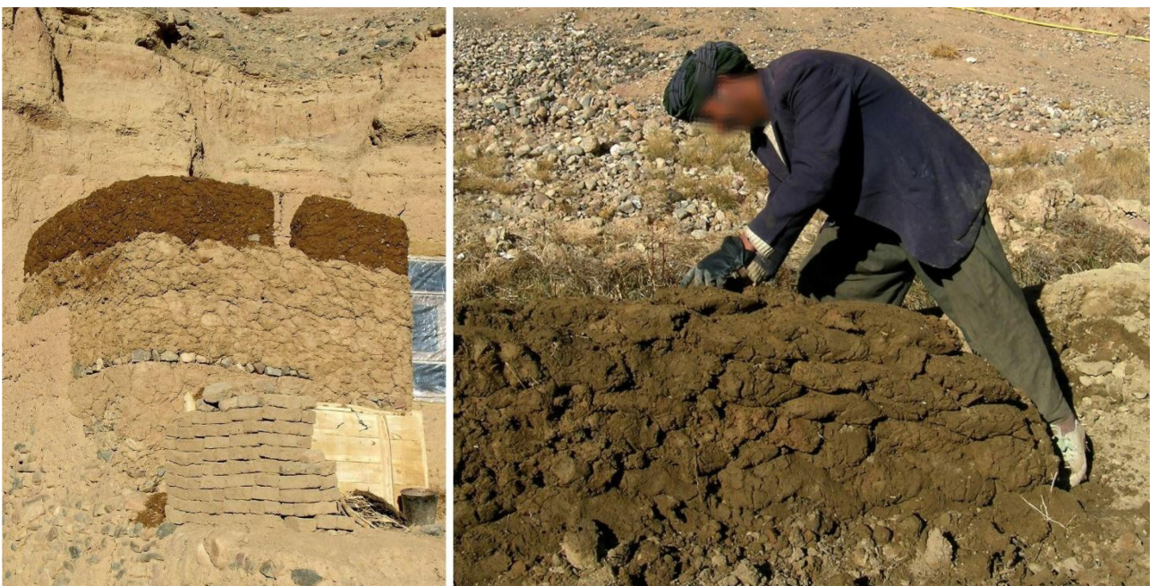
Figure 5.9: Walls under construction in the valley of Bamiyan, Afghanistan
