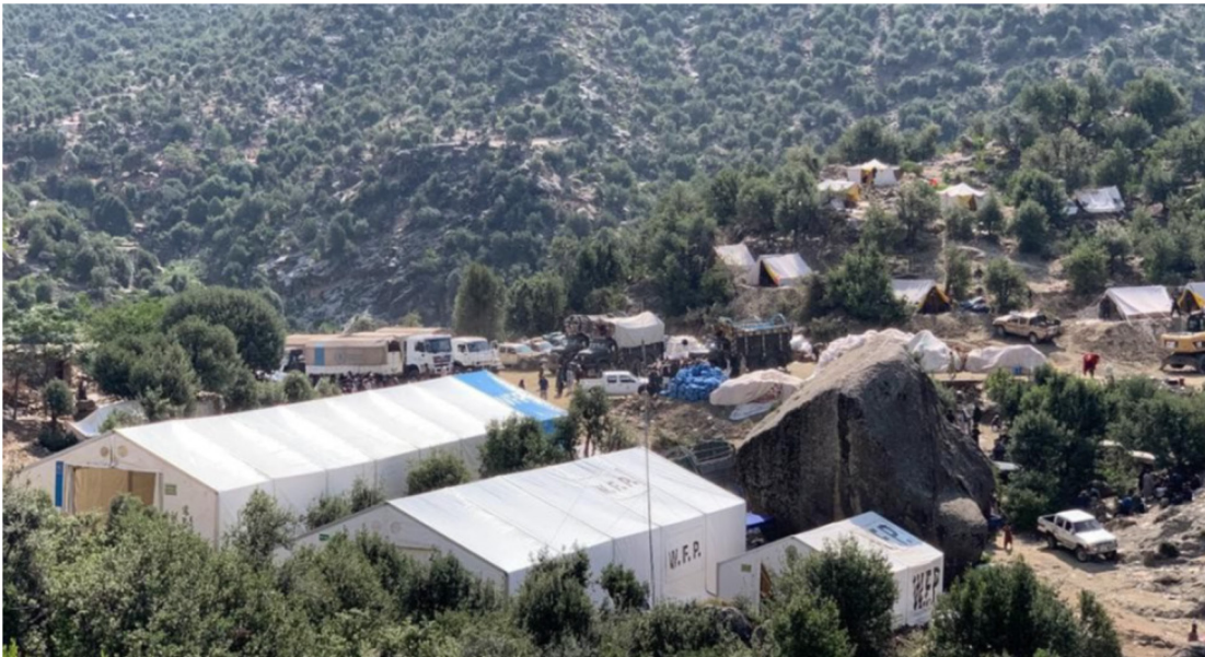
Figure 3.1: Humanitarian Hubs: WFP along with other agencies established humanitarian hub in Mazar Dara of Nurgal and in Dewagal village of Chawkai districts and also installed MSUs in each camp
