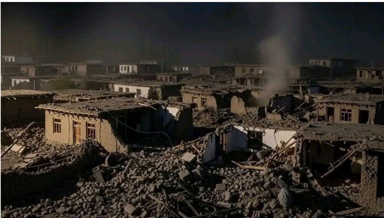
Fig. 5.16: Damaged adobe houses. Unidentified village (India Today NE https://tinyurl.com/2zrdve7e )
