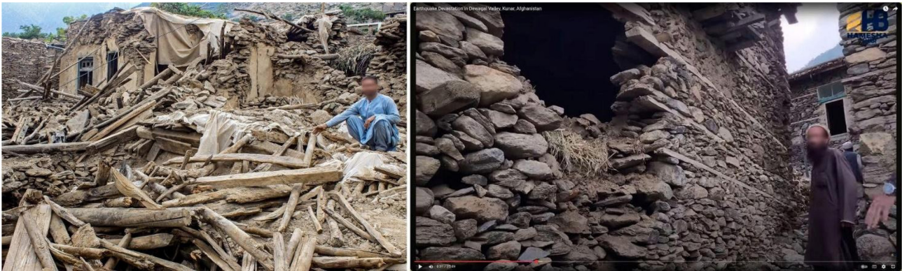
Figure 5.15: A series of damaged stone masonry buildings. Left: AFP/Getty Images; Right: Dewagal Valley (Youtube, Hameshabahar Afghanistan channel https://tinyurl.com/5xacux3v )
