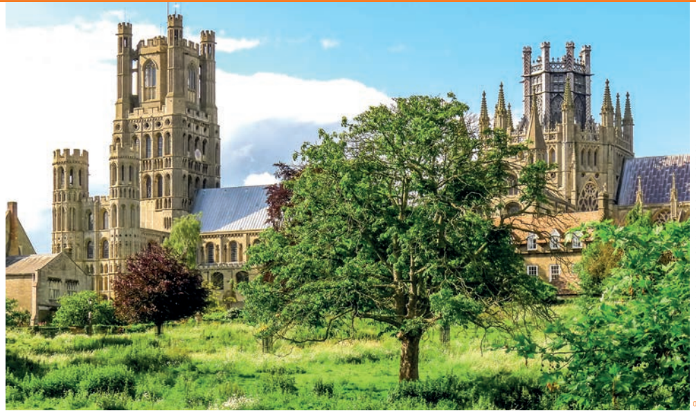
FIGURE 2: Heyman’s developing expertise in structural masonry led to work on many cathedrals, beginning with restoration of the West Tower at Ely Cathedral (pictured, left)
