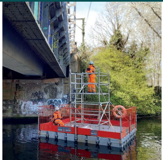
FIGURE 3: Access arrangement for examination of bridge
