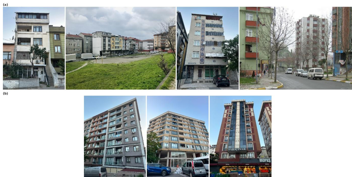
Figure 15: Contrasting residential building typologies, European side of Istanbul. (a) Pre-1994 low-rise RC frame stock representative of the vulnerable building inventory; Ataköy, Bakırköy (photographs 1 and 3: B. Karagöz, 2025); Bağcılar (photograph 2: M. Flesier, CC BY-SA 4.0; photograph 4: İ. Dinç, CC BY-SA 3.0). (b) Post-2000 construction, Ataköy, Bakırköy (B. Karagöz, 2025).
