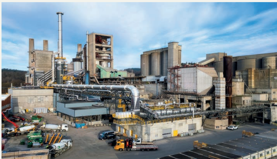
FIGURE 2: Carbon capture plant at Heidelberg Materials' Brevik cement works in Norway
