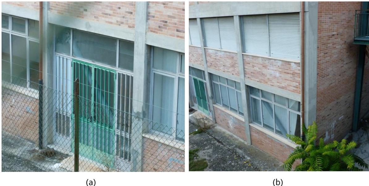
Figure 7-10 Istituto Tecnico commerciale (lat. 42.791702, long. 13.095641), (a), (b) North elevation illustrating tubular steel bracing in bays along the length of the building and possible, repaired damage to the columns.
