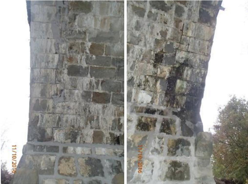
Figure 8-20 Meridian cracks by the side arches, South on the left and North on the right
