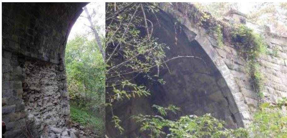
Figure 8-25 North abutment failure (left); detachment of the edge arch at the spandrel connection (right)
