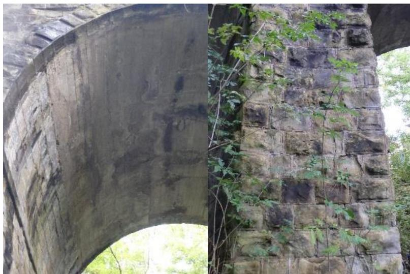
Figure 8-26 Horizontal cracks at the haunch (left), pier vertical cracks (right)
