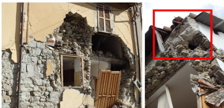
Figure 5-18: a) Detail of masonry wall and ties in Arquata del Tronto Alta; b) details of anchor and ring beam above.
