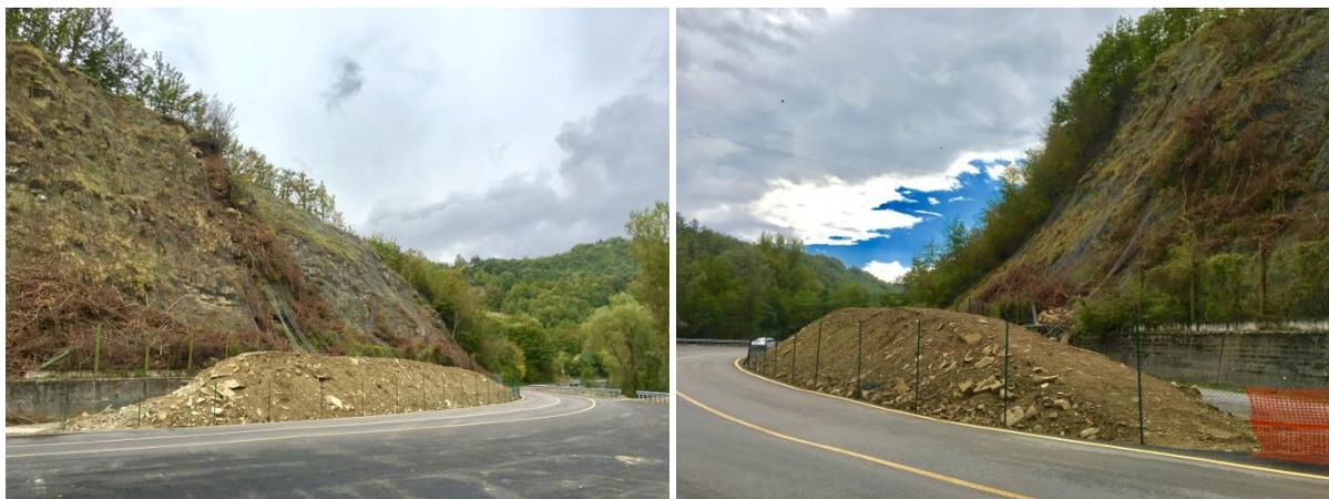
Figure 4-9: Rock fall along the SR260. The detached boulders punched through the wire mesh and catchment fence located above the retaining wall. A protective embankment and new road had been already constructed on the side of the old road at the time of the EEFIT mission.
