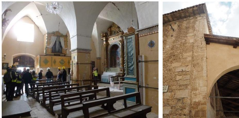
Figure 6-4 Interior view highlighting widespread cracks and detachment of the front façade wall; b) Vertical crack between the façade and the edge spine wall.
