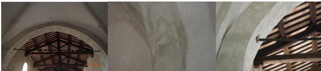
Figure 6-18 View of chancel arch and cracks highlighting hinges formation. Note pull out of the steel tie.
