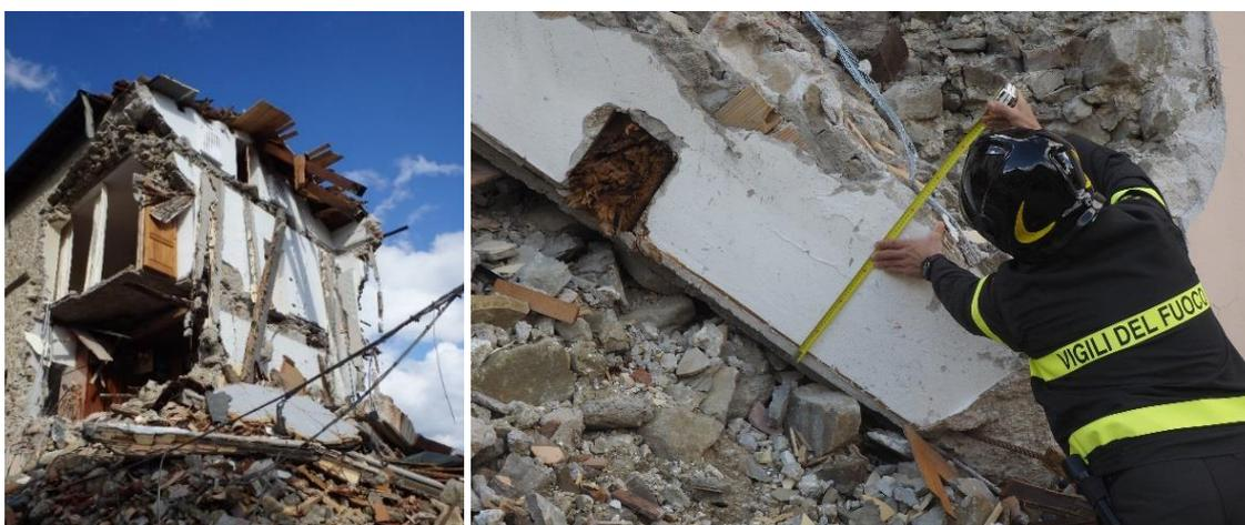
Figure 5-21 a) and b) Collapsed corner building and its ring beam
