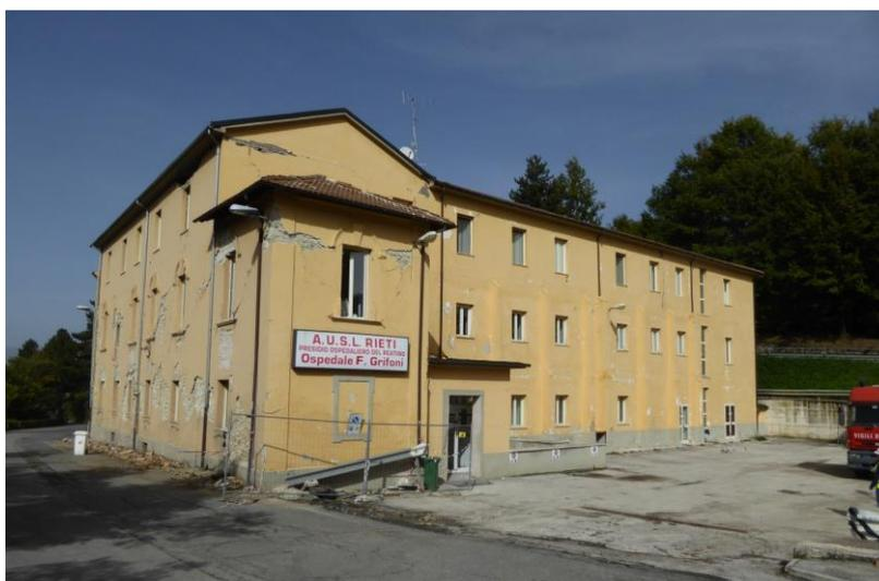
Figure 7-45 Amatrice hospital (lat.  $42^{\circ}37'40.85''N$ , long.  $13^{\circ}17'10.37''E$ ). Three-storey masonry part of the hospital.
