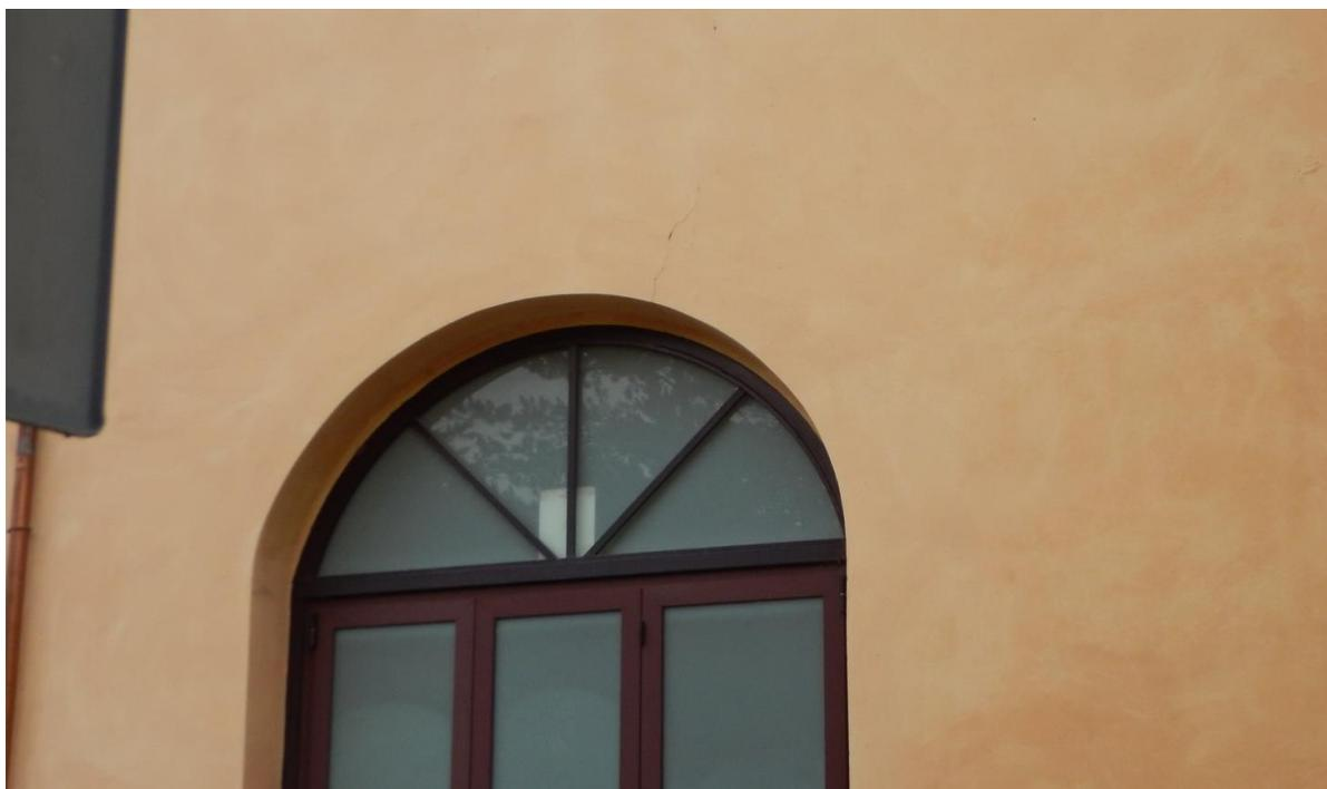
Figure 7-41 Norcia hospital (lat. 42°47'22.83"N, long. 13° 5'50.28"E). Cracking above window.
