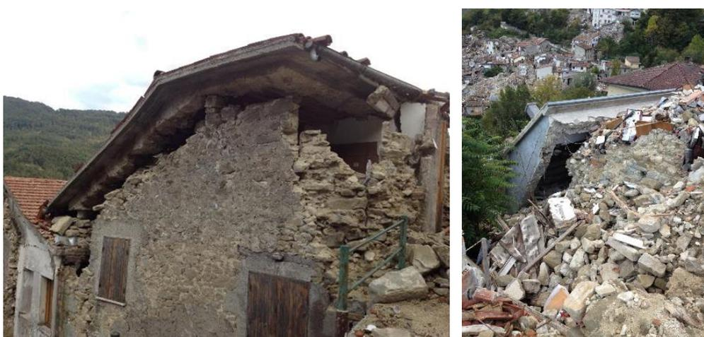
Figure 5-23: Heavy concrete roofs in Pescara del Tronto, causing partial and total collapse
