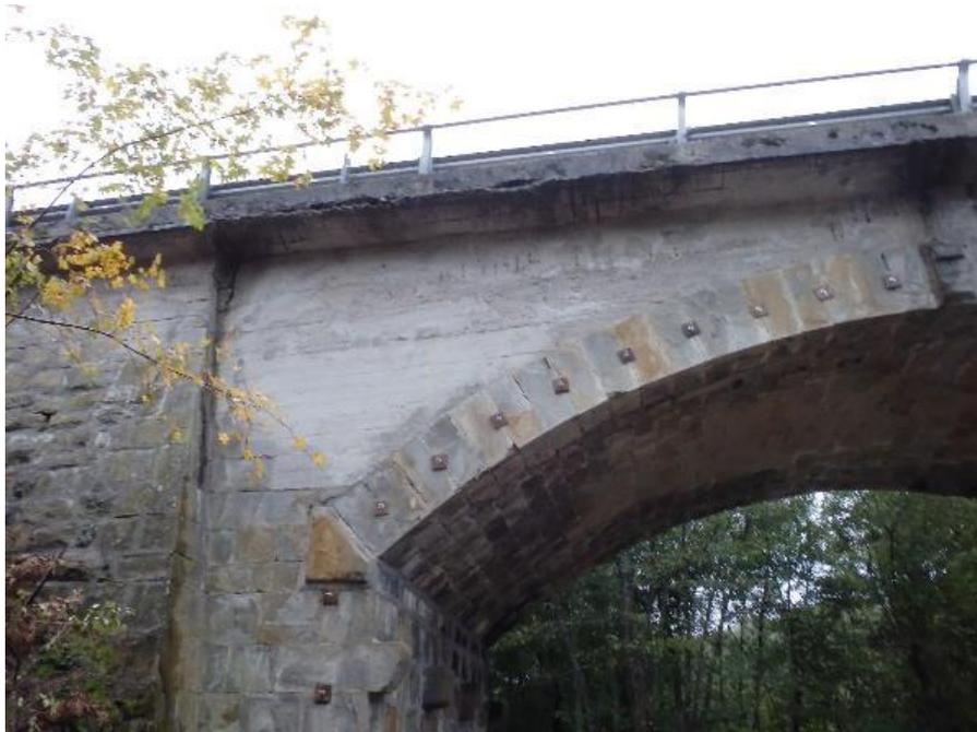
Figure 8-21 Tie rods and concrete spandrel at the bridge North side
