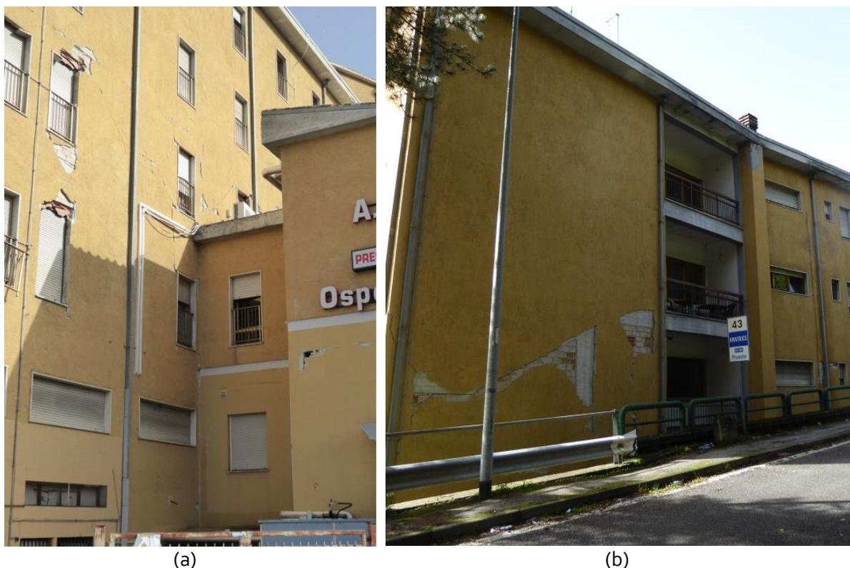
Figure 7-46 Amatrice hospital (lat.  $42^{\circ}37'40.85''\text{N}$ , long.  $13^{\circ}17'10.37''\text{E}$ ). RC part of the building, damage to masonry infills, no structural damage was detected from the survey made from the outside of the building.
