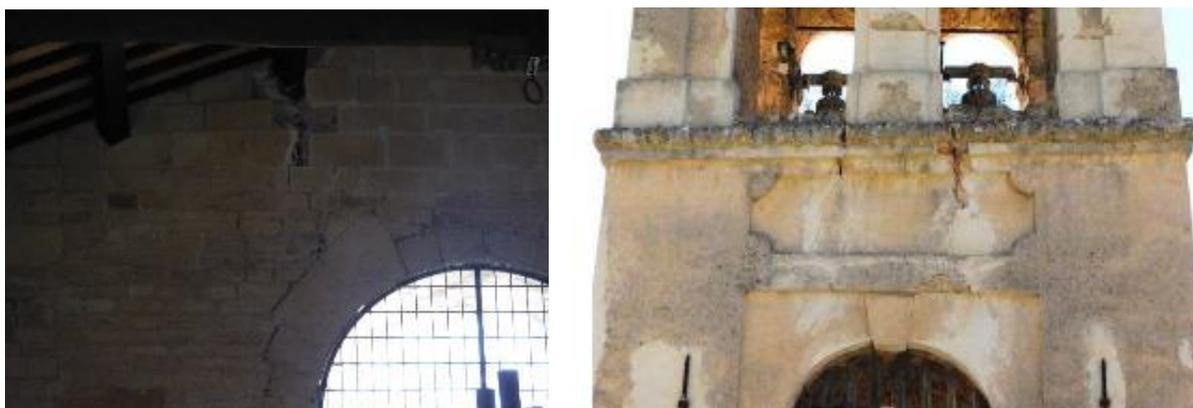
Figure 6-20 a) Cracks on the façade wall by the rose window. b) Cracks on the bell tower.
