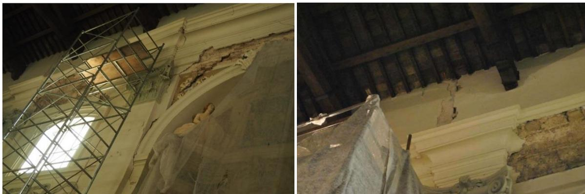
Figure 6-25 Large cracks on the side walls.
