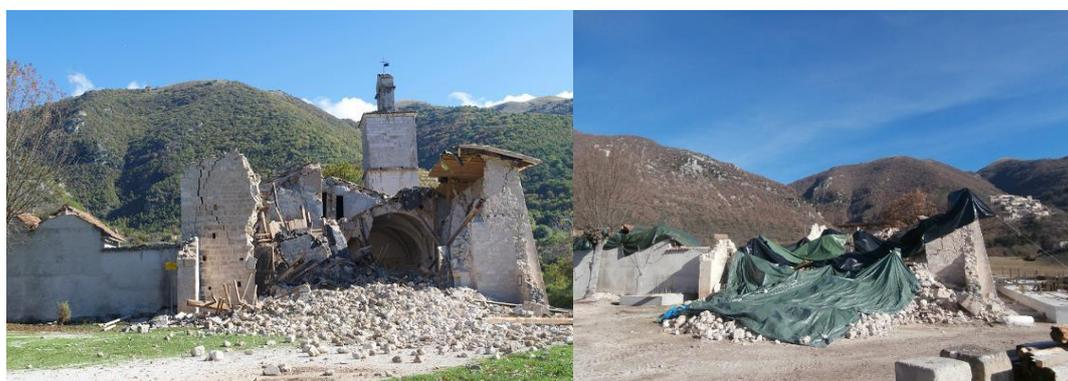
Figure 6-9 a) Church collapse after the 26th October earthquakes (image from <http://www.umbria24.it>); b) Complete collapse after the 30th October earthquake
