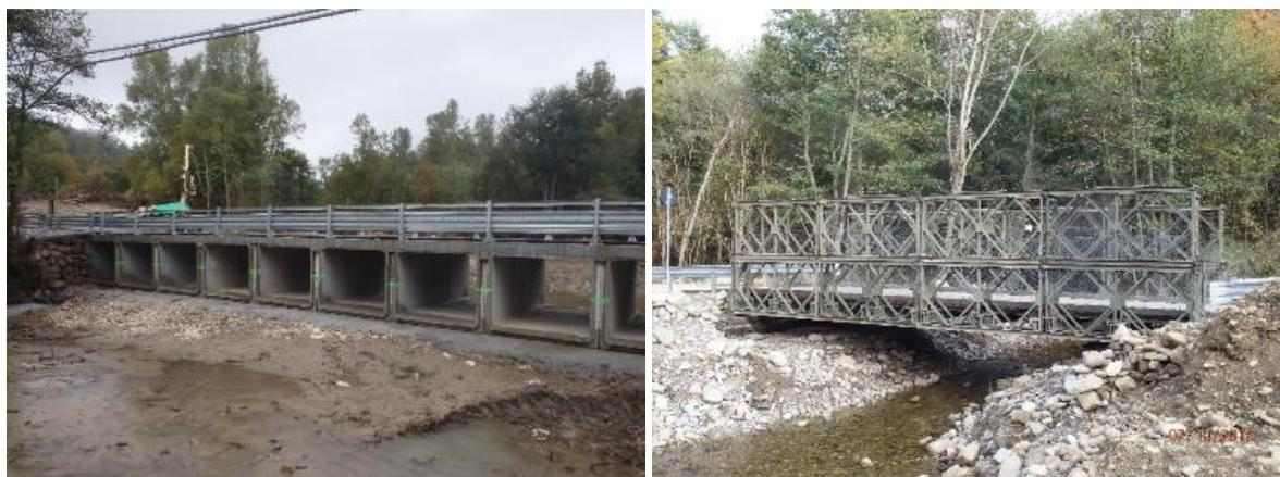
Figure 8-3 Temporary bridge bypassing Ponte a Tre Occhi; b) Temporary bridge near Ponte delle Rose.
