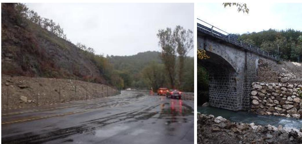
Figure 8-19 SR260 diversion (left), newly made earthworks and gabions at the West abutment (right)
