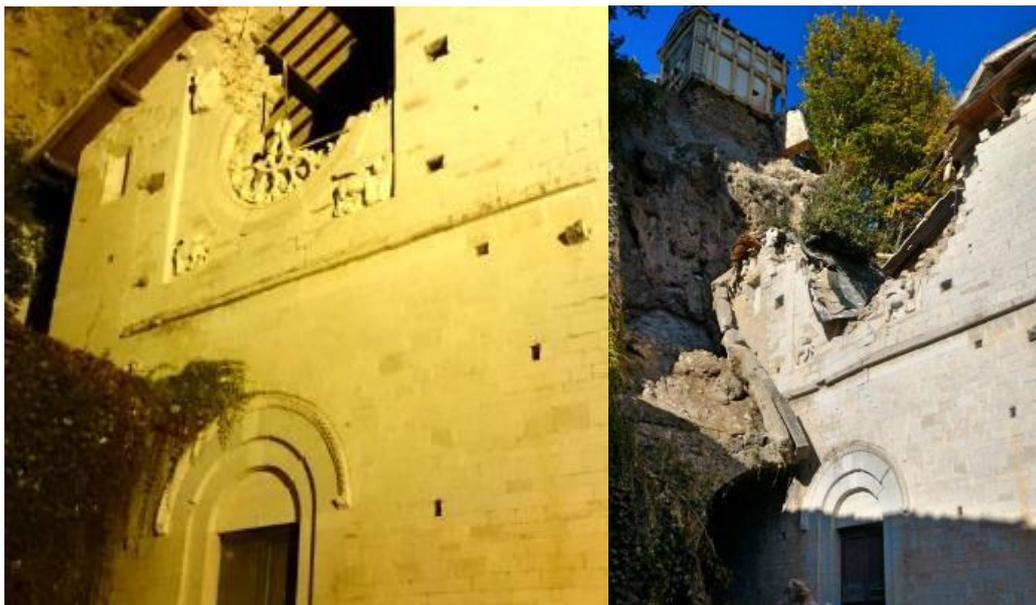
Figure 6-21 Partial façade collapse a) after the 26th October; and b) after the 30th October earthquakes (images from <http://www.umbria24.it>).
