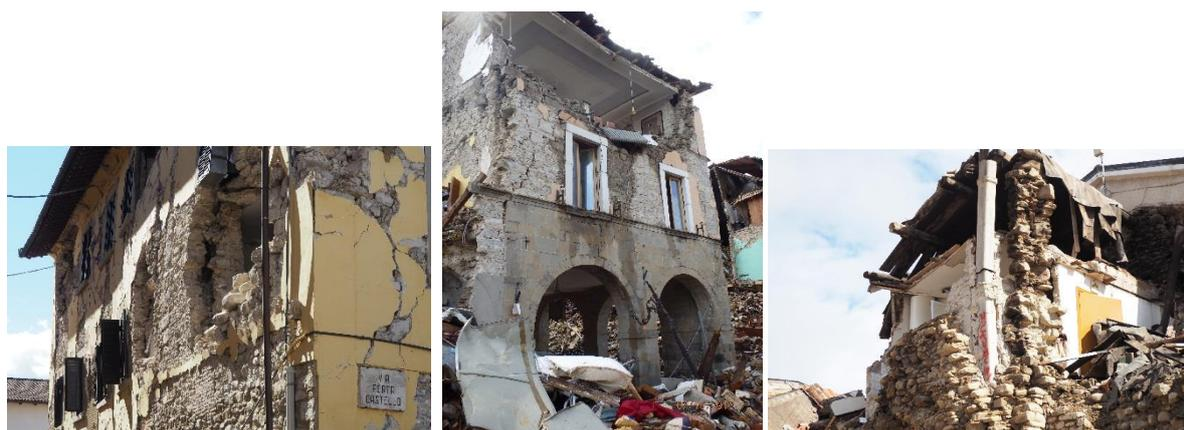
Figure 5-8: Amatrice. a) Typical 2 leaves with cavity masonry wall system. b) Vaulted structures at the ground level of a three storey building. c) Inner chimney, located at the corner of a residential unit.
