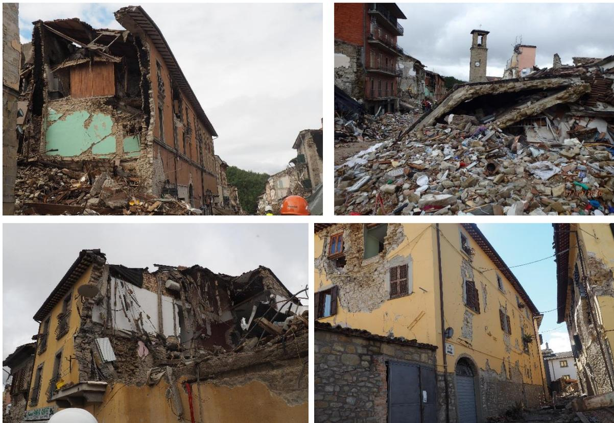
**Figure 5-9: Out-of-plane failures and total collapse caused by concrete roof slabs.**
