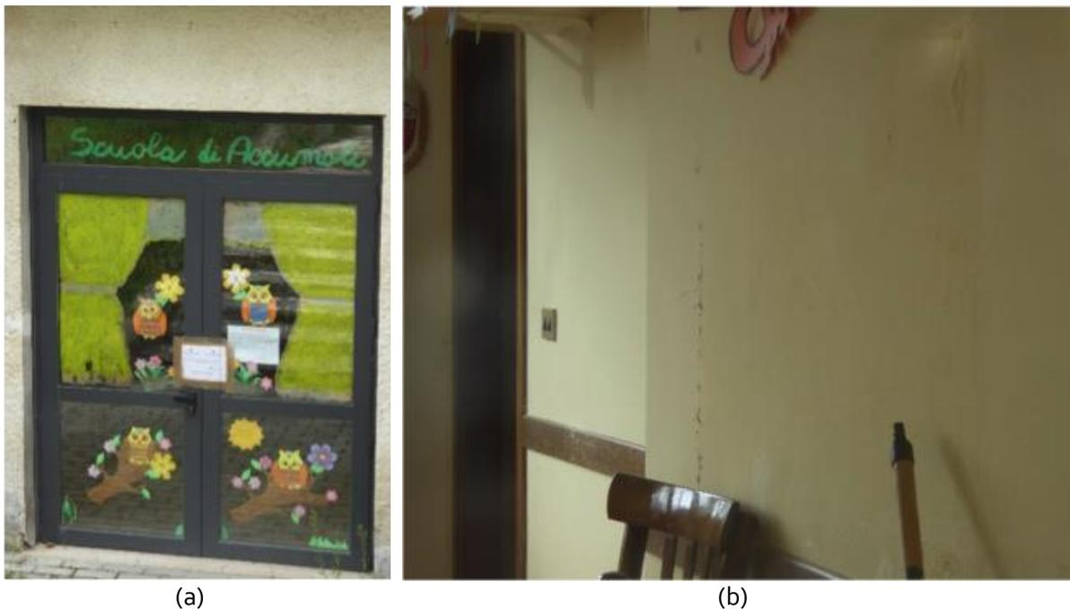
Figure 7-23 Accumoli Scuola dell'Infanzia (lat. 42.693956, long. 13.246677), (a) main entrance of the school with indication of prevented use. (b) cracks in masonry infill walls.
