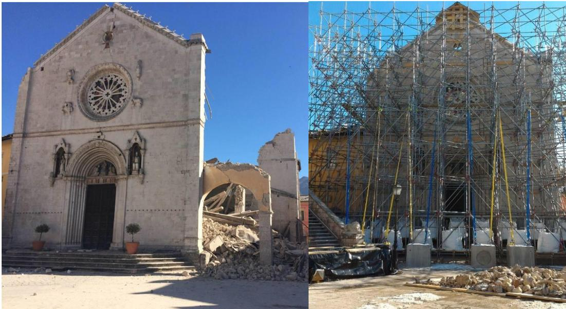
Figure 6-28 Cathedral front façade still standing after 30th October earthquake (note the vertical crack), and with the shoring structure installed in December (images from <http://www.umbria24.it>).
