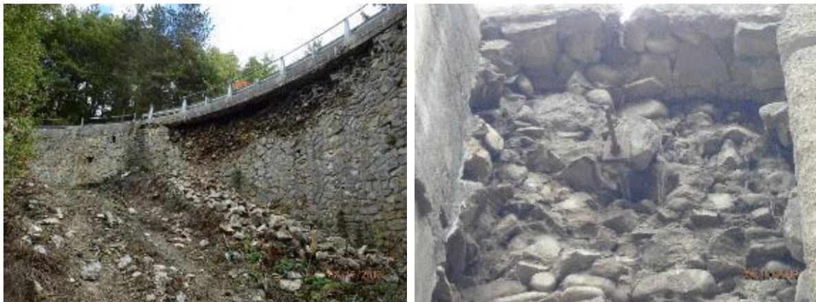
Figure 8-9 Failure of the East abutment northern wall; b) detail of tie rod anchorages exposed
