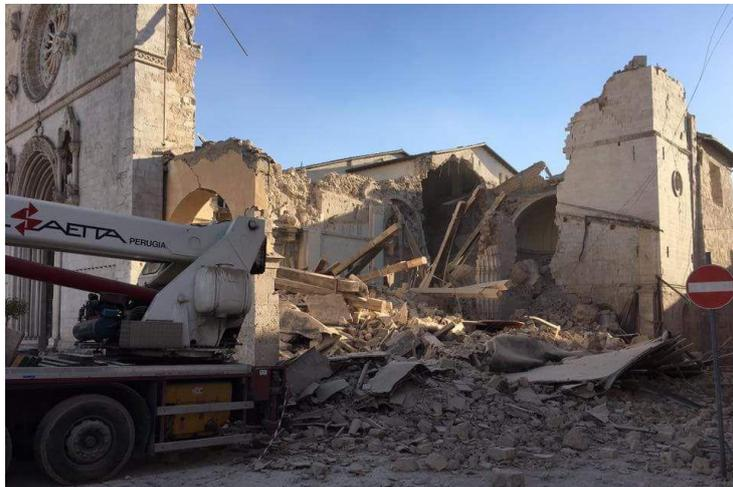
Figure 6-27 Collapse of the S. Benedetto Cathedral following the 30th October earthquake (image from <http://www.umbria24.it>).
