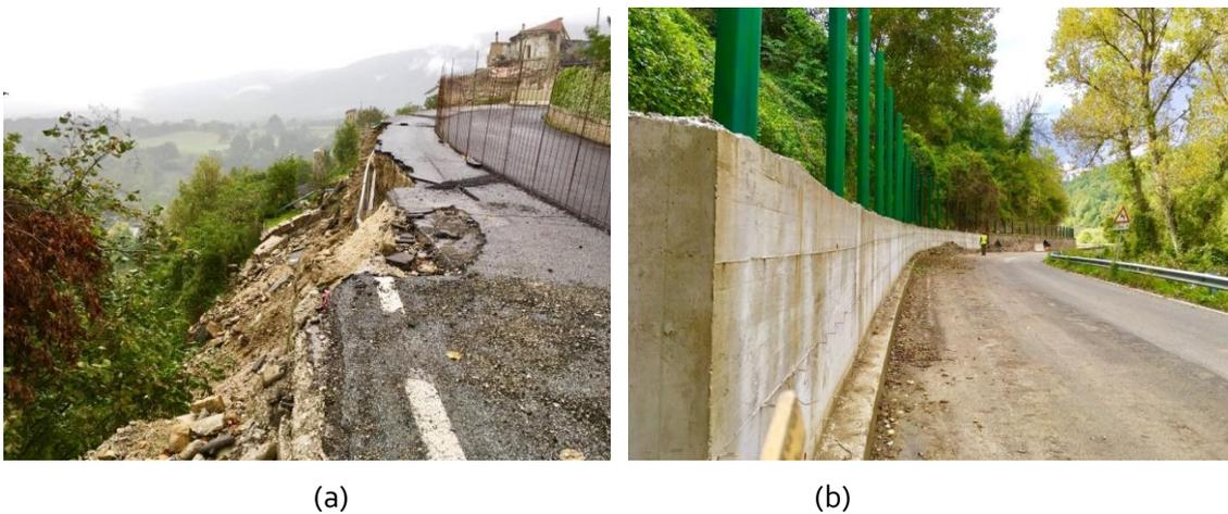
Figure 4-7 : Slide and retaining wall failure observed along SS26o road on the northern-western part of Amatrice: (a) view from the crest and collapsed retaining wall whose debris are visible in the background; (b) view from the base. The displaced material had already been removed and a new retaining wall was being constructed at the time of the EEFIT mission (October 2016). An existing undamaged retaining wall is visible in the background.
