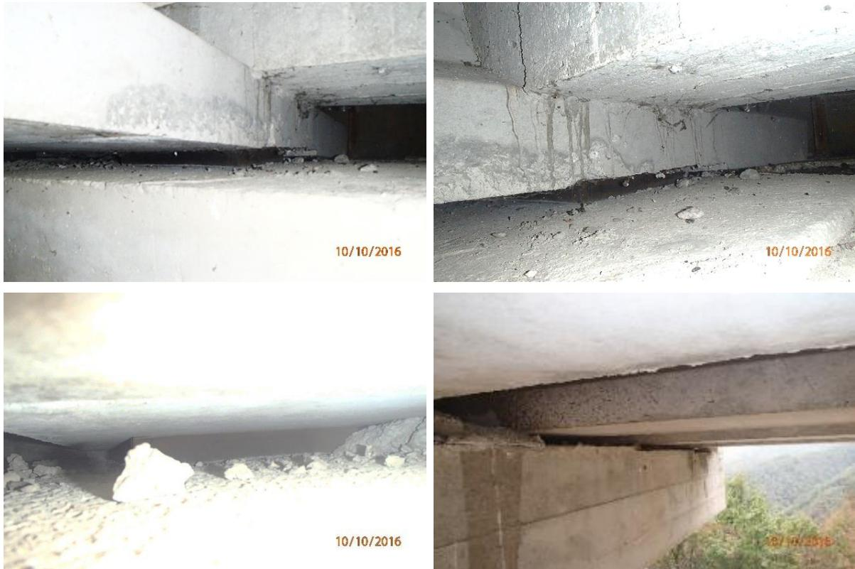
Figure 8-35 Bearing pads of the second viaduct investigated
