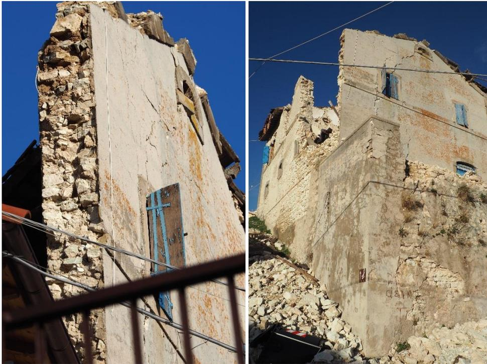
Figure 5-32 a) and b) Failure Mechanisms: partial overturning of the façade and collapse of the corner
