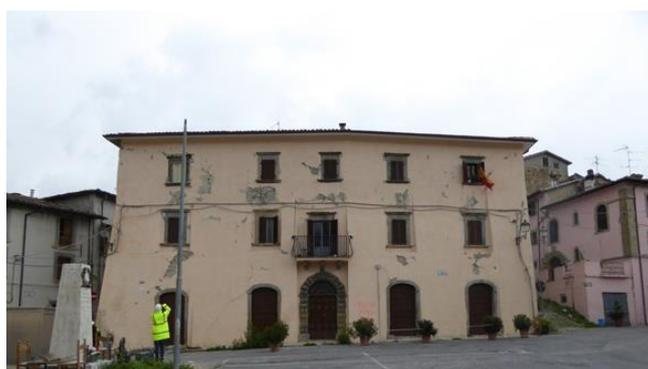
Figure 5-3 Alignment of vertical openings in the main square in Accumoli. The building also has buttresses to the first two storeys of the façade
