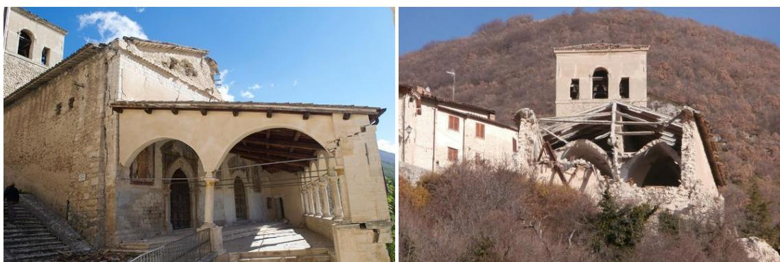
Figure 6-5 a) Damage to the front façade and entrance porch after the 26th October shocks (courtesy of Ing. Andrea Giannantoni); b) Collapse of the front façade and entrance porch after the 30th October earthquake.
