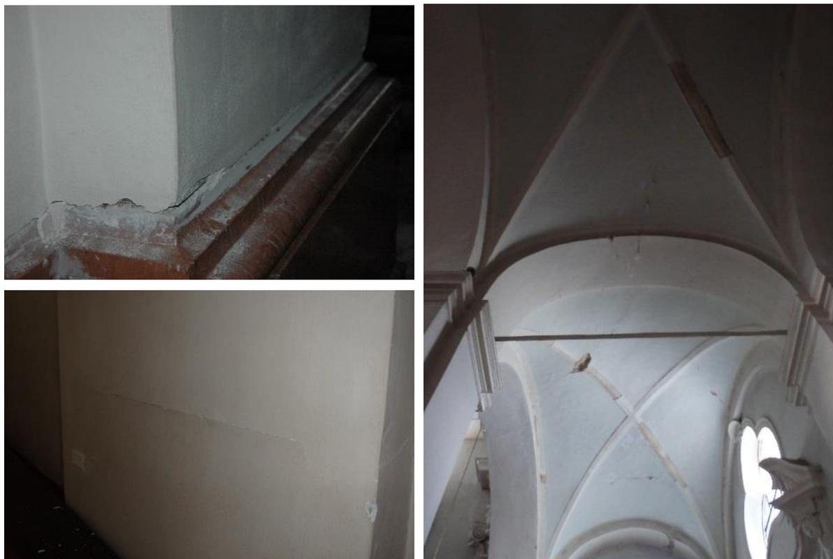
Figure 6-31 a) East aisle cracks at the pillar base (top left), b) at the vault crown (right) and c) at the side wall base (bottom left).
