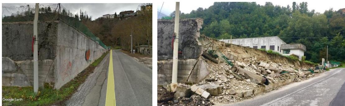
Figure 4-8 : Retaining wall failure located in the locality "Ponte Sommati": (a) Google street view before 24th August 2016 event; (b) collapsed retaining wall.
