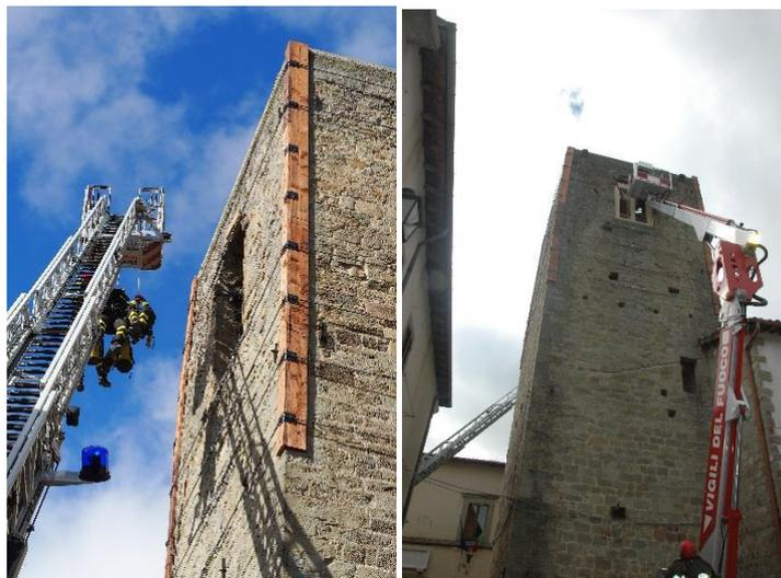
Figure 5-14 : Civic Tower in Accumoli: live intervention by Vigili del Fuoco to secure the tower with temporary shoring and hoops
