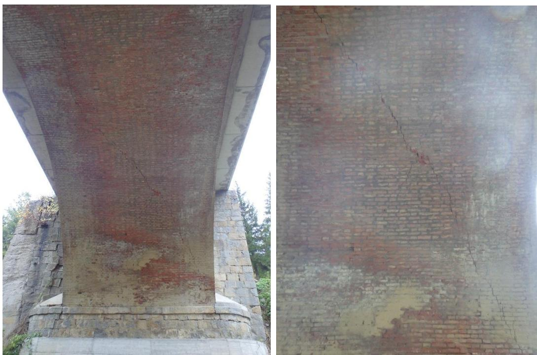
Figure 8-10 Photographs of the eastern arch X-shaped cracks.
