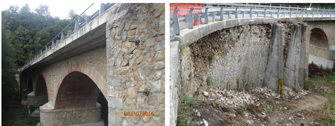
Figure 8-4 "Ponte a Tre Occhi" bridge southern view. Concrete buttresses on the eastern abutment
