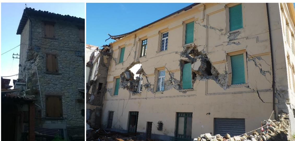
Figure 5-7: a) stone masonry building with ties and grouting of the rubble stone masonry in Pescara del Tronto; b) ONMI Institute in Amatrice, where seven people died. The concrete beams can be seen punching through the façade.
