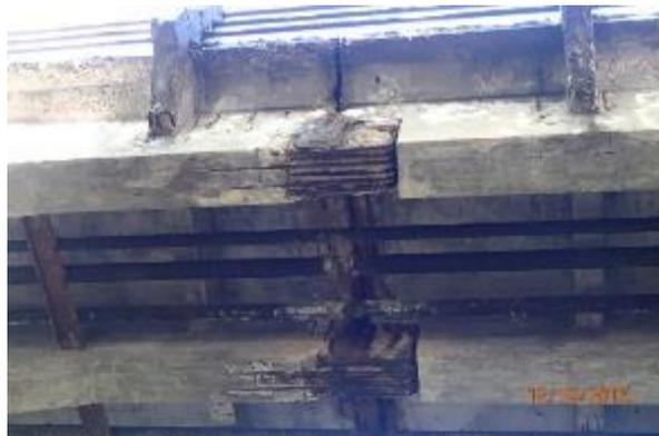
**Figure 8-29 "Sedia Gerber" type joint at the middle span**
