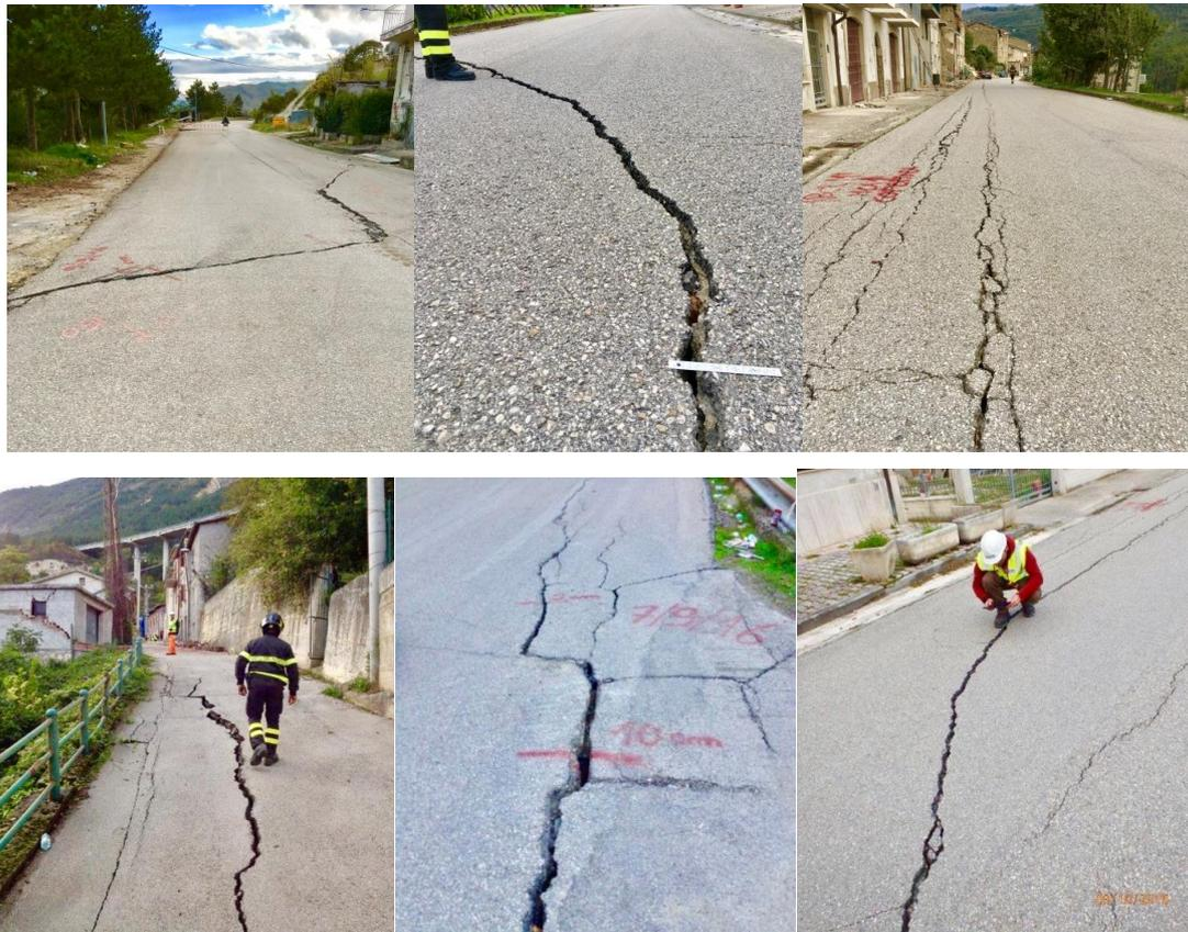
Figure 4-22: Ground cracks on paved roads along SP129 road.
