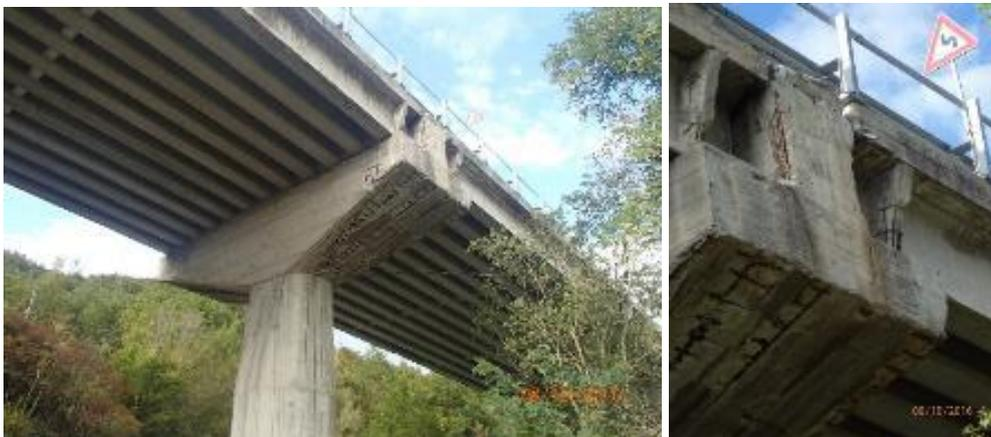
Figure 8-33 Damage observed on the first viaduct investigated ( $42^{\circ}45'23.6''\text{N}$   $13^{\circ}16'37.6''\text{E}$ )
