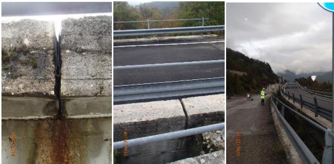
Figure 8-36 Expansion joint and repair works on the surface of the second viaduct investigated
