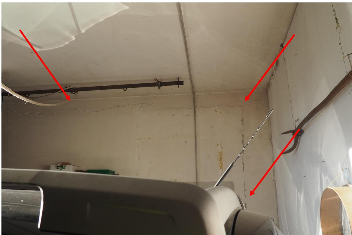
Figure 5-34 Cracks surveyed in RC buildings in Castelluccio di Norcia
