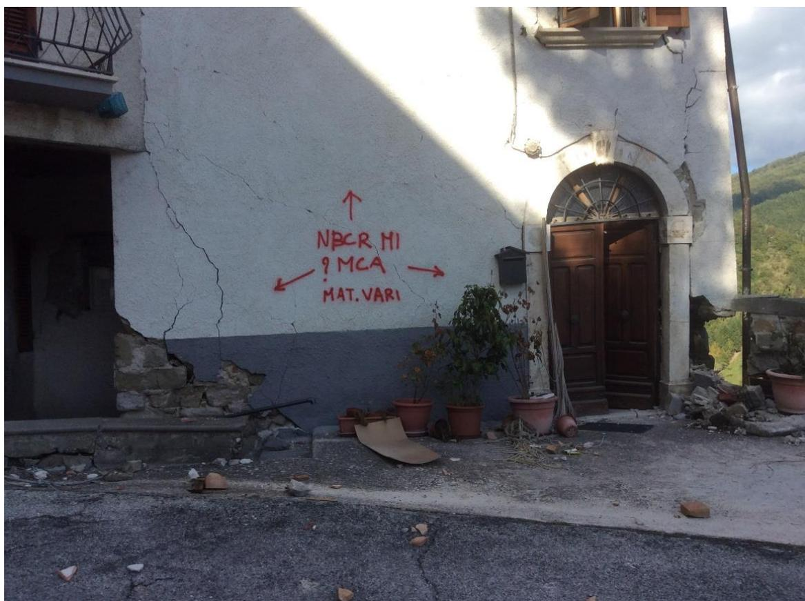
Figure 9-2 Fire Service notation of hazardous materials in a damaged building
