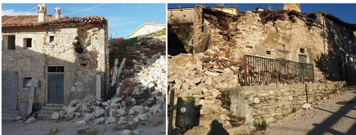
Figure 5-31 Traditional stonework and horizontal structural elements in Castelluccio
