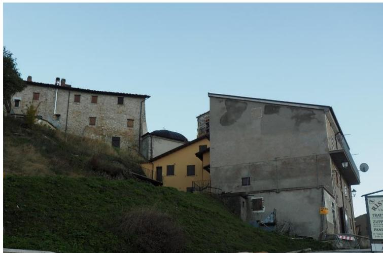
Figure 5-33 Typical residential building on steep slope. The building on the right is a concrete frame. The damage observed in this structure is shown in Figure 5-34
