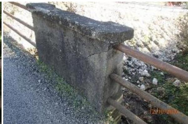
**Figure 8-28 Damage on the parapet and details of the parapet**
