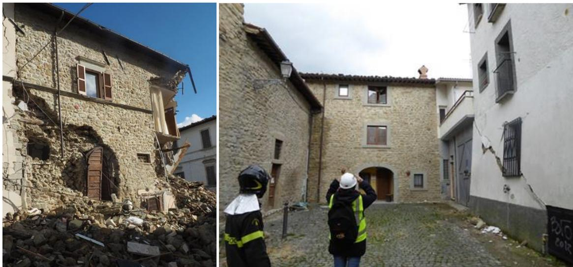
Figure 5-6: Consolidation of local masonry fabric: a) poor grouting in Arquata del Tronto; b) adequate quality grouting and rc frames around opening, delivered a better seismic performance (Amatrice)
