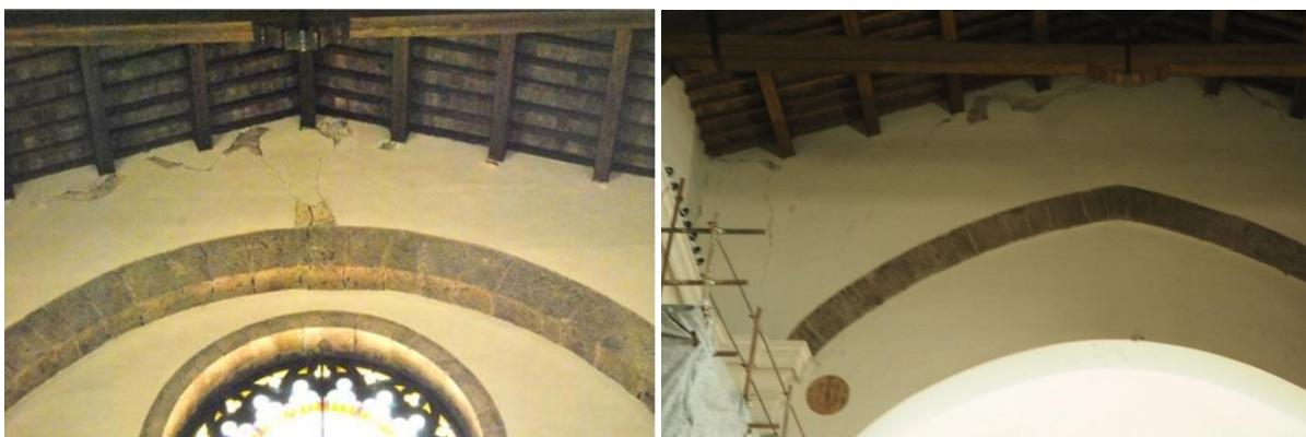
Figure 6-24 Cracks and initial pull-out of purlins a) on the front façade and b) above the chancel arch
