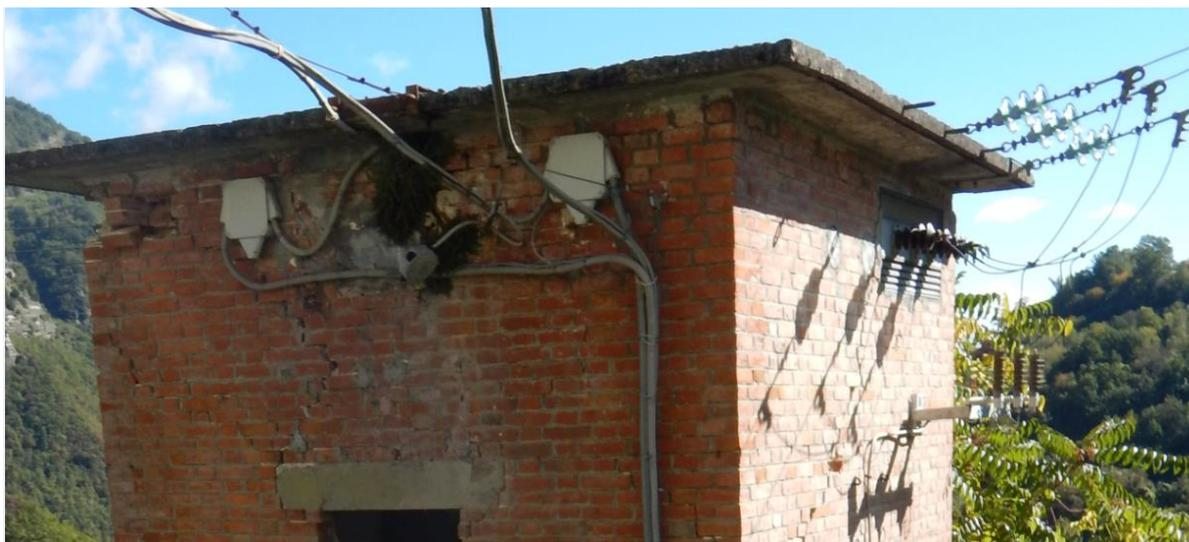
Figure 7-61 Arquata del Tronto – Electricity Transformer (lat.  $42^{\circ}46'21.912''\text{N}$ ; long.  $13^{\circ}17'50.022''\text{E}$ ), zoom of damage at the roof level.
