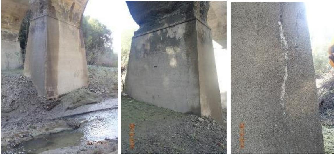
Figure 8-14 Images highlighting foundation scour (left) and vertical cracks in the bridge piers.
