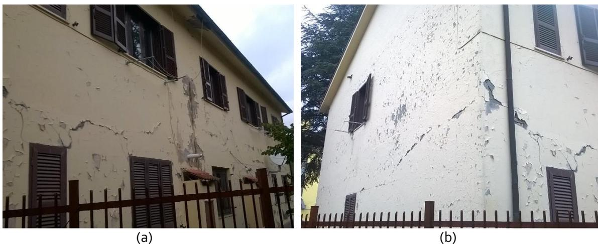
Figure 7-58 Amatrice Corpo Forestale (lat. 42°37'34.33"N long. 13°17'31.24"E) damage observed, widespread cracking to (a) East and (b) North facades.
