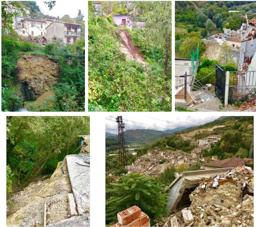
Figure 4-21 Observed slides in the locality of Pescara del Tronto and related induced-damage.
