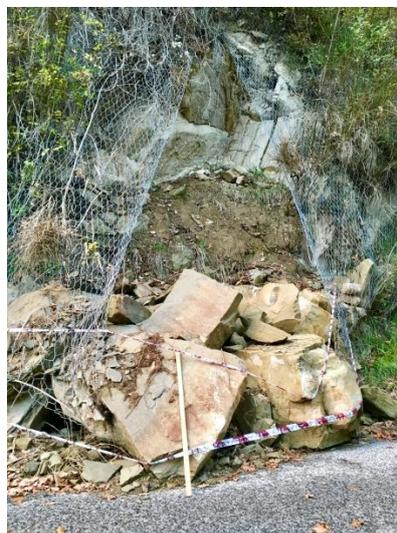
Figure 4-14: Rock slide along the main access road to Accumoli, where boulders detached from the bedrock and punched through the wire mesh.
