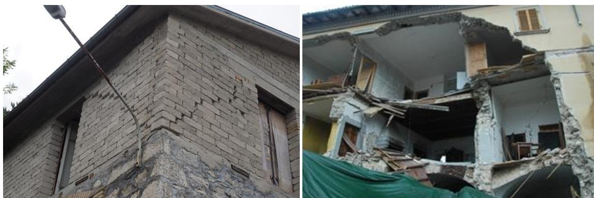
Figure 5-5: a) Shear crack of corner in building with second floor addition in concrete blocks and ring beams; b) out of plane failure of façade wall of 3 storey high building with traditional vaulted structures at ground storey, intermediate timber floors and RC roof slab. No evidence of ties.
