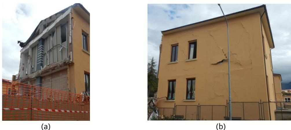
Figure 7-26 Amatrice School Capranica (lat. 42°37'38.10"N, long. 13°17'27.49"E), (a) evidence of the retrofitting intervention with FRP on columns of the RC part of the building; (b) evidence of cracked plaster from which the presence of fibres of reinforcement as prevented failure and produced a more widespread cracking.
