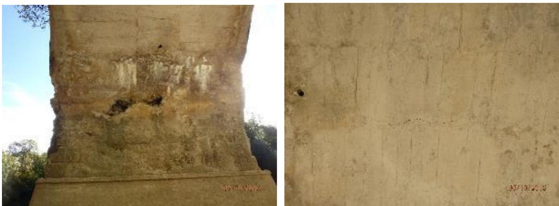
Figure 8-16 Localised ejection of material at the arch soffit (left), bridge arch longitudinal cracking (right)
