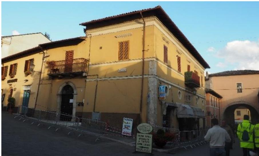
Figure 5-28 Residential building in Norcia, nearby Porta Romana. Note the buttresses, ties, and quoins, as prescribed in the 1859 decree. A diagonal airline crack is visible in the return wall.
