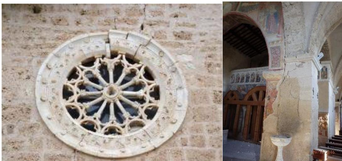
Figure 6-8 a) Diagonal crack through the rose window; b) Pillar split through vertical crack, and shear failure of the top part corresponding to the same damage observed in figure 6.7 for the screen wall.
