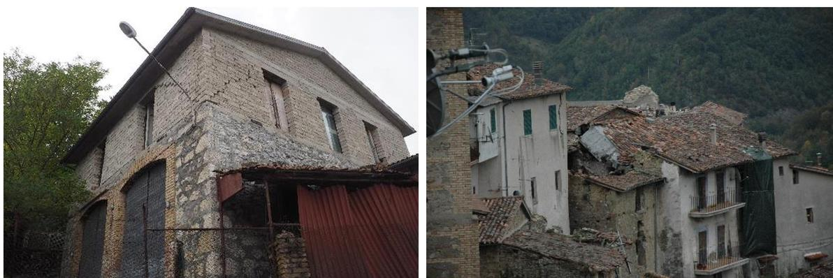
Figure 5-13 a) Corner expulsion in a building retrofitted with ring beam; b) Roof failures and vertical cracks in several poorly maintained buildings.
