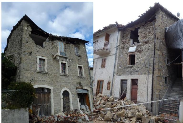
Figure 5-25: Typical structural damage recorded in Pescara del Tronto along the Salaria Road.
