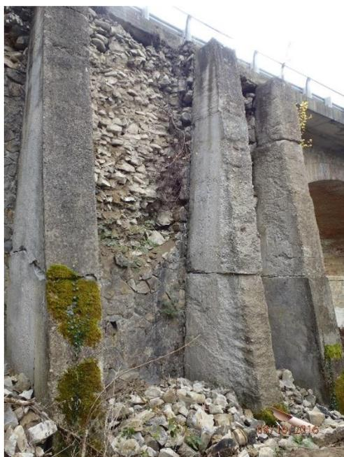
Figure 8-8 Gravity buttresses failure
