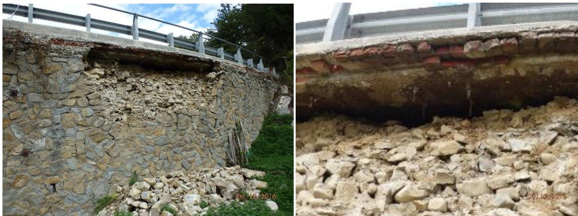
Figure 8-7 Failure of the East abutment southern wall; b) detail of the exposed deck slab connectors
