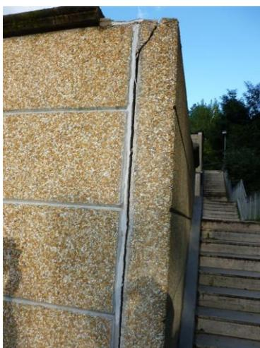
Figure 7-52 Norcia COC (lat.  $42^{\circ}47'43.89''\text{N}$ ; long.  $13^{\circ}5'29.26''\text{E}$ ). nonstructural damage to precast panel.
