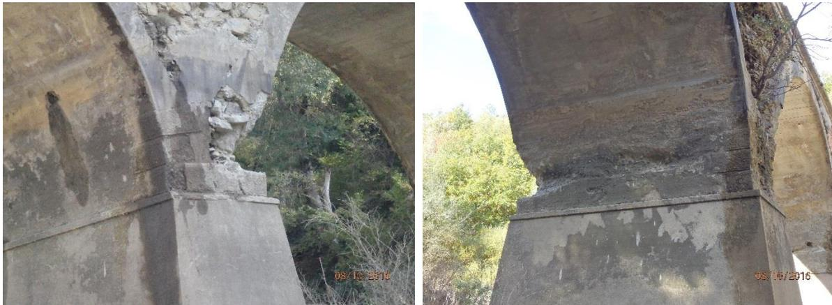
Figure 8-15 Hinges by the pier springers
