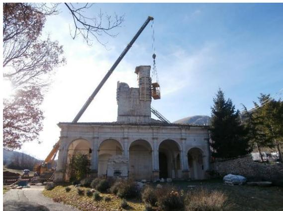
Figure 6-14 a) Front elevation after the 26th October shocks (image from <http://www.umbria24.it>); b) Front elevation in December 2016. Note damage to the bell piece laying on the front yard.
