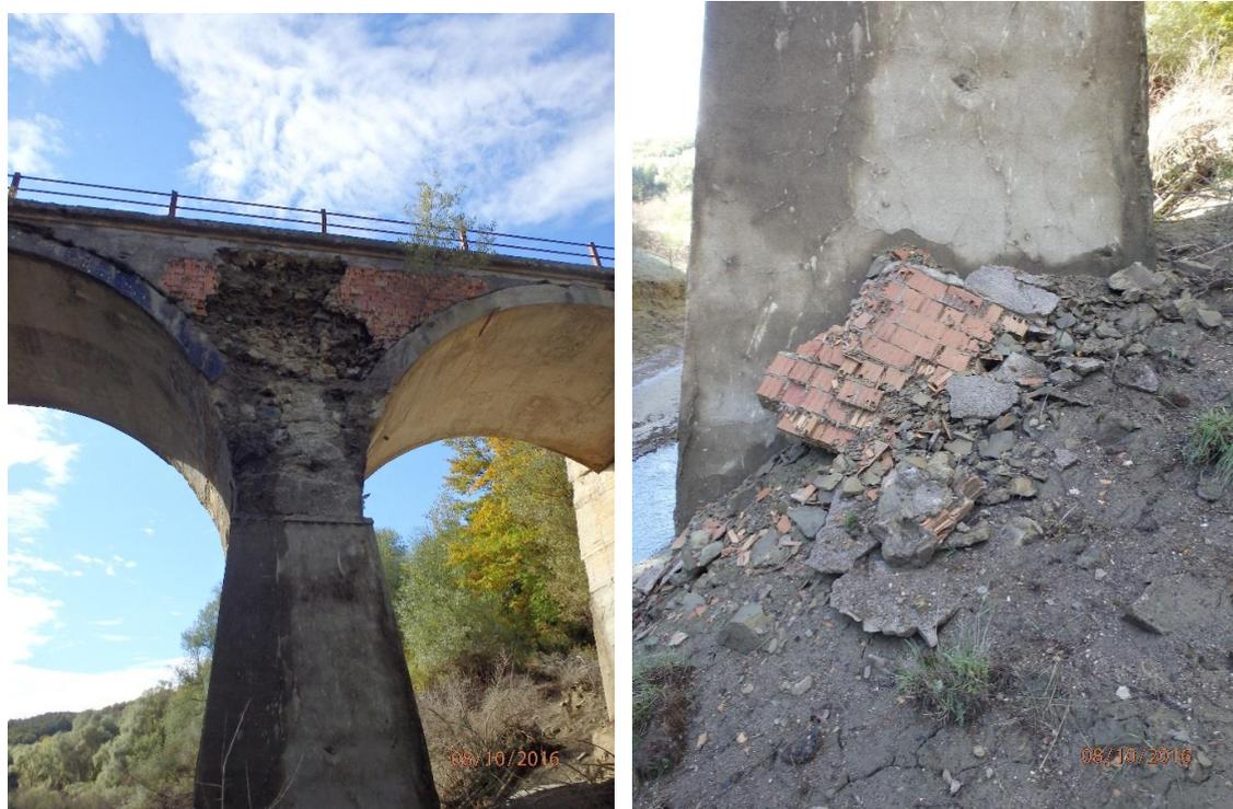
Figure 8-17 Spandrel masking walls failure
