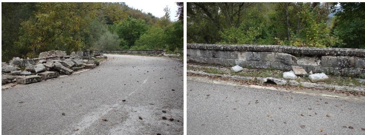
Figure 8-23 Collapse (left) and damage (right) of the masonry parapets.
