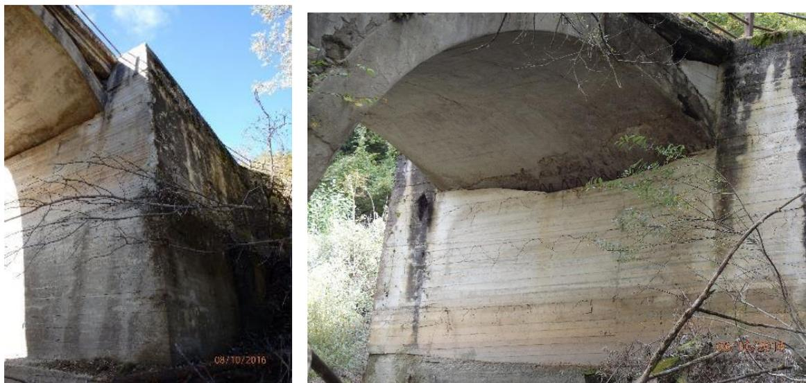
Figure 8-13 Images showing the RC abutment walls and arches concrete lining
