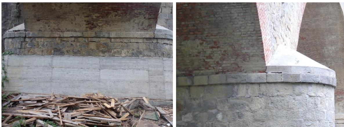
Figure 8-11 Horizontal cracks at pier heads
