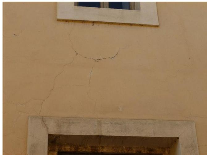
Figure 7-50 Norcia Caserma (lat. 42°47'41.37"N; long. 13° 5'31.19"E). Cracking between windows
