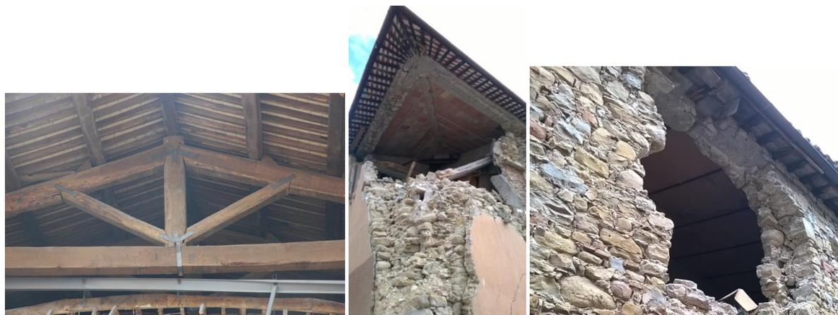
Figure 5-4: Examples of (a) traditional wooden roof structure; (b) concrete roof with lightweight brick tiles; (c) steel beam profile roof on mixed masonry -concrete ring beam.
