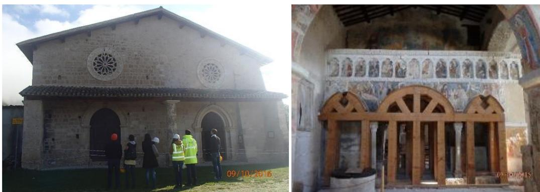
Figure 6-6 a) Front view of the S. Salvatore Church in Campi; b) The screen supported by a timber shoring system in the northern nave
