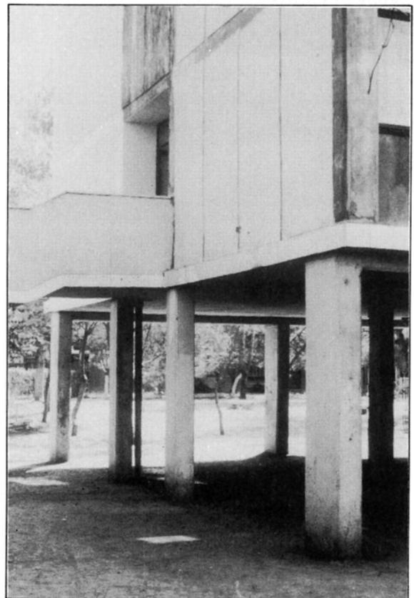
PLATE 5.17 Undamaged block at Villa Olympia
