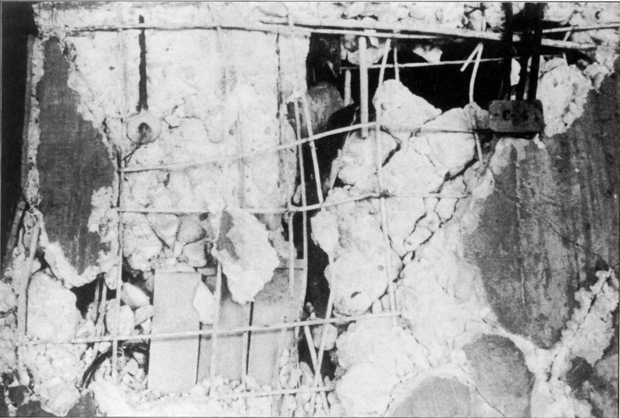
PLATE 5.20 Damage to internal shear wall in Villa Portales (location X, PLATE 5.18)
