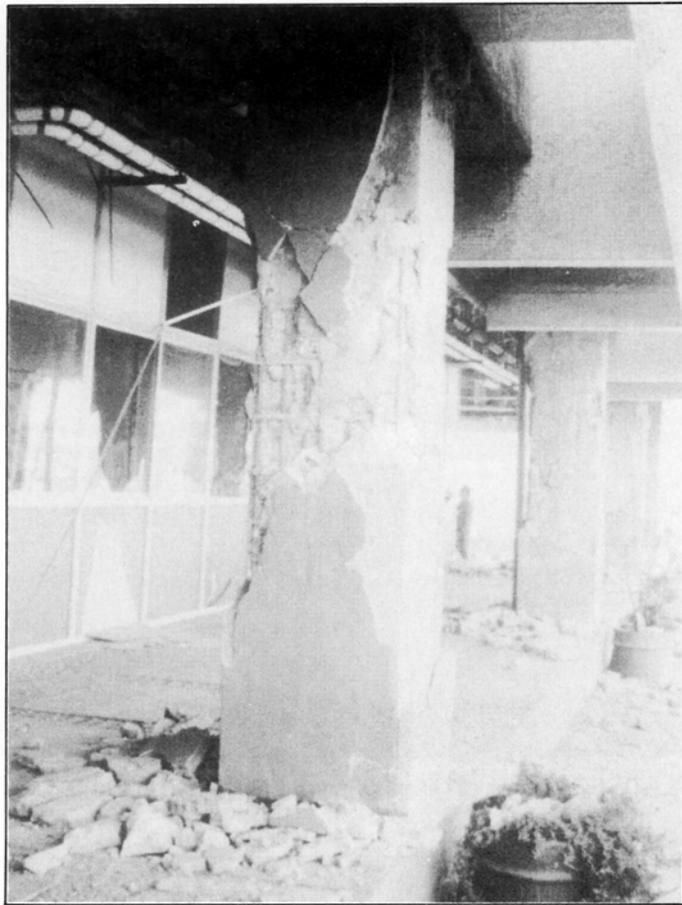
PLATE 5.1 Compression failure in external columns
