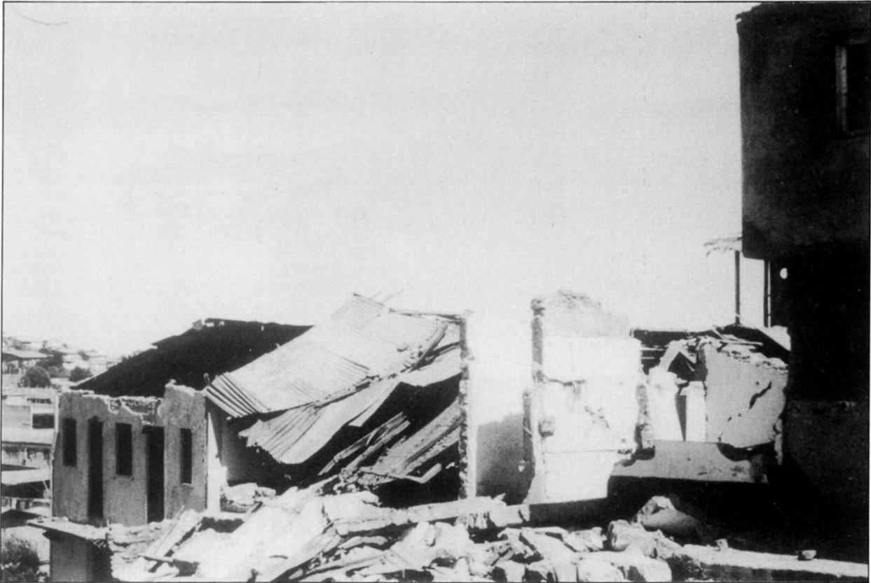
PLATE 5.24(a) Heavily damaged masonry houses
