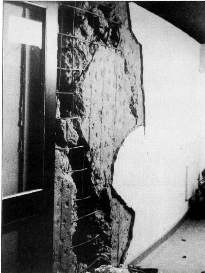
PLATE 5.8 Major vertical crack in Hangaroa apartments
