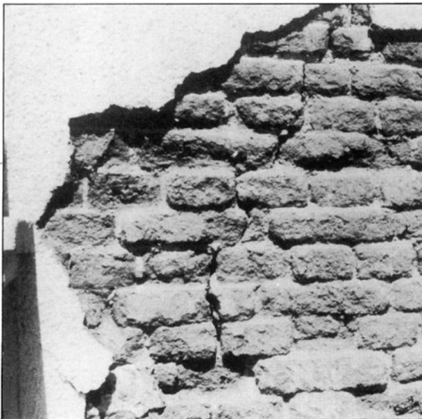
PLATE 5.28(b) Detail of cracked adobe bricks
