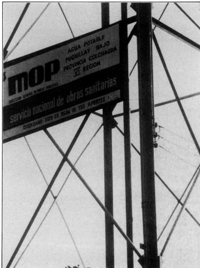
PLATE 5.36(b) Detail of buckled braces
