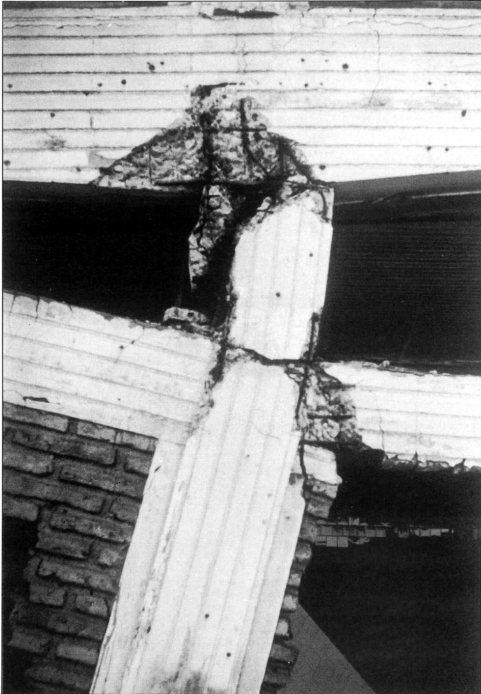
PLATE 5.44 Damaged to rc frame building due to lateral spread of quay, San Antonio Docks [see PLATE 5.42 (a)]
