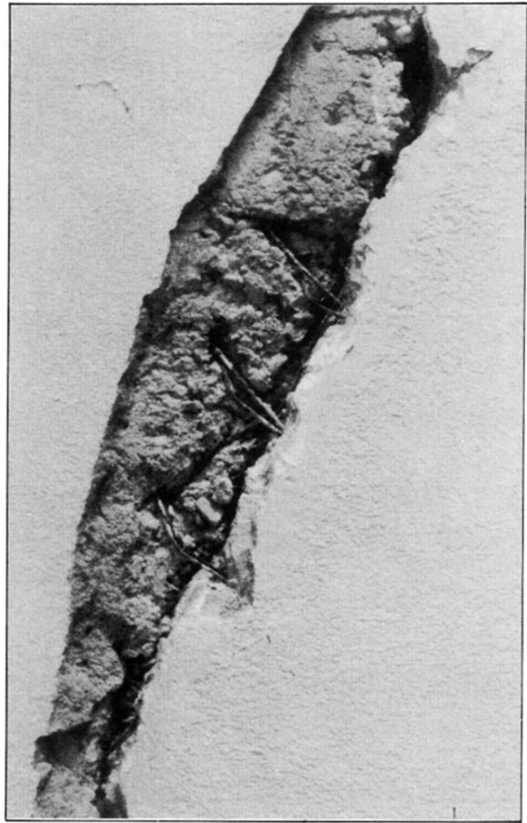
PLATE 5.9 Patch repair to previous earthquake damage, Acapulco apartments, Viña del Mar
