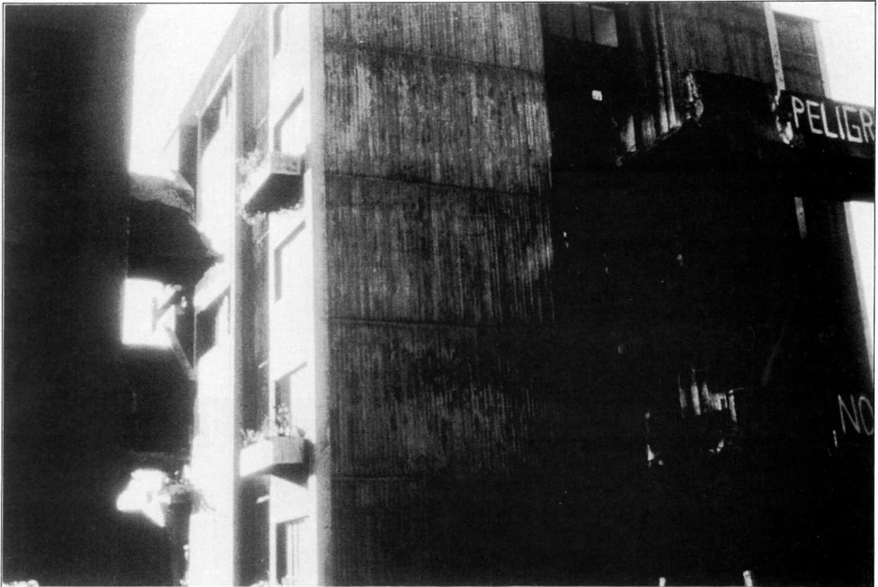
PLATE 5.15 Damaged bridge links in Viña del Mar building
