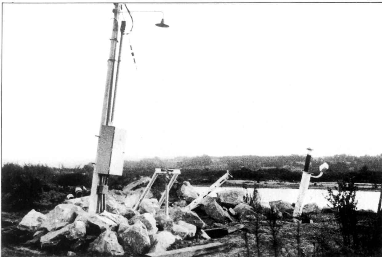
PLATE 5.45(a) Failed well point
