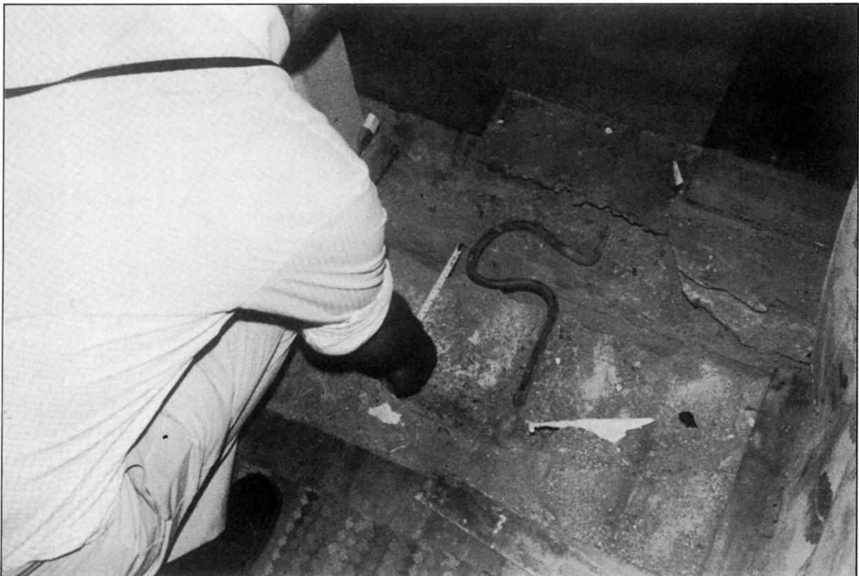
PLATE 5.22 Expansion loop in water pipe crossing expansion joint, Villa Portales, Santiago
