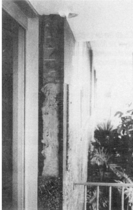
PLATES 5.52 and 5.53 *Loss of cladding and cracking of masonry in-fill in a modern office building in King Street, Newcastle (location 19)*
