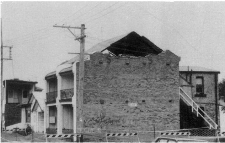
*PLATE 5.5 Gable end wall collapse in residential two storey brick masonry building (location 11)*
