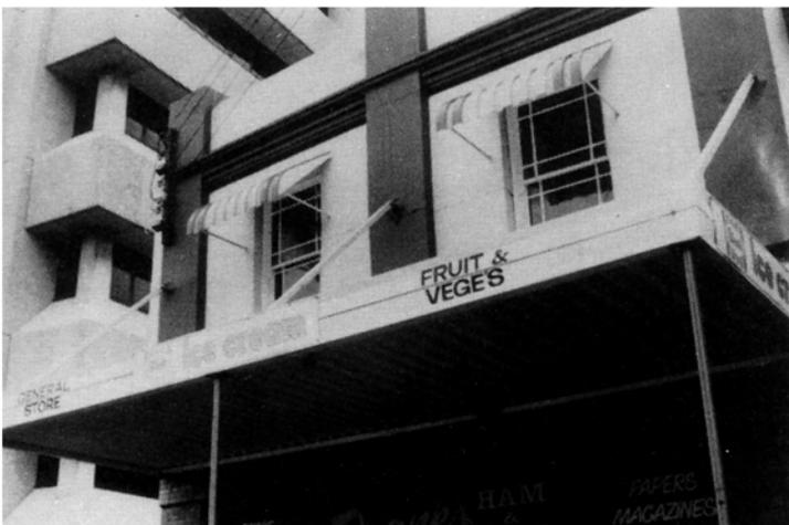
PLATE 5.35 *Cracking of facade near tie-back positions for suspended awning*
