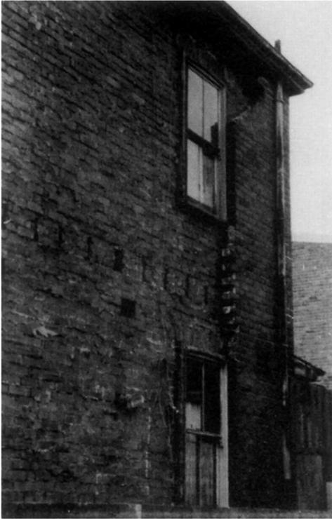
PLATE 5.1 *Collapse of outer skin of cavity unreinforced brick masonry wall (location 18)*
