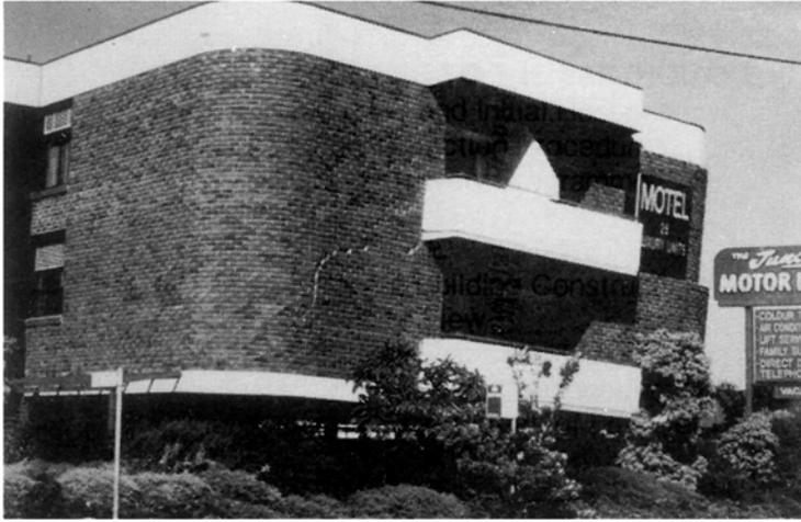
PLATES 5.63 and 5.64 *The combination of a soft first storey and a highly asymmetric stiffness layout led to shear failure and crushing at the top of a row of exterior reinforced concrete columns at the Junction Motel. This building was demolished immediately after the earthquake (location 39)*
