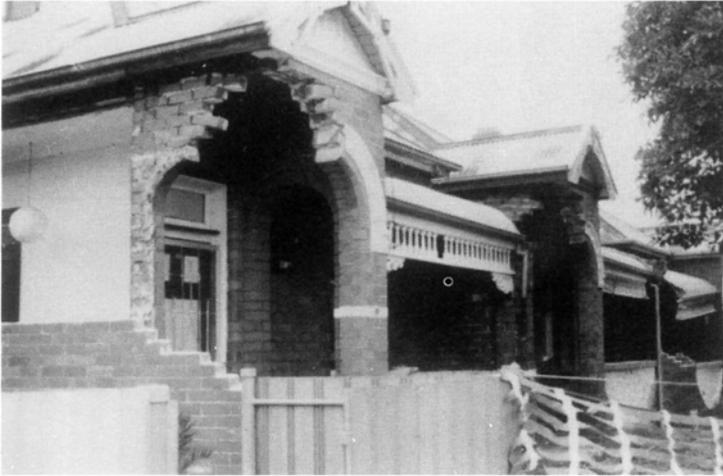
PLATE 5.9 *Damage to exterior ornamental brick columns and arches (location 8)*
