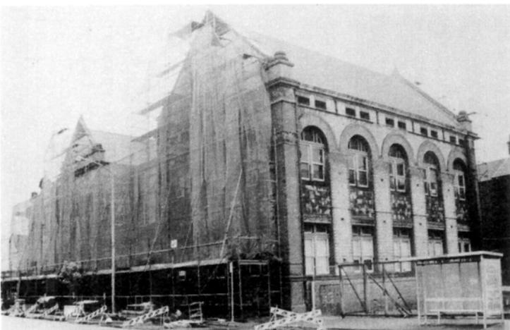
PLATE 5.41 *Extensive cracking was observed in the facade of this brick masonry college building in the Newcastle central business district (location 17)*
