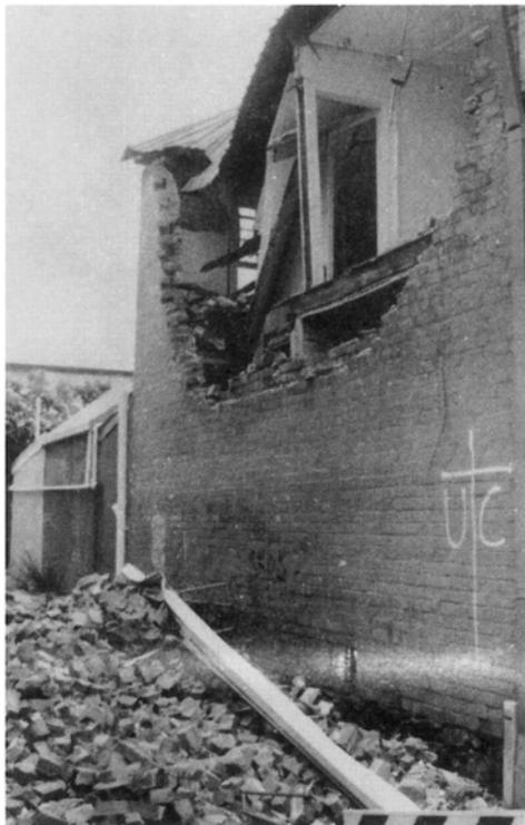
PLATE 5.3 *Collapse above first floor level of solid double unreinforced brick masonry wall (location 25)*
