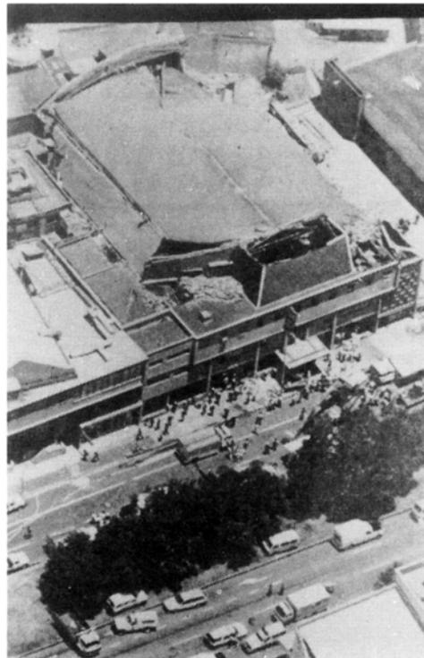
PLATES 5.61 and 5.62 *Extensive structural damage and collapse at the Newcastle Working Mens' Club, where nine persons died in the earthquake (location 20)*
