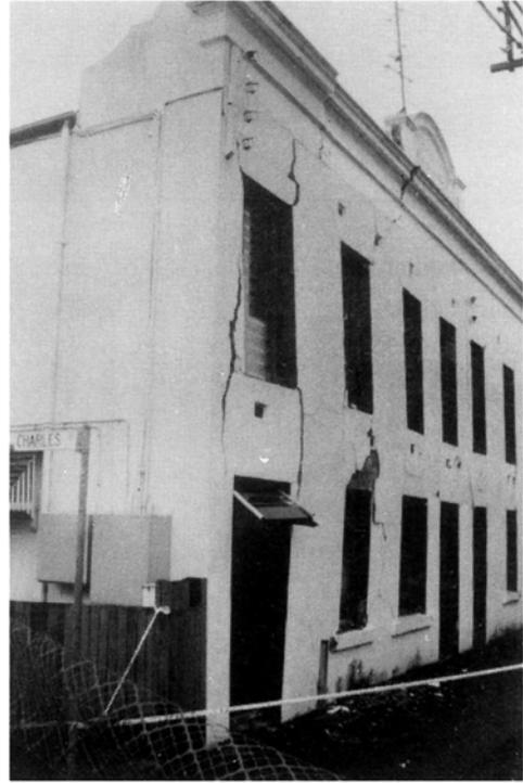
PLATES 5.12 and 5.13 *Cracking and leaning of parapets and facades in an older two storey brick masonry building (location 24)*
