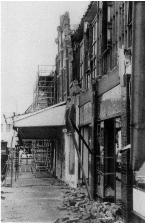
PLATE 5.33 *Collapsed second storey brick masonry facade in two storey commercial building. The remaining facade is leaning dangerously away from the building (location 21)*
