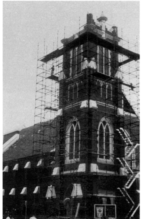
PLATES 5.67 and 5.68 *Partial collapse and severe cracking of masonry spire and tower, a common form of damage to churches in Newcastle (locations 26 and 7)*
