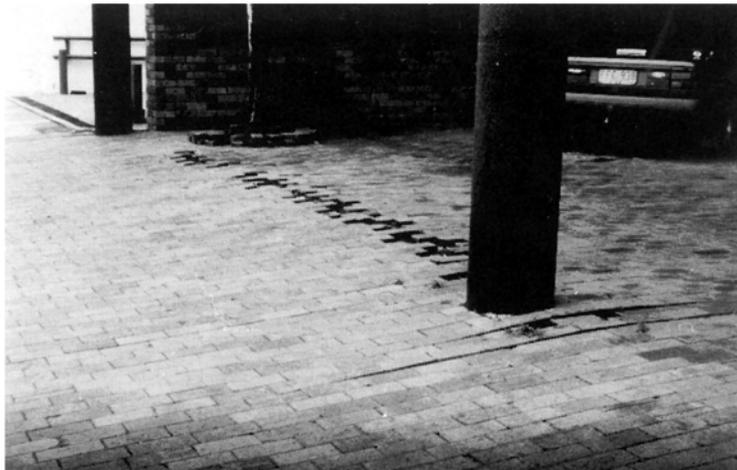
*PLATE 5.78 Evidence of localised ground compression causing bulging of brick paving (location 14)*
