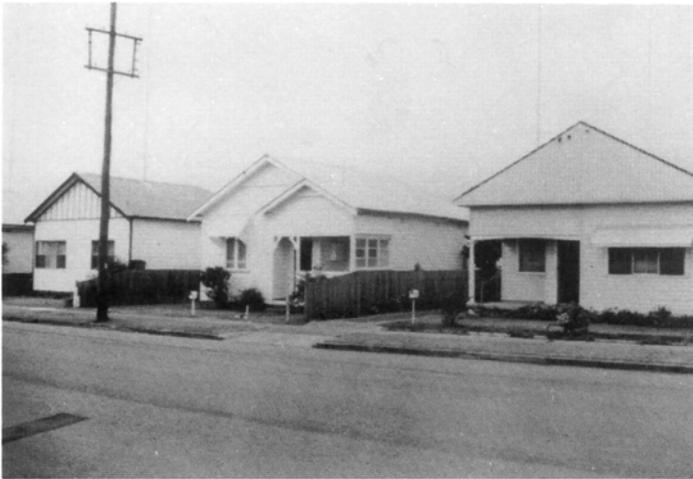
PLATE 5.70 *Typical single storey timber framed weatherboarded dwellings, which suffered only minor damage in the earthquake*
