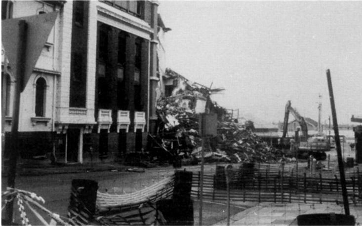
PLATE 7.1 *The George Hotel in the Newcastle central business district, a five-storey unreinforced brick masonry building which had to be demolished nine days after the earthquake (location 34)*
