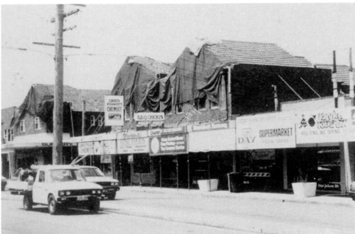
PLATE 5.38 *Gable end failures in a group of modern two storey commercial brick masonry buildings (location 2)*
