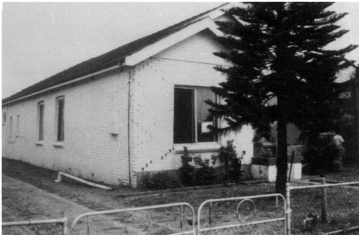
*PLATE 5.7 Diagonal shear cracking near corners of brick masonry dwelling (location 4)*
