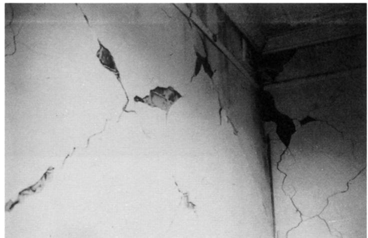
*PLATE 5.8 Cracking of internal load-bearing walling in single-storey brick*
