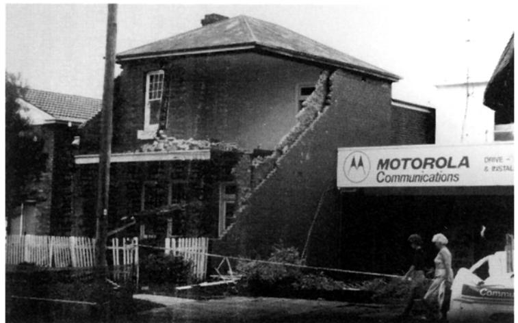
PLATE 5.4 *Front and side wall collapse in modern unreinforced brick masonry two storey dwelling (location 12)*
