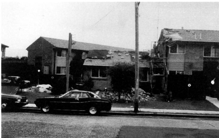
PLATE 5.11 *Secondary damage to roofing due to chimney and side wall collapse in an adjacent building (location 37)*
