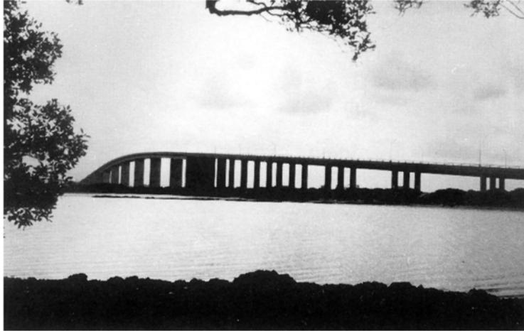
*PLATE 5.77 General view of the Stockton Bridge, north of Newcastle which showed slight settlement of the western abutment due to the earthquake (location 1)*
