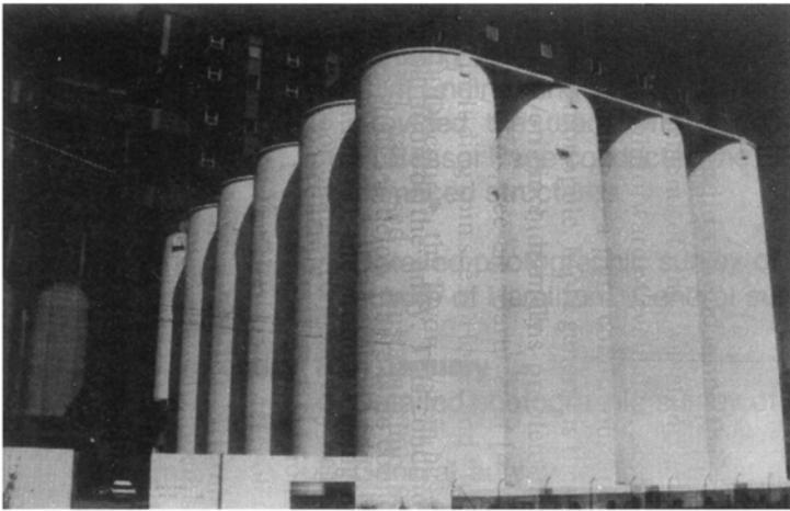
PLATES 5.74 and 5.75 *Minor spalling of concrete in storage silos was the only evident form of damage to industrial facilities in Newcastle (location 16)*
