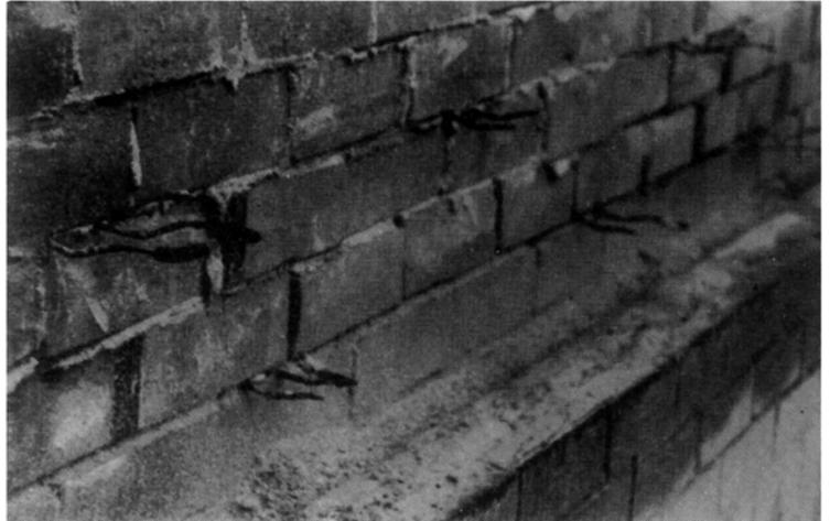
PLATE 5.2 *Corroded ties in cavity brick masonry wall construction (location 18)*
