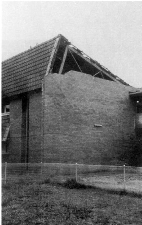
PLATE 5.44 *Brick masonry parapet collapse at the Tighes Hill Technical College, Newcastle (location 6)*
