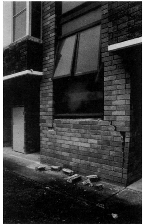
PLATES 5.16 and 5.17 *Severe cracking in unreinforced brickwork near corners, doors and window openings at first storey level of the building shown in PLATES 5.14 and 5.15*
