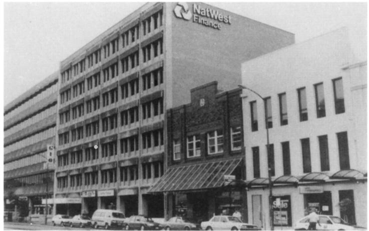
PLATES 5.57 and 5.58 *There was no recorded earthquake damage to these two modern multi-storey reinforced concrete frame and frame-shear wall buildings in the Newcastle central business district (locations 28 and 14)*
