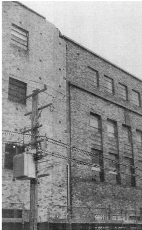
PLATE 5.51 *Partial collapse of parapet in the steel-framed Hamilton Telephone Exchange building (location 9)*
