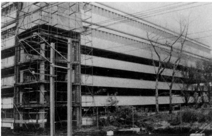
PLATE 5.56 *Total collapse of the lower five storeys of unreinforced brick masonry walling attached to reinforced concrete frame car park and office building (location 29)*
