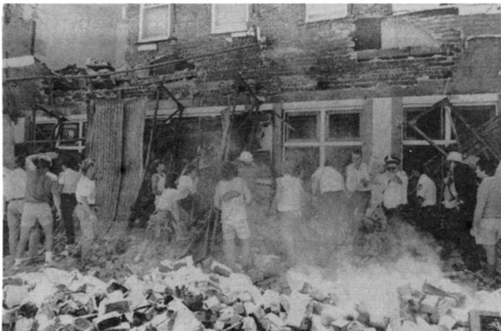
PLATE 5.20 *Rescue operations and emergency strengthening of a partially collapsed two storey brick masonry building in Beaumont Street, Hamilton*
