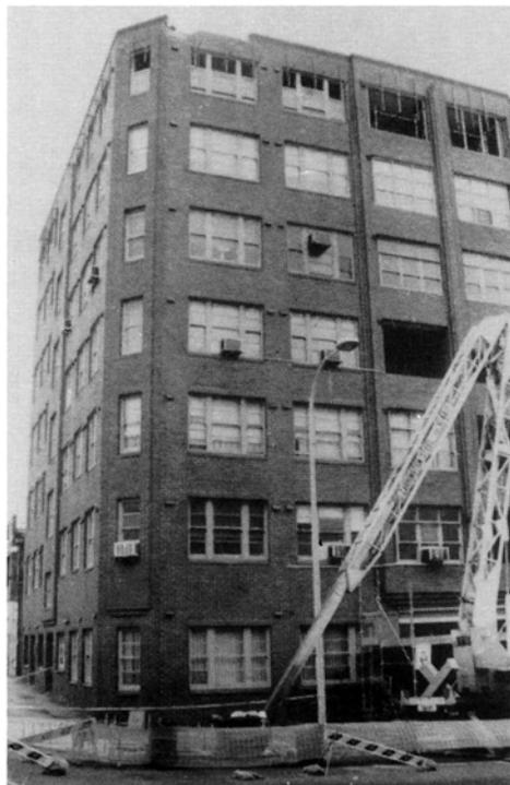
*PLATE 5.50 Parapet failure in a brick clad, seven storey steel framed office building in the Newcastle central business district (location 34)*
