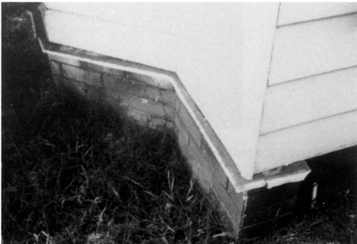
PLATE 5.71 *Sliding movement between timber structure and its support foundations (location 5)*
