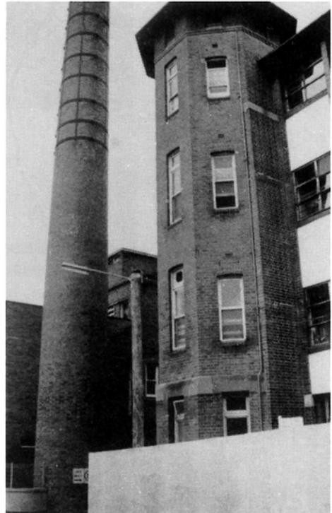
*PLATE 5.49 The 30m high brick chimney at the Royal Newcastle Hospital showed no signs of earthquake damage*
