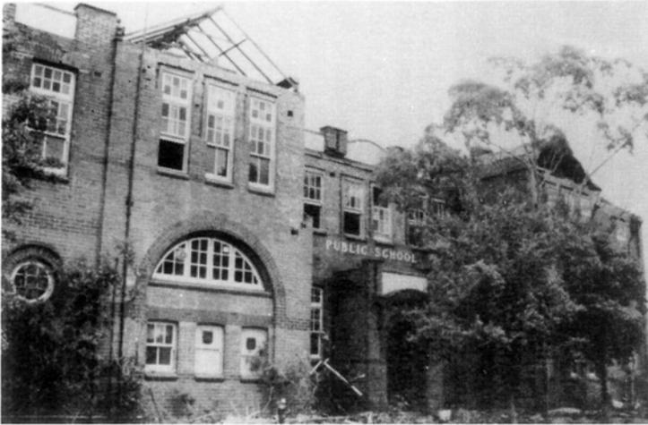
PLATES 5.39 and 5.40 *Extensive damage to roof, parapets and gable ends in a 100 year old school in The Junction, Newcastle (location 38)*
