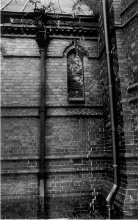
PLATE 5.66 *Vertical crack in the outer wall of the Newcastle Christ Church Cathedral, reportedly dating from the earthquake in 1925 (location 32)*
