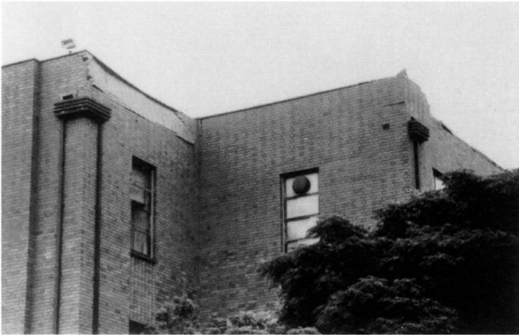
*PLATE 5.45 Damage to brick masonry cladding at the Tighes Hill Technical College, Newcastle (location 6)*
