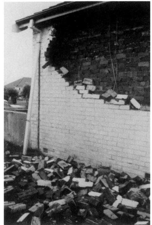
*PLATE 5.6 Outer skin cavity wall failure in older residential brick masonry building (location 4)*
