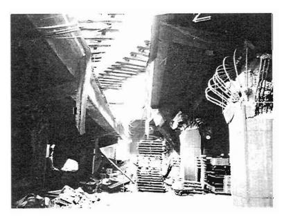
Plate 4.161: Collapsed infill slab due to buffeting between viaduct and warehouse
