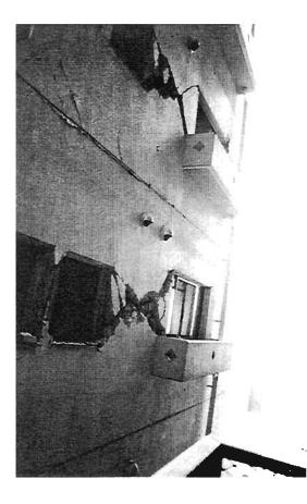
Plate 4.54: X-cracking in perforated shear walls
