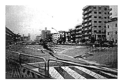
Plate 8.33: Collapse of the Daikai Station
