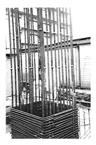
Plate 4.168: Column reinforcement in modern RC construction
