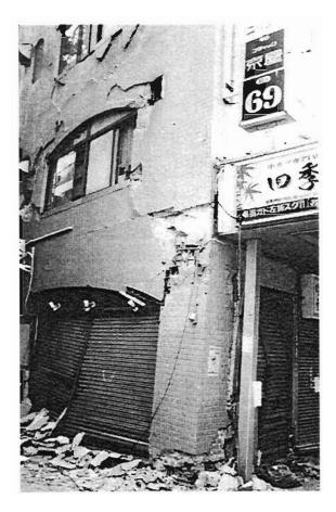
Plate 4.45: Corner joint damage in irregular building
