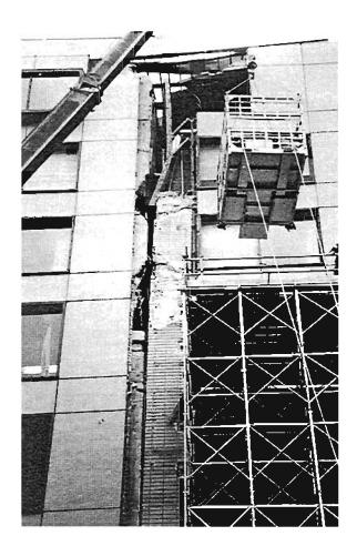
Plate 4.157: Buffetting damage in top storey
