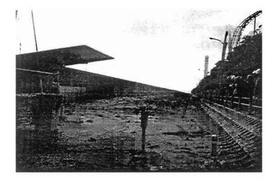
Plate 8.13: Erupted sand deposits found at the boundary between Phase 1 and 2 sections of Port Island
