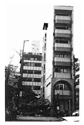
Plate 4.81: High aspect ratio building with cold formed RHS columns
