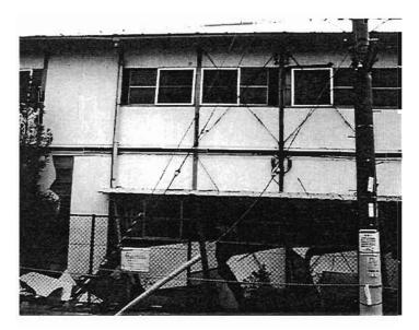
Plate 4.103: Prefabricated building with wire bracing
