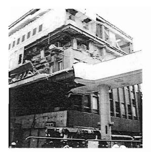
Plate 4.89: SRC building damaged by link bridge
