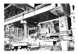
Plate 6.58 Railway near Centre of Kobe -Damage to Steel Portal Pier centrifugally cast columns lacked ductility
