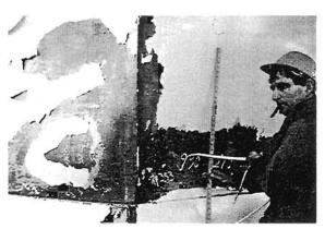
Plate 6.50 Hanshin Expressway - Damage to Circular Steel Pier Column freshly flaked paint on column near Kobe centre indicates strong north-south cyclic action Plate 6.49 Hanshin Expressway - Damage to Rectangular Steel Pier Column extent of buckle indicated by Dr Peter Merriman
