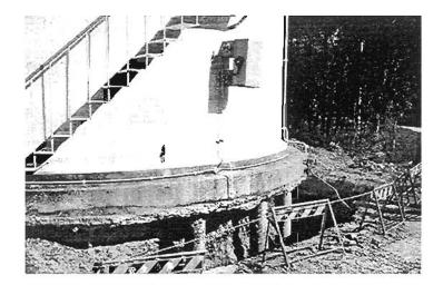
Plate 8.22: Excavated piles under a water tank at the Higashinada Power Station (Photo by C. Bolton)
