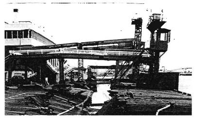
Plate 7.38 Settlement damage to ferry terminal
