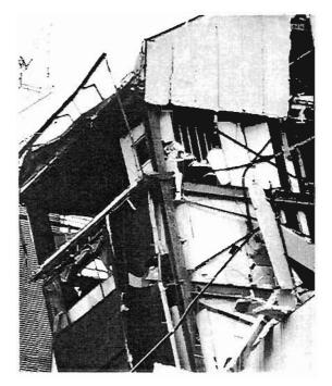
Plate 4.69: Snapped bracing
