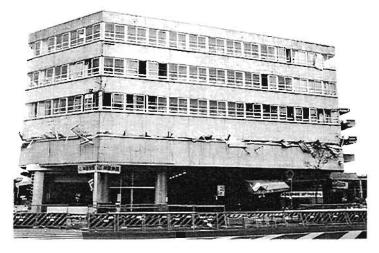
Plate 4.16: 1st Storey collapse due to change in column shape
