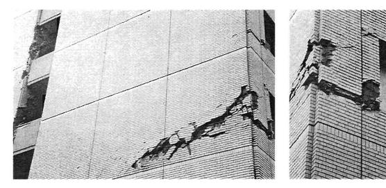
Plate 4.28: Flexural/shear failure in shear wall building
