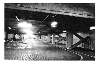
Plate 4.132: Internal bracing of the Diamaru
