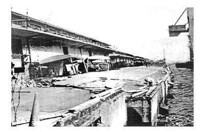
Plate 8.16: Lateral movement of concrete caisson walls at the Shinko Pier in Port Kobe
