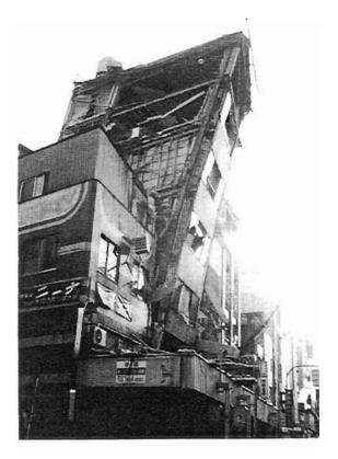
Plate 4.68: Sway after snapping of bracing flats in upper stories
