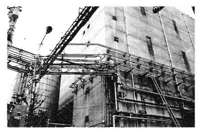
Plate 7.22 Pipework on wall of brewery
