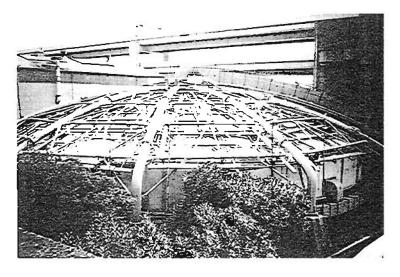
Plate 7.14 Glassfibre panel roof, with temporary supports
