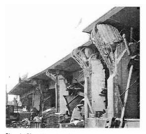
Plate 4.176: Differential drifts between transverse joints
