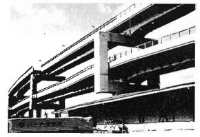
Plate 6.17 Route 2 near downtown Kobe:Large transverse displacement of deck at movement joint supported on cantilever from portal pier
