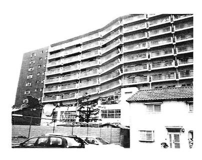
Plate 4.21: Partial storey collapse due to shear wall failure one end of building
