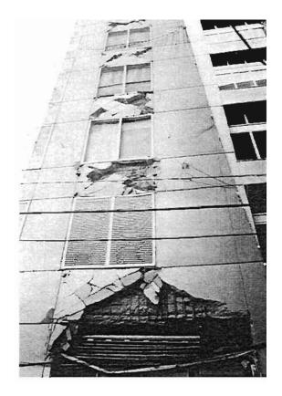
Plate 4.36: Damaged connection beams
