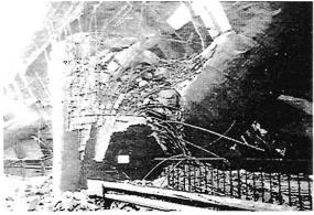
Plate 6.25 Hanshin Expressway, Kobe Route 3, Fukae-Honcho Section close-up of pier in foreground of Plate 6.22 showing small lateral bars and curtailed longitudinal bars.
