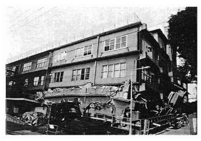
Plate 4.110: Precast concrete building with partial collapse induced by link bridge
