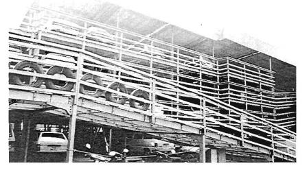
Plate 4.135: Undamaged flimsy and flexible car park
