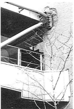
Plate 4.145: Connection damage between new buildings
