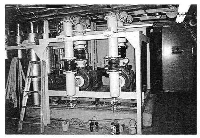
Plate 7.25 Pumps in basement; well anchored
