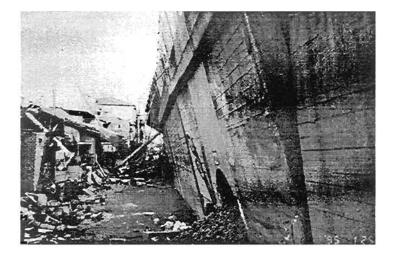
Plate 8.34: Tilt of a concrete gravity retaining wall (photo by Prof. J. Koseki)
