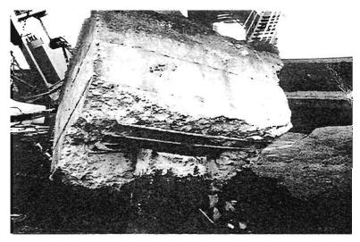
Plate 7.10 Steel pile unconnected to foundation
