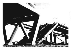
**Plate 6.5** Nishinomiya Harbour Bridge on the Hanshin Bay Expressway Approach span fell due to loss of support as main pier shifted towards main span.
