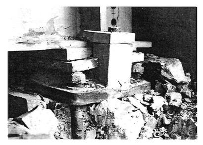
Plate 4.112: A garage base plate which performed well despite the failure of the supporting plinth
