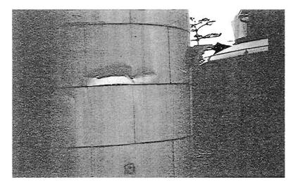
Plate 7.16 Buckling in tank wall
