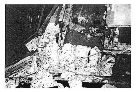
Plate 4.93: Column pulled out of plinth
