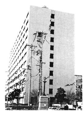
Plate 4.27: Coupled shear wall building
