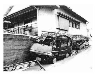
Plate 4.102: Collapse of steel frame building with soft storey
