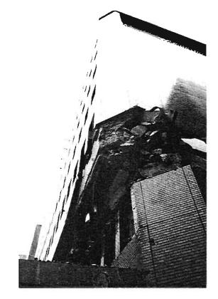
Plate 4.9: Streetwise displacement at adjacent corner
