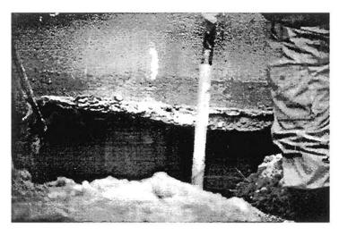
Plate 8.23: Hairline cracks observed in the piles of the water tank (photo by C. Bolton)
