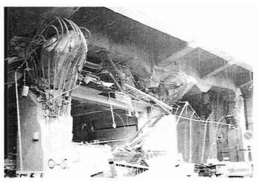
Plate 4.177: Incipient longitudinal hinge and more developed transverse hinges
