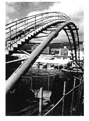
Plate 7.39 Arch pipebridge Intact despite support movement K Soga University of Cambridge
