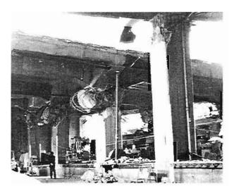
Plate 4.178: Incipient internal transverse hinge
