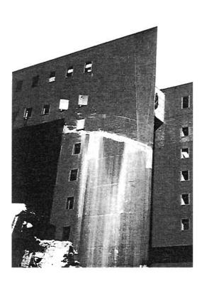
Plate 4.29: Substantial perforated shear wall building
