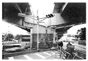
Plate 6.31 Hanshin Expressway, Kobe: Damage to large pier at level of construction joint and/or curtailment of reinforcement.
