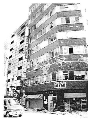
Plate 4.155: Collapse of 3<sup>rd</sup> storey of corner building due to buffeting
