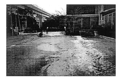
Plate 8.2: Liquefied sand deposits at a parking area at Minatojima, Port Island
