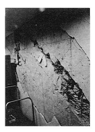
Plate 4.37: Shattered shear wall
