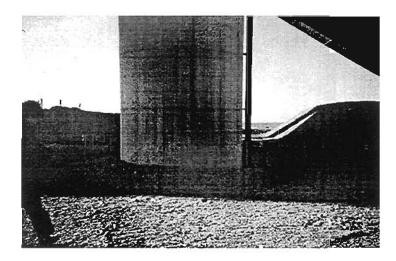
Plate 8.27: Lateral movement of the surface ground pushing the pier of the Nishinomiya Bridge
