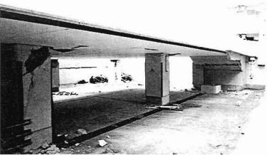
Plate 4.57: Anchorage of ramp to first floor
