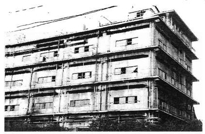
Plate 4.107: An undamaged clerestory windowed building on reclaimed land near the coastal highway
