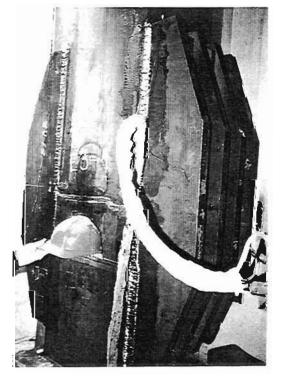
Plate 4.78: Fin strengthening at column fractures
