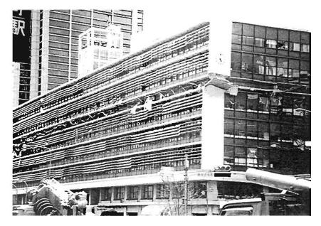
Plate 4.87: The old town ball with collapsed 6th storey
