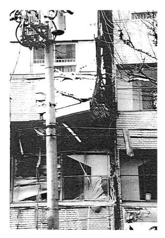
Plate 4.156: Column damage due to buffetting
