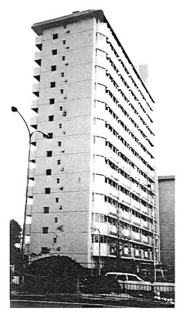
Plate 4.32: Shear wall compression failure with consequential shear fracture along vertical axis
