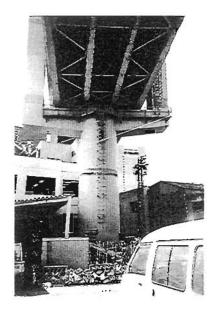
Plate 6.51 Hanshin Expressway Route 2 near the centre of Kobe- Damage to Circular Steel Pier Column viewed along the line of the structure shows a symmetric buckle at change in wall thickness
