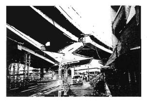
Plate 6.9 Hanshin Expressway to the west of Kobe centre:Large sideways shift towards south of curved deck, same interchange as Plate 6.8
