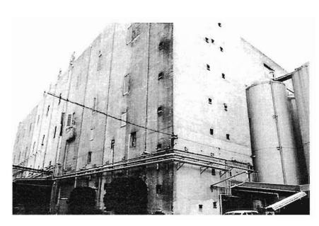
Plate 4.106: Unperforated shear wall of factory in port area
