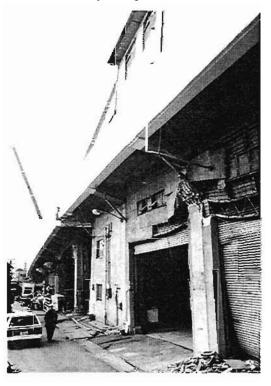
Plate 4.180: Incipient external transverse hinge
