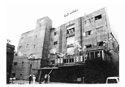
Plate 4.105: Mid-height failure of substantial irregular structure
