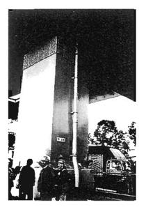
Plate 6.47 Hanshin Expressway - Damage to Rectangular Steel Pier Column stiffened walls buckled exposing orange coloured primer/undercoat
