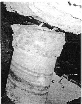
Plate 7.12 Poorly connected RC pile
