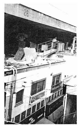
Plate 4.160: Damaged stub column under viaduct due to building restraint
