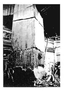
Plate 6.34 Hanshin Expressway, Kobe: Flexure/shear failure at laps in main bars - bond lost with cover concrete
