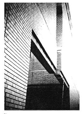
Plate 4.26: Relative displacement between buildings
