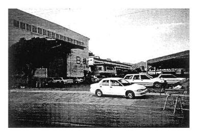
Plate 8.32: Less liquefaction settlement found at an improved ground site on Port Island (The foreground is an untreated site, whereas the background behind the car is a treated site)
