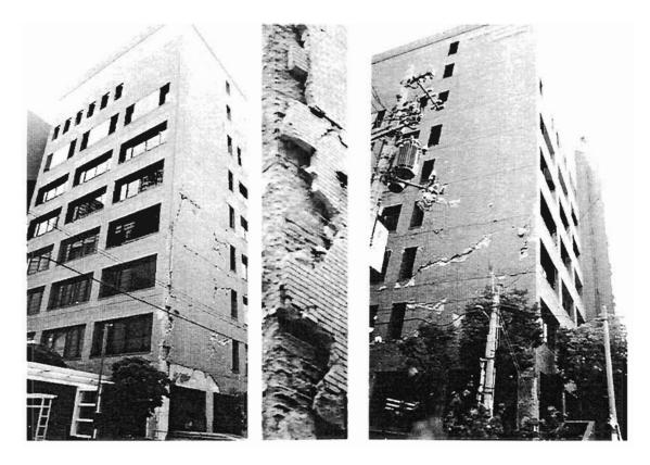
Plate 4.22: Spalling attributable to lack of longitudinal shear walls
