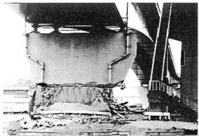
Plate 6.40 East Bank at the Maya Ohashi Bridge on the Harbour Highway liquefaction caused extensive lateral spreading
