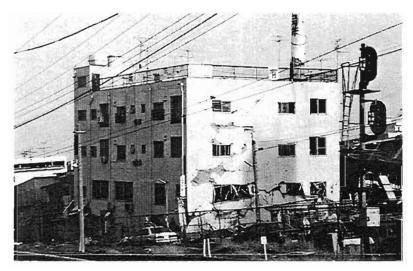
Plate 4.109: Local failure at long 1st floor window of building recessed into sloping site
