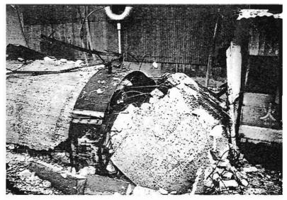
Plate 7.34 Fallen section of RC stack
