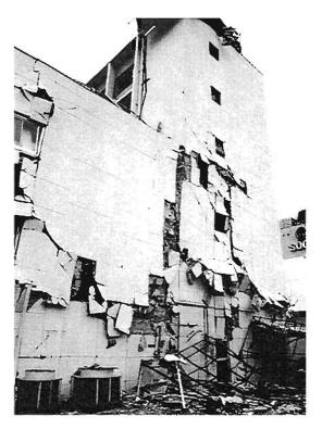
Plate 4.40: Damage at root of tower
