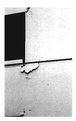
Plate 4.123: Cracking at ends of connecting
