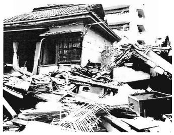
Plate 4.100: Severe cracking in masonry due to heavy roofs
