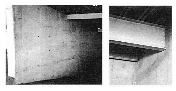
Plate 4.128: Repaired cracks in transverse wall
