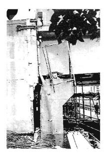
Plate 6.63 Footbridge over Canal, Kobe lateral spreading caused banks to move inwards, and girder sliced through roadway
