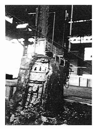
Plate 4.175: As 4.174 but severely corroded
