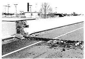
Plate 6.23 Ramp onto Hanshin Expressway near centre of Kobe: Hammering at joint has damaged deck joint and parapets
