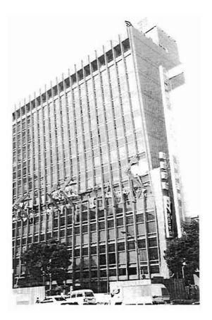
Plate 4.10: Streetwise tilt of 12 storey frame/shear wall structure
