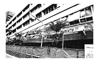
Plate 4.17: 2nd & 3rd Storey collapse in long building
