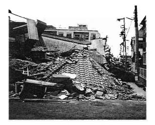
Plate 4.99: Collapse with roof intact
