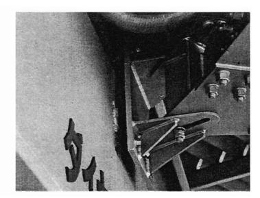
Plate 4.143: Failed top-beam connection
