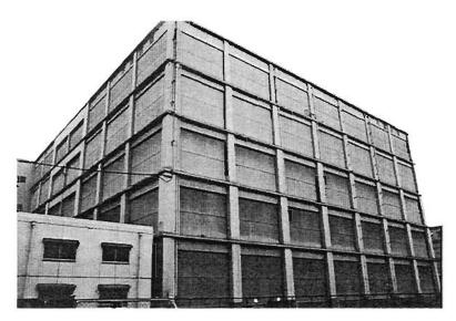
Plate 4.117: Undamaged Japanese framed-wall building
