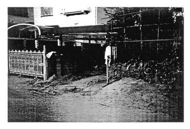
Plate 8.30: No apparent damage to the foundation of a bouse even large amount of erupted sands
