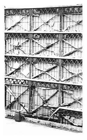
Plate 4.73: In-plane buckling of bracing
