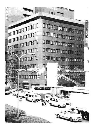
Plate 4.7: RC Building with collapse in 3rd storey
