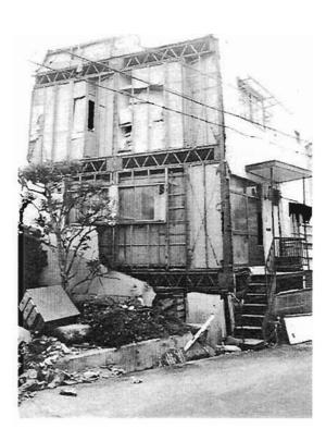
Plate 4.101: Wire bracing in tall panels
