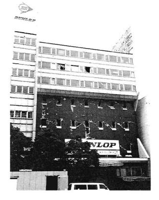
Plate 4.30: Distributed inelasticity in shear wall structure
