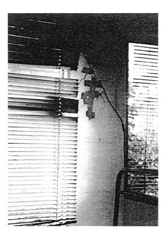
Plate 4.3: Internal RC column damage
