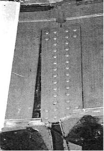
Plate 4.95: Rotated joint with rotation concentrated at span connection
