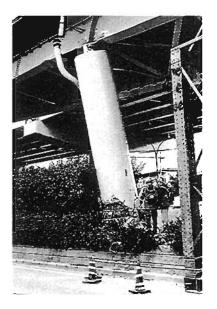
Plate 6.28 Ramp onto Hanshin Expressway, Kobe: Base of column in Plate 6.27: simple and almost non-existent laps offered no confinement. Failure is at location of curtailment of inner main bars.
