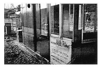
Plate 8.14: A dried water splash marker of liquified soils found at the toll gate box on Port Island
