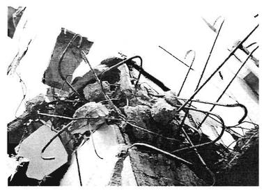
Plate 4.41: Disintegrated corner with reinforced fascia panels
