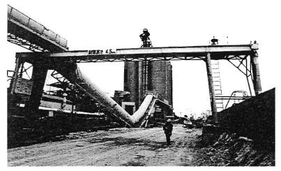
Plate 7.37 Collapsed section of conveyor
