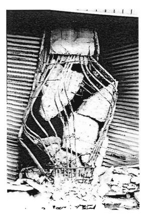
Plate 4.47: Failed off-centre central column
