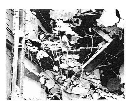
Plate 4.75: Building with failed welds at beam/column connections
