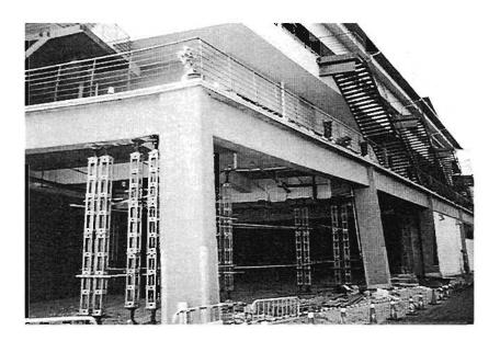
Plate 4.94: Damage attributable to lack of foundation tie beams
