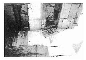
Plate 6.19 Shinkansen Bullet Train Line, Nishinomiya: Retrofit steel fabrication intended to provide lateral restraint to deck had been twisted out of position.
