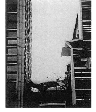
Plate 4.88: Collapsed and surviving link bridges
