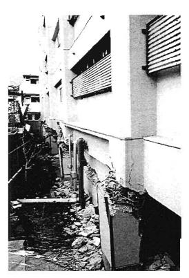
Plate 4.58: Severed shear wall
