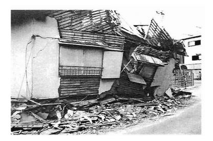
Plate 4.96: Collapsed timber-framed houses
