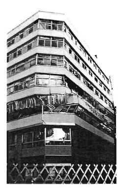
Plate 4.13: 2nd Storey collapse in 7 storey corner building
