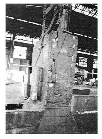
Plate 4.174: Cracked encased base of lattice column
