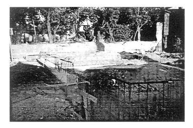
Plate 8.31: A house foundation with reinforcements found in Nishinomiya
