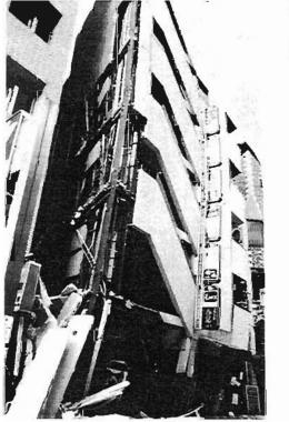
Plate 4.70: Sway after apparent failure
