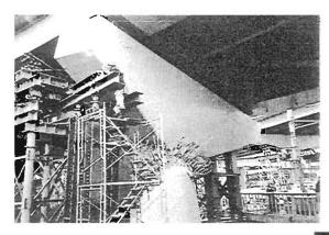
Plate 6.35 Hanshin Expressway to the west of Kobe centre: Shear-flexure failure at underside of column crosshead - lack of confinement
