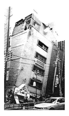
Plate 4.31: Rigid body rotation in one-sided collapse
