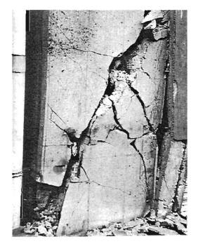
Plate 4,183: Incipient shear failure
