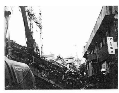
Plate 4.159: Collapse of viaduct span due to building restraint
