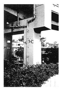
Plate 6.53 Hanshin Expressway Route 2 near the centre of Kobe- Damage to Rectangular Steel Pier Column change in wall thickness is likely to explain location of buckle in this stiffened box column
