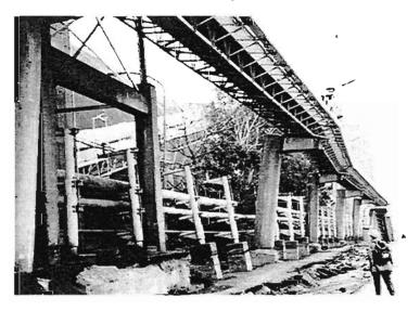
Plate 7.36 Overhead Conveyor with ground settlement
