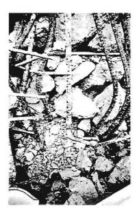
Plate 6.42 Pier on East Approach to the Maya Ohashi Bridge on the Harbour Highway damage at one corner of the pier in Plate 6.41 - note the failure of the welded bar in the centre of the Plate
