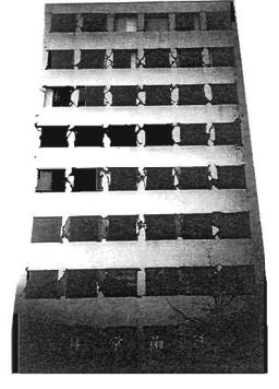
Plate 4.4: Distributed RC multion damage due to minimal damage in corner multions
