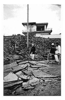
Plate 3.4: Pavement rupture due to the movement of the Nojima fault at Okura, Awaji Island
