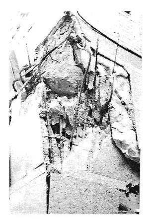
Plate 4.49: Exploded corner column joint
