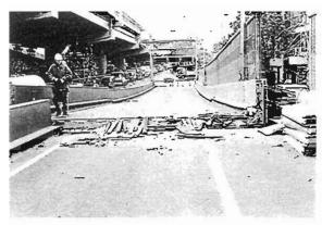
Plate 6.11 Ramp onto Hanshin Expressway near centre of Kobe: Approximate one metre shift of first ramp span towards the north
