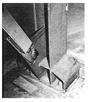
Plate 4.136: Column base/brace connection
