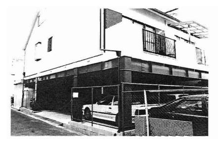
Plate 4.104: House with ground floor moment resisting frame
