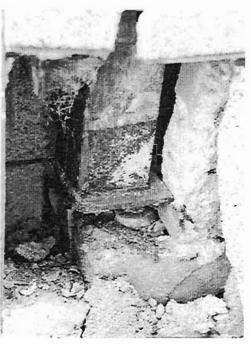
Plate 4.82: Disintegrated plinth of corner column
