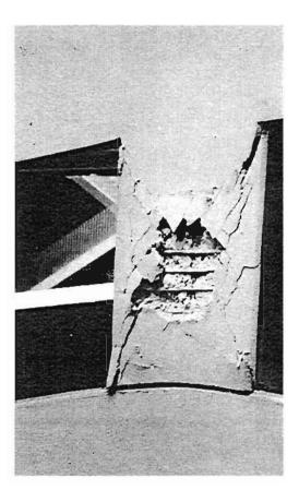
Plate 4.125: Damage to confined concrete at end
