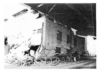
Plate 4.158: Substation collapsed against viaduct damaging viaduct
