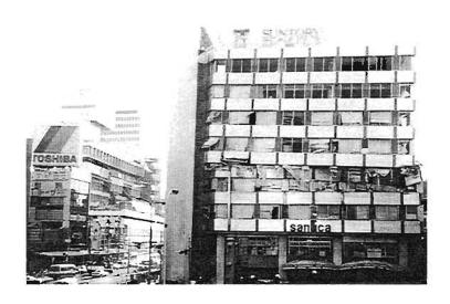
Plate 4.14: 4th and 5th Storey collapse in 9 storey building
