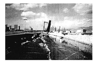
Plate 8.9: Grabens and depressions at the apron slabs behind quay walls
