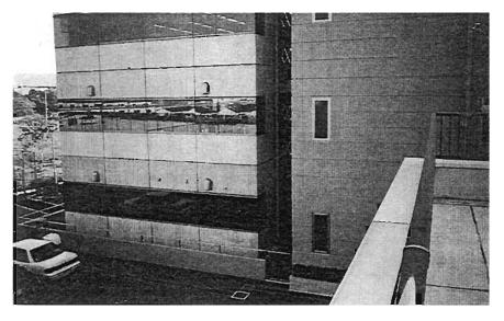
Plate 4.146: The MTRC (base-isolated RC building frame building on the righ and expansion joints in be
