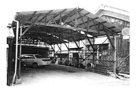
Plate 4.114: Undamaged bamboo portal garage
