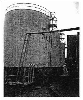
Plate 7.24 Lightly restrained pipes deformed not fractured
