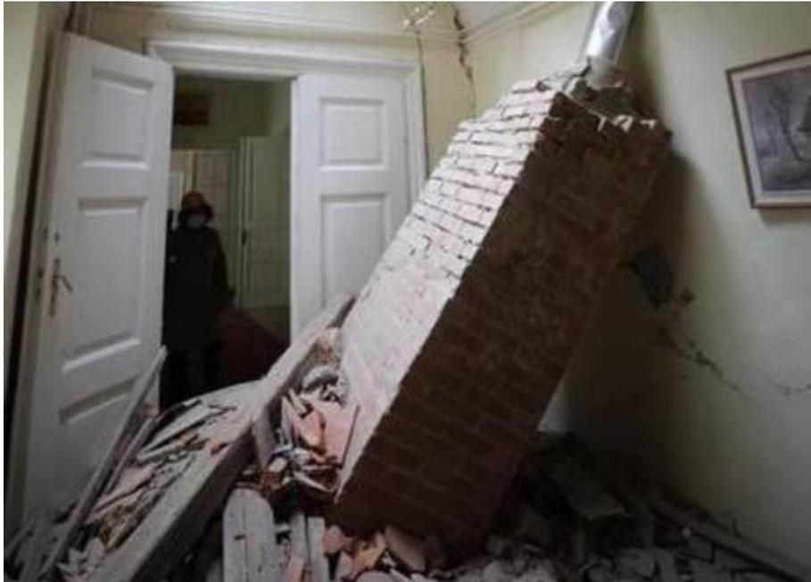
Figure 5-1 Damage of chimney falling indoor Source: City of Zagreb
